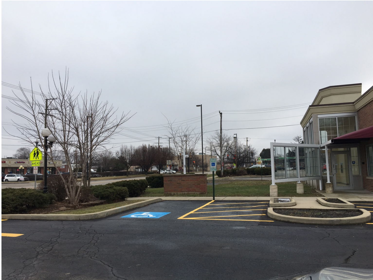
Existing conditions of subject property (looking east)
