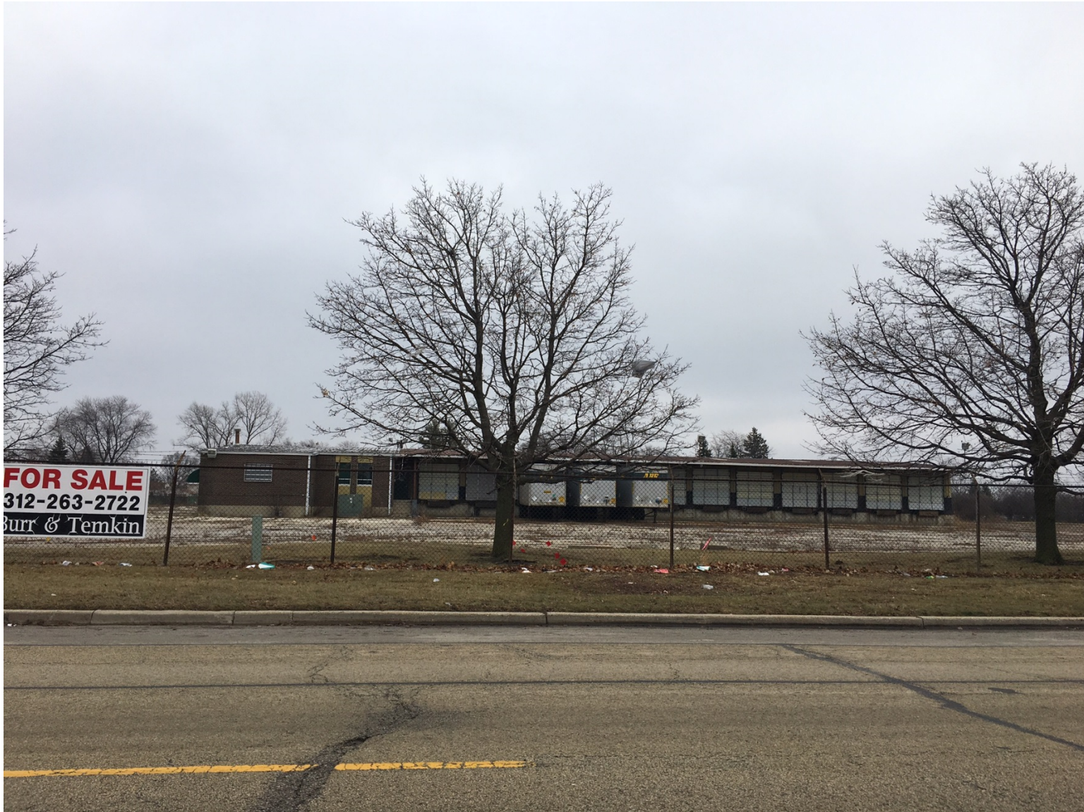
Existing conditions of subject property (looking east)
