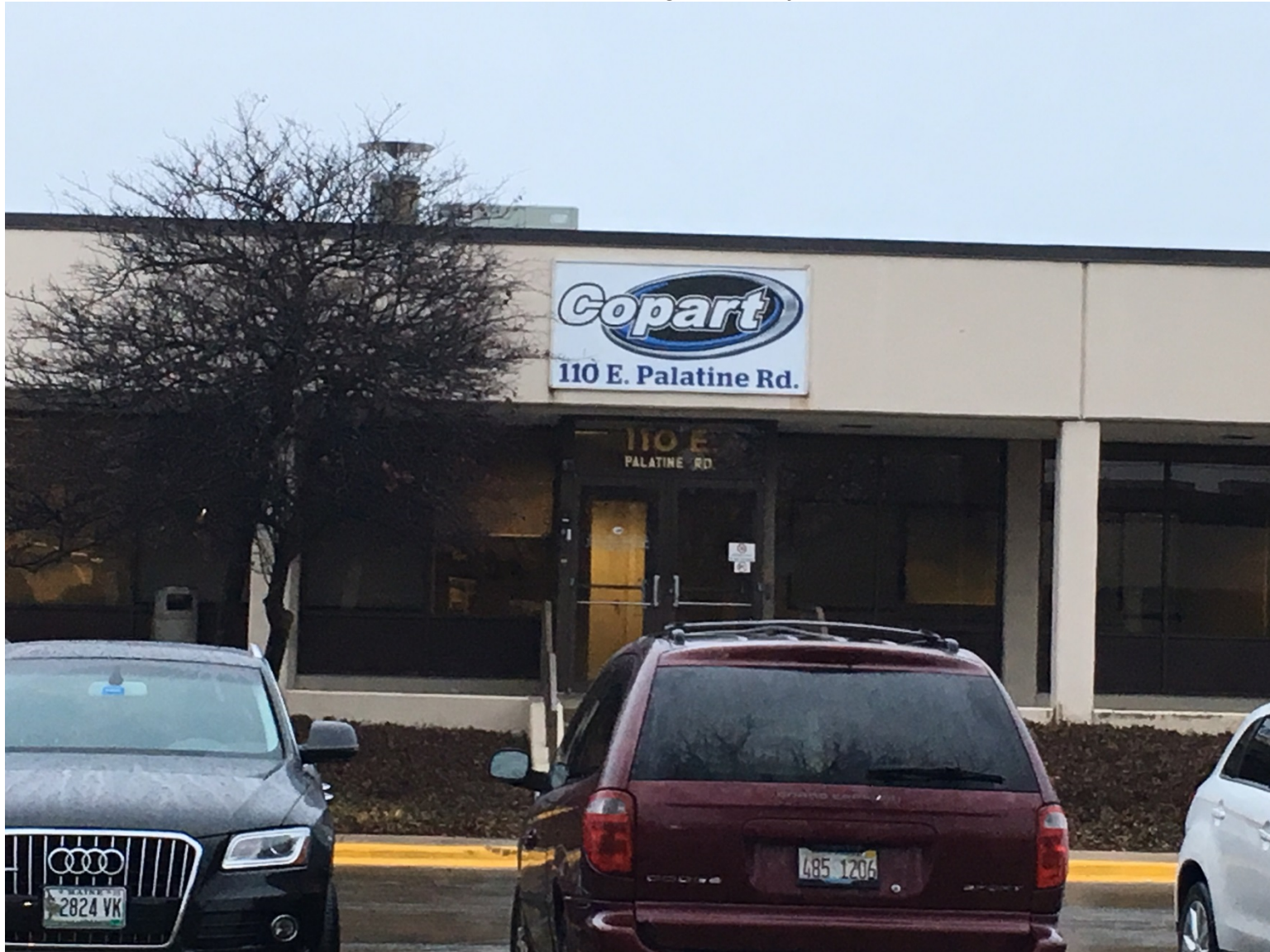
Existing conditions of wall sign – looking north
