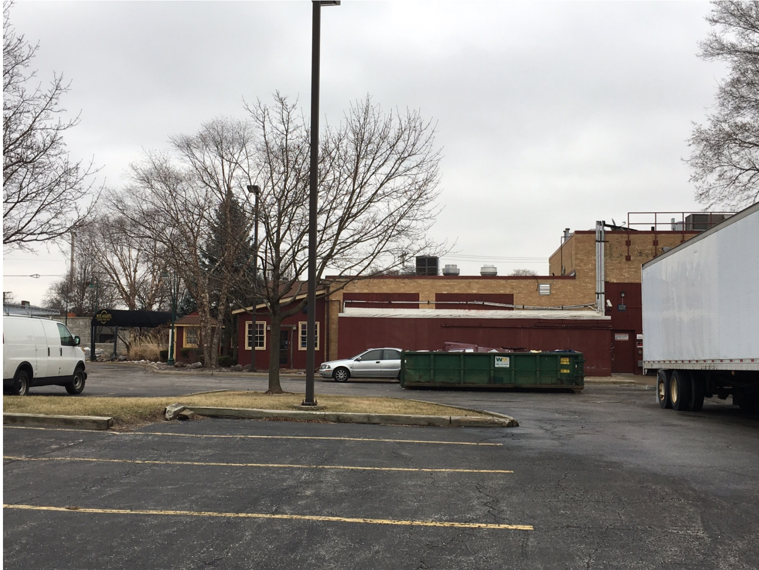
Existing conditions of rear of building (looking east)
