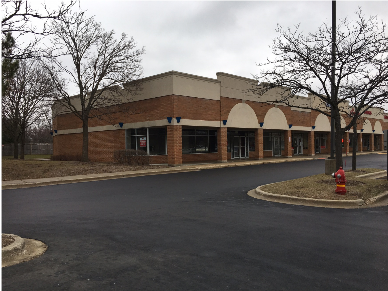
Existing conditions of subject unit (looking northeast)
