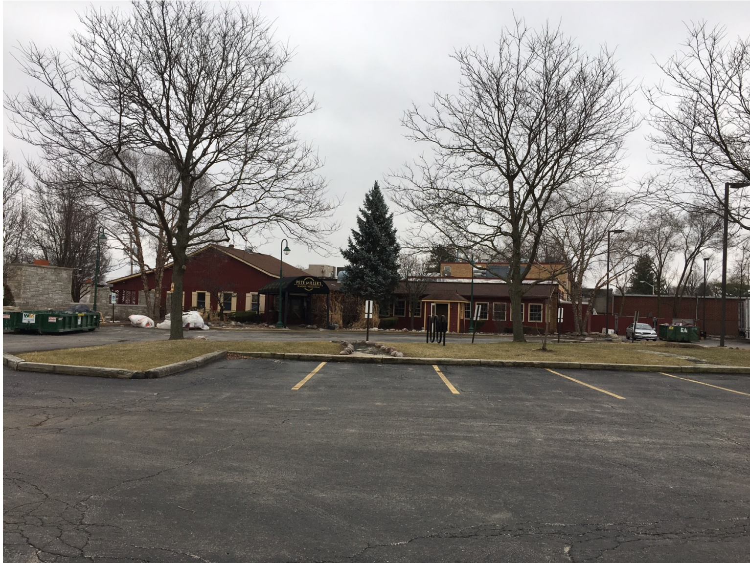
Existing conditions of building (looking south)
