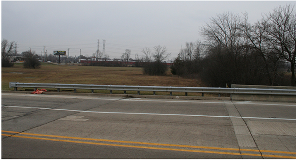
Looking West from Northgate Parkway bridge
