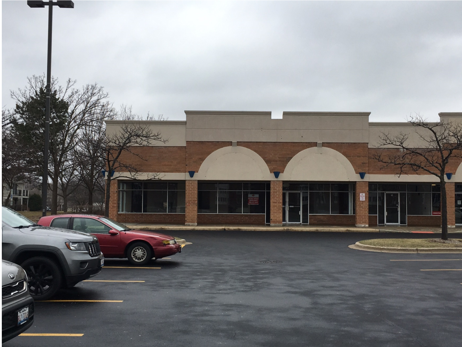
Existing conditions of subject unit (looking north)
