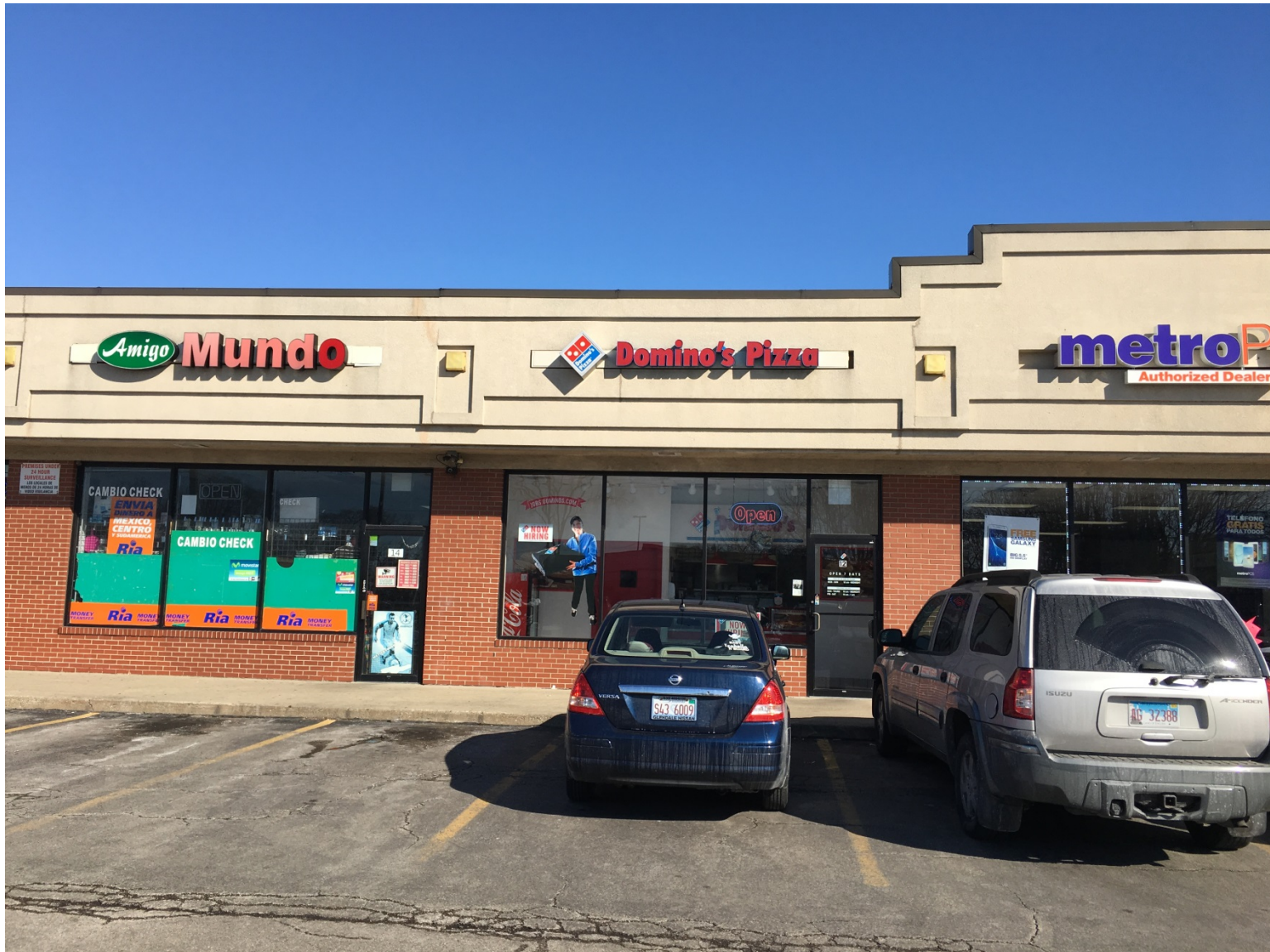
Existing conditions of store front – looking north
