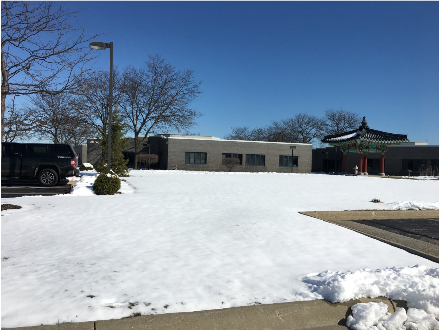
Existing conditions of subject property (looking northeast)
