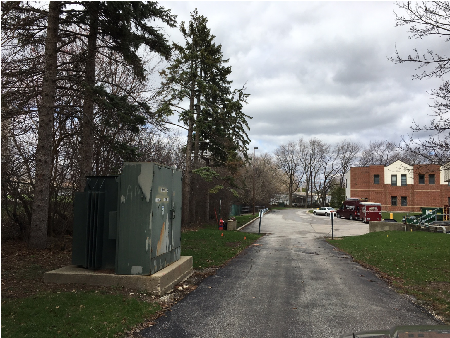
Proposed path area, adjacent to northern end of fire lane – looking north
