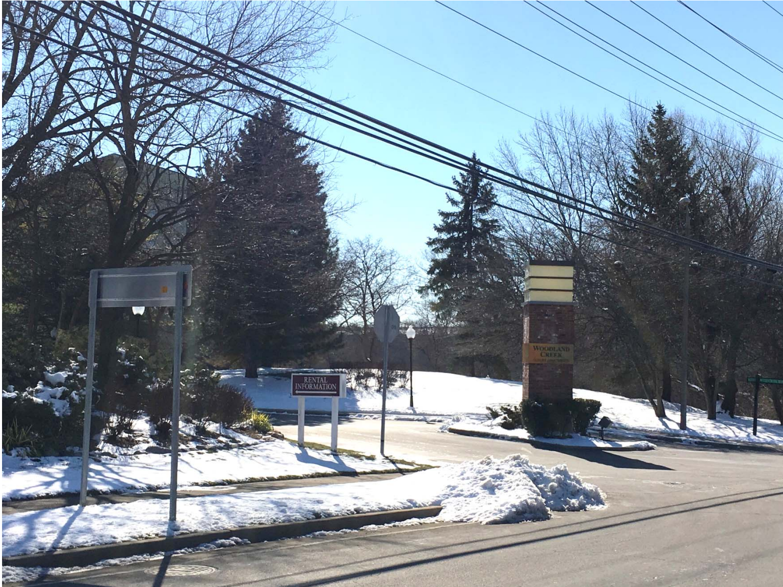
Existing conditions of single-pillar subdivision sign (looking southeast)
