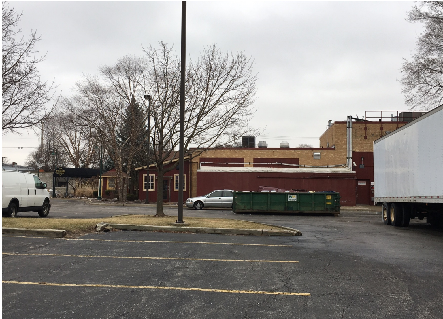
Existing conditions of rear of building (looking east)
