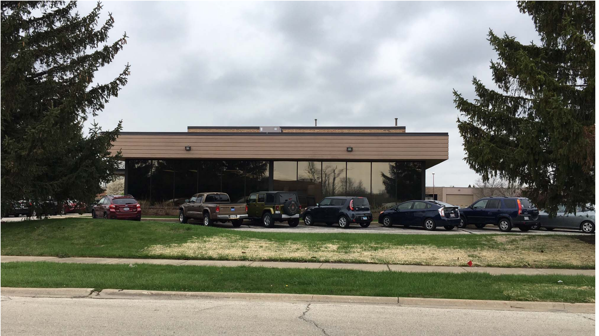
Existing conditions along Chaddick Drive – looking west
