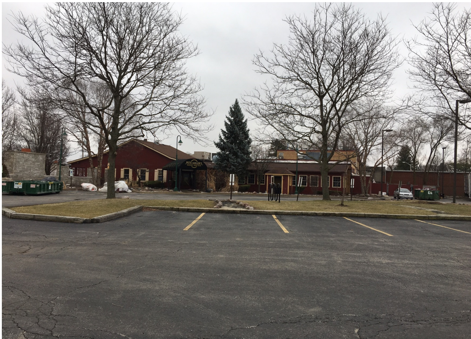
Existing conditions of building (looking south)
