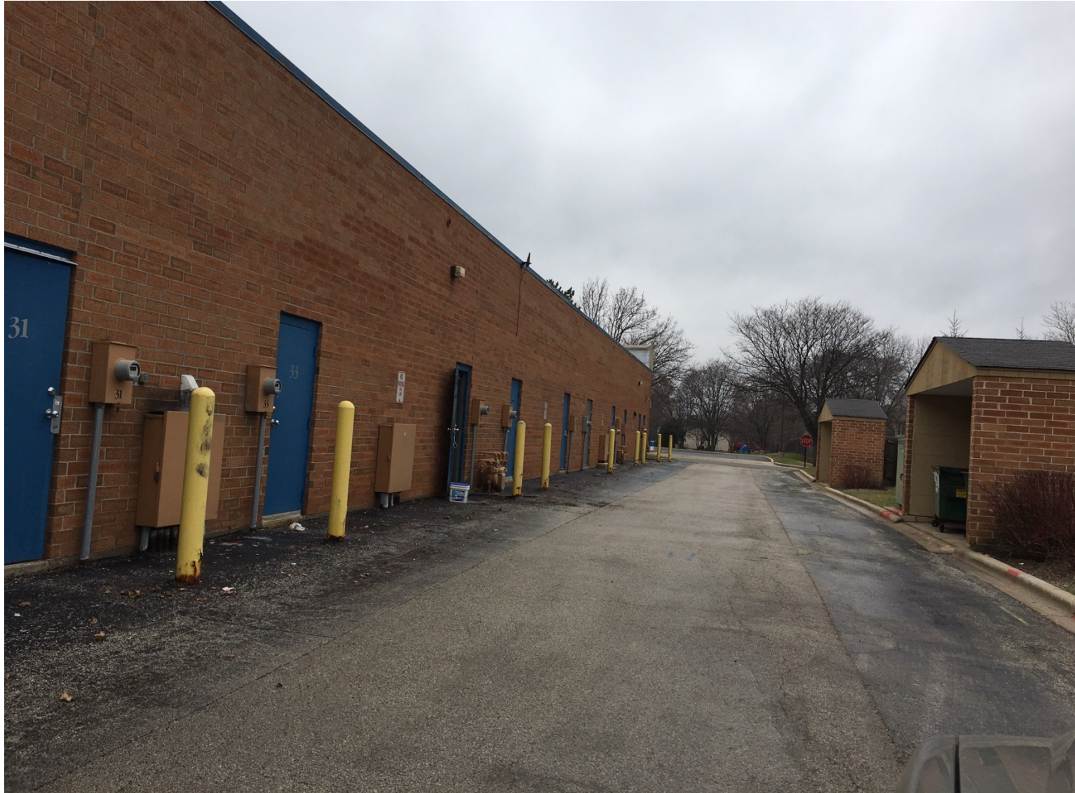
Existing conditions of rear access drive and trash enclosures (looking west)
