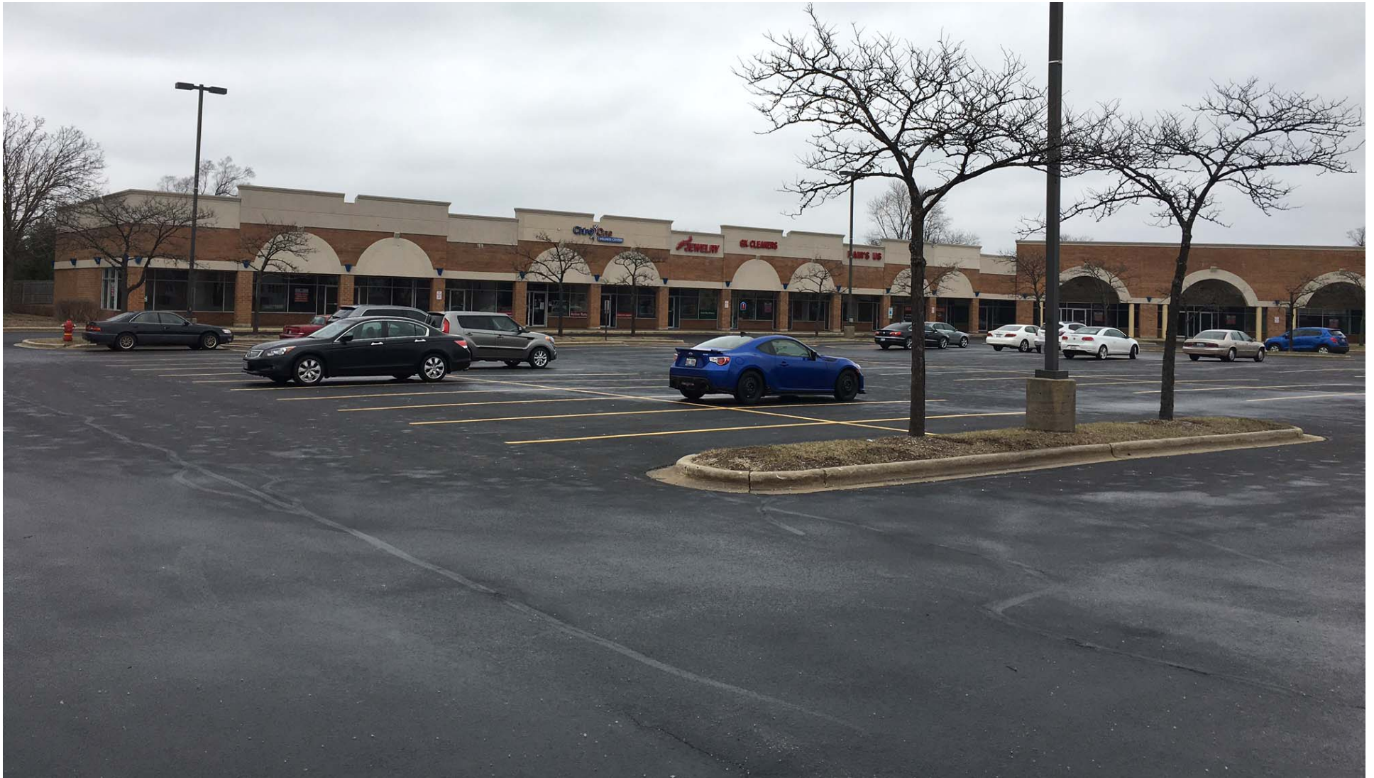
Existing conditions of subject property (looking northeast)
