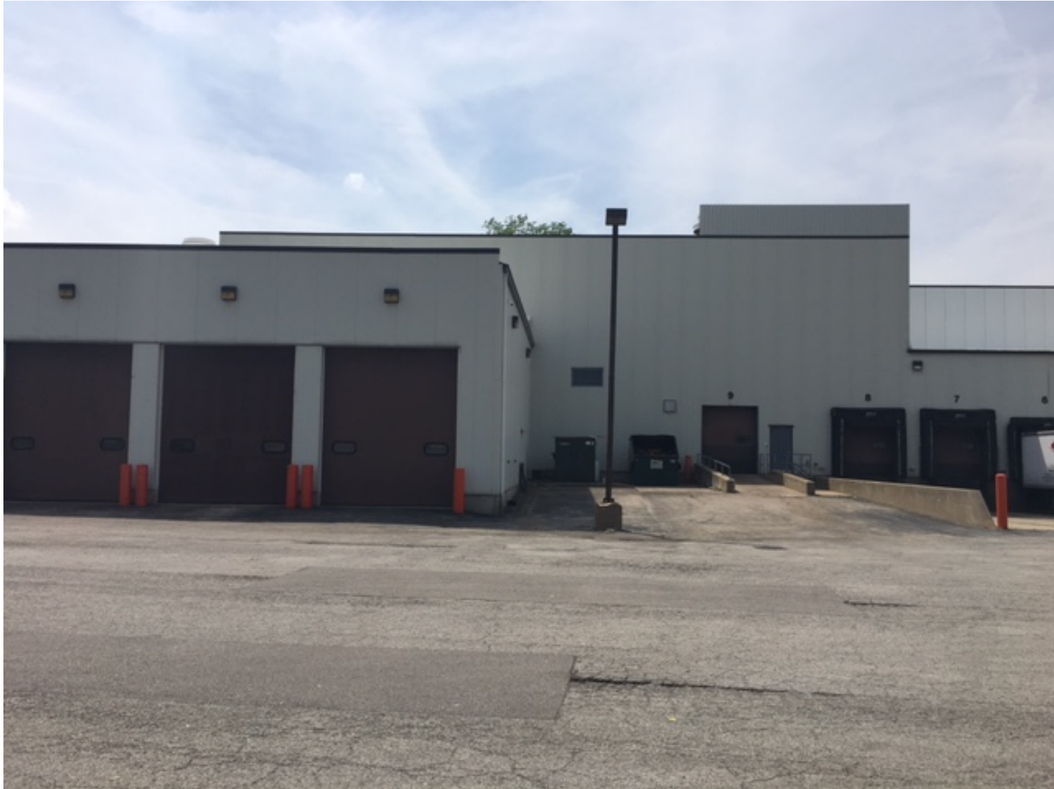
Existing conditions of east façade – looking west
