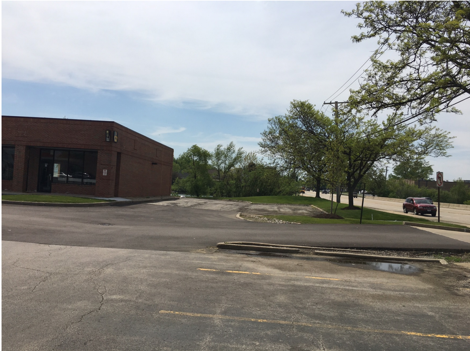
Existing conditions of north edge of property (along Hintz Road) – looking west
