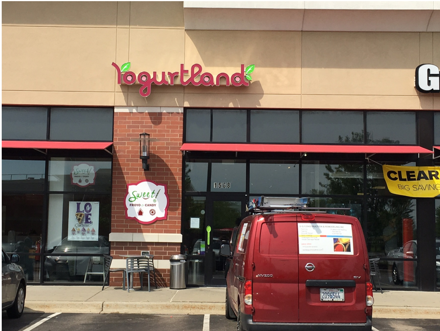
Existing conditions of front façade – looking north
