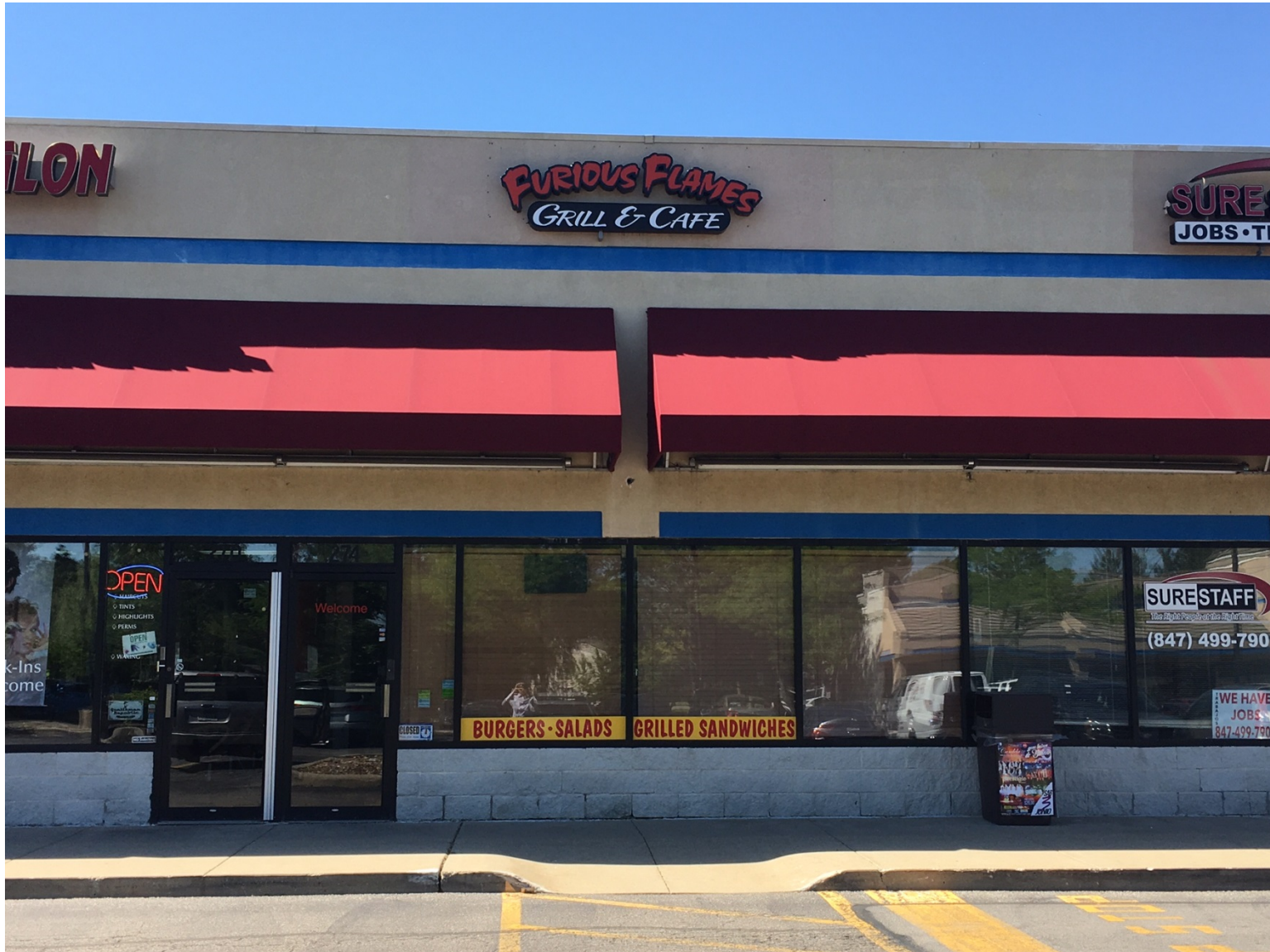
Existing conditions of front façade – looking south
