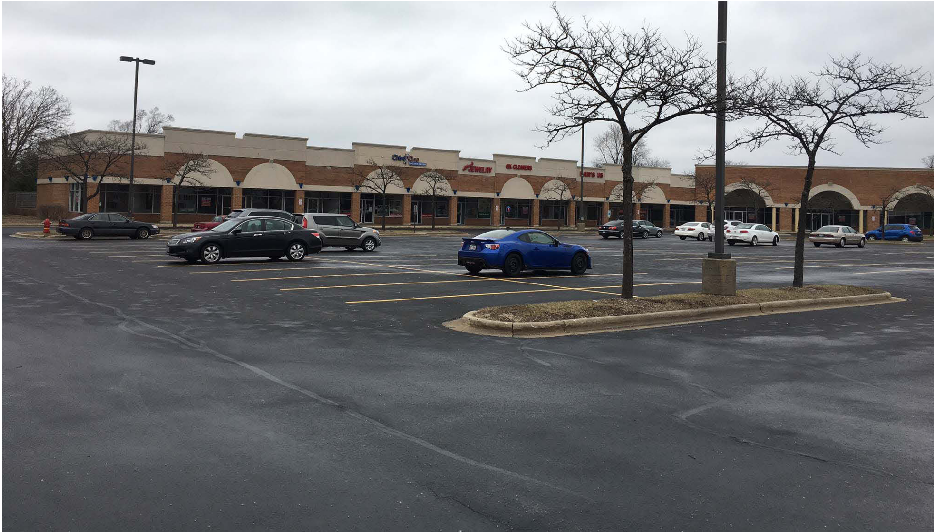
Existing conditions of subject property (looking northeast)
