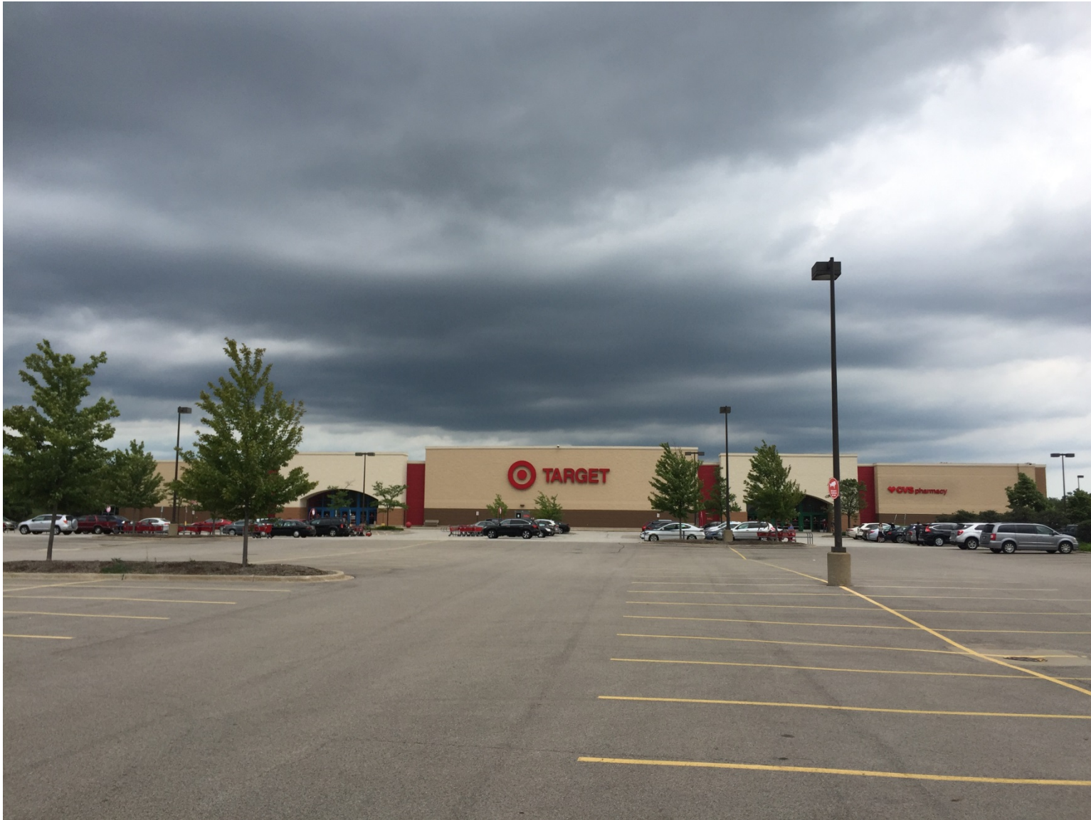
Existing conditions of the store (looking east)
