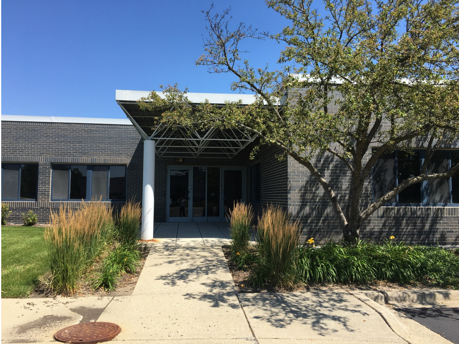
Existing conditions of West Entry (looking north)
