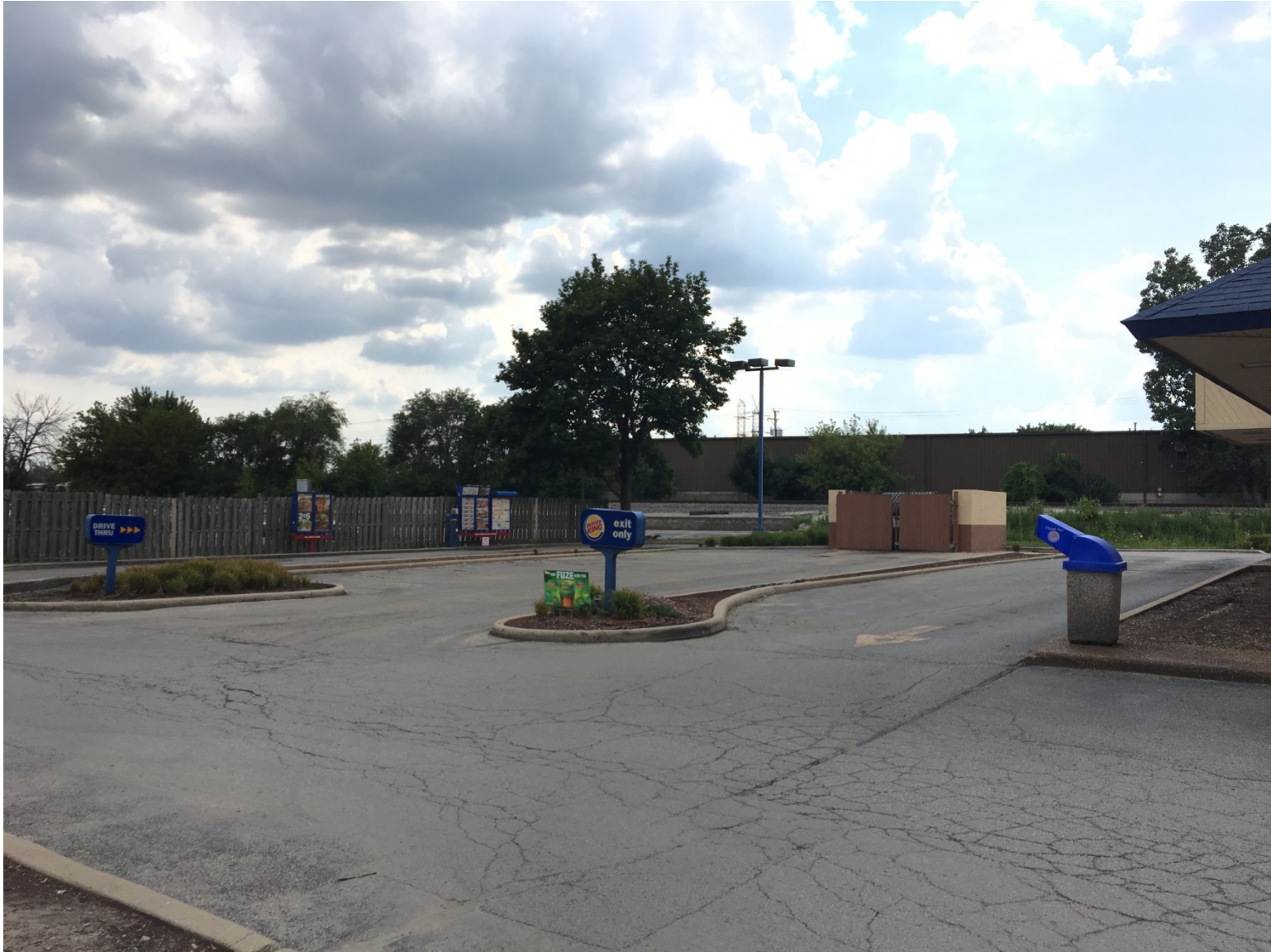
Existing conditions drive-thru configuration (looking southwest)
