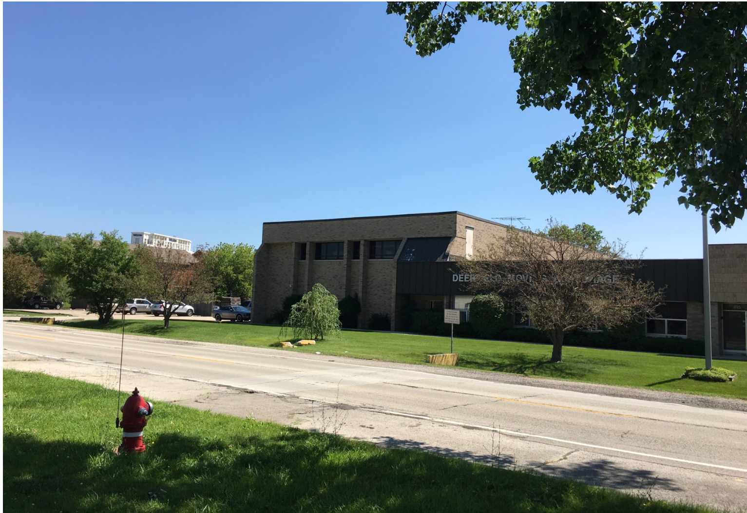
Existing conditions of the property (looking east)
