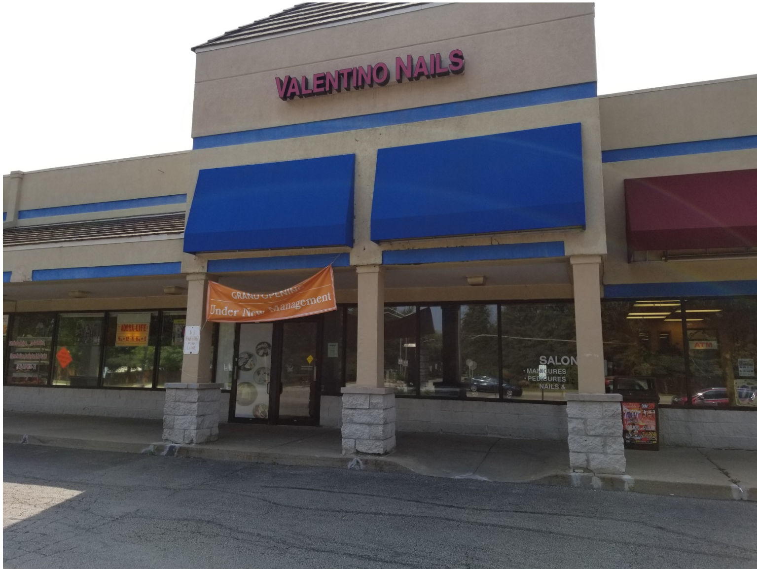
Existing conditions of front façade – looking south
