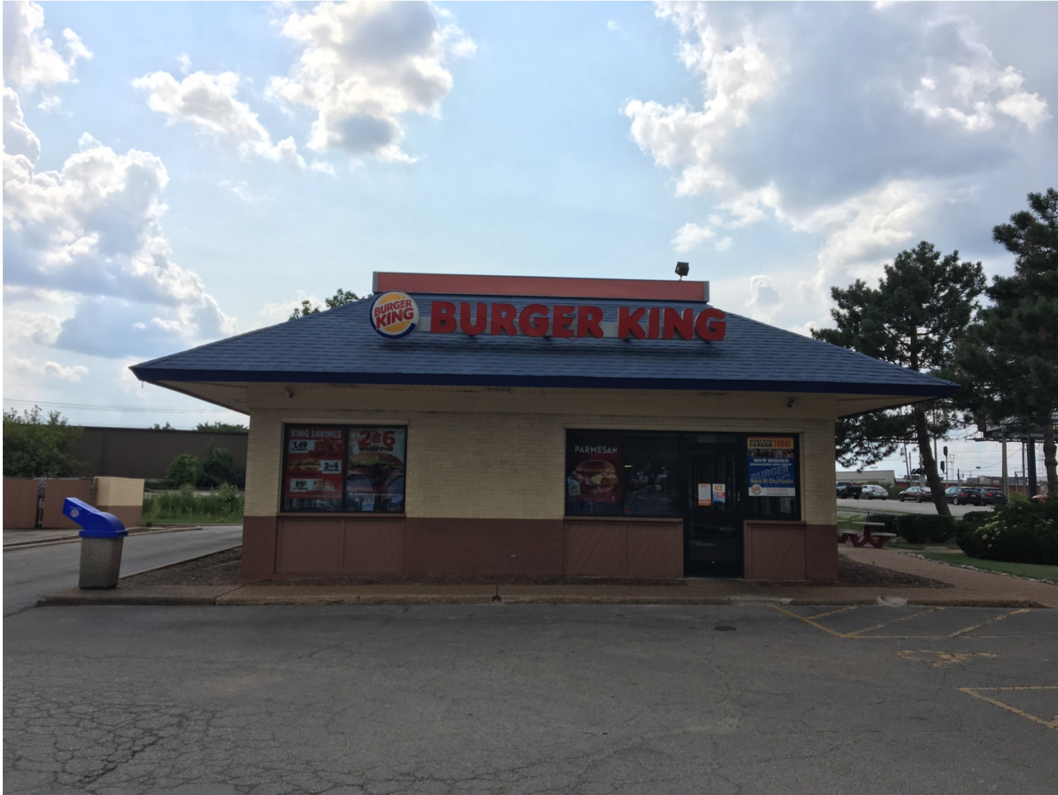
Existing conditions of front (east) building façade (looking west)
