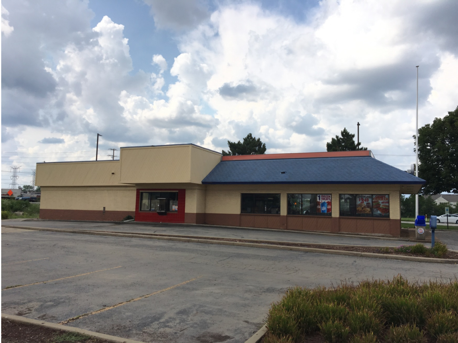
Existing conditions of side (south) building façade (looking north)
