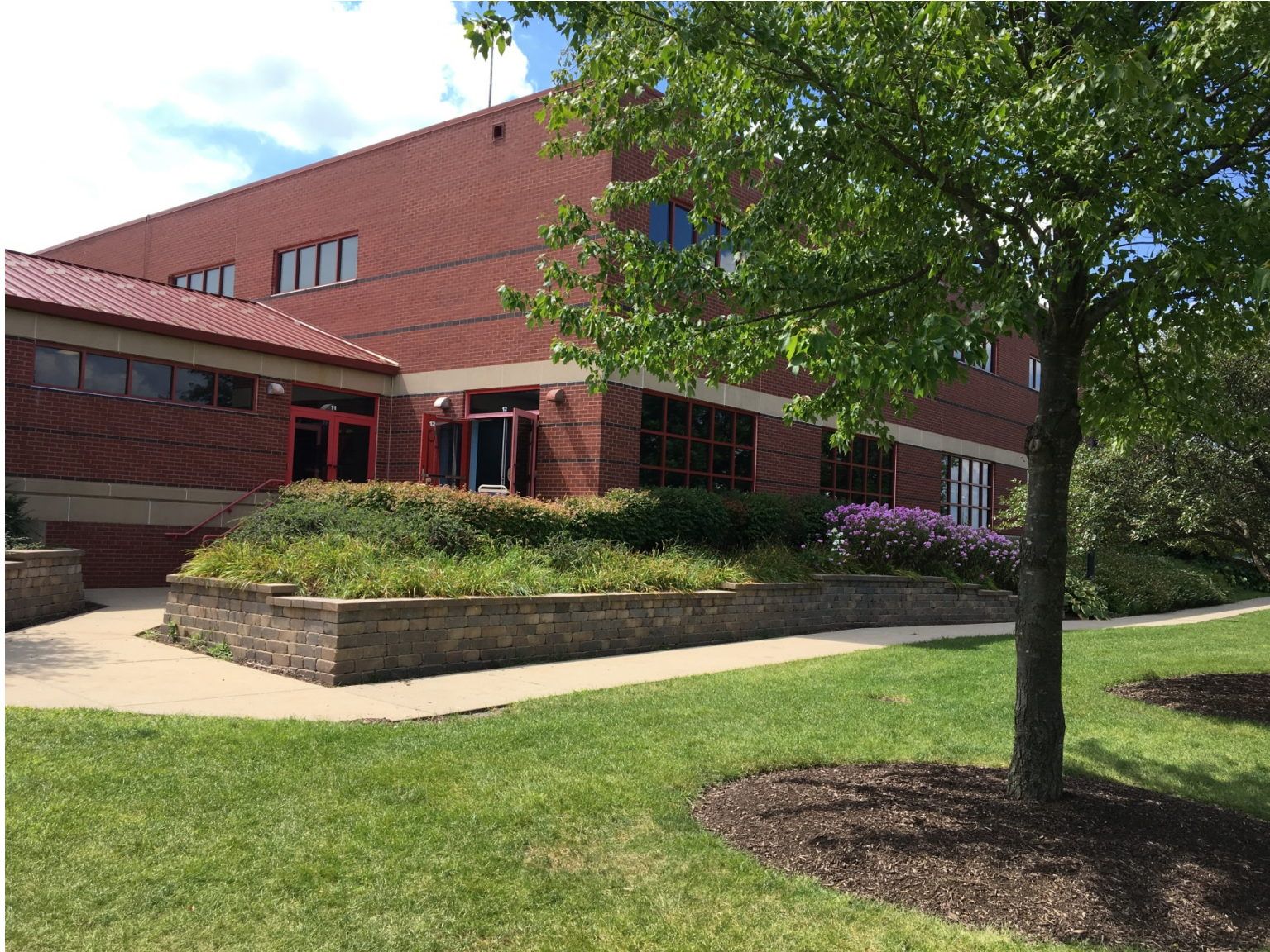
Existing conditions of southeast corner of building (looking west)
