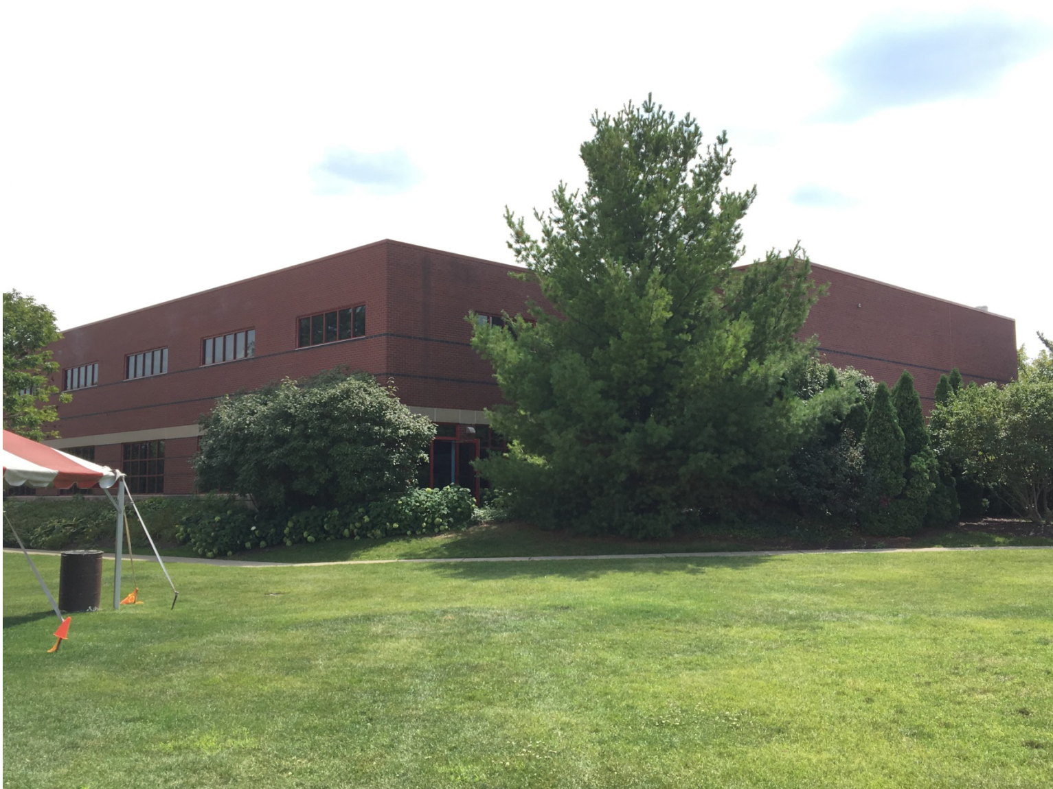
Existing conditions of northeastern facades (looking southwest)
