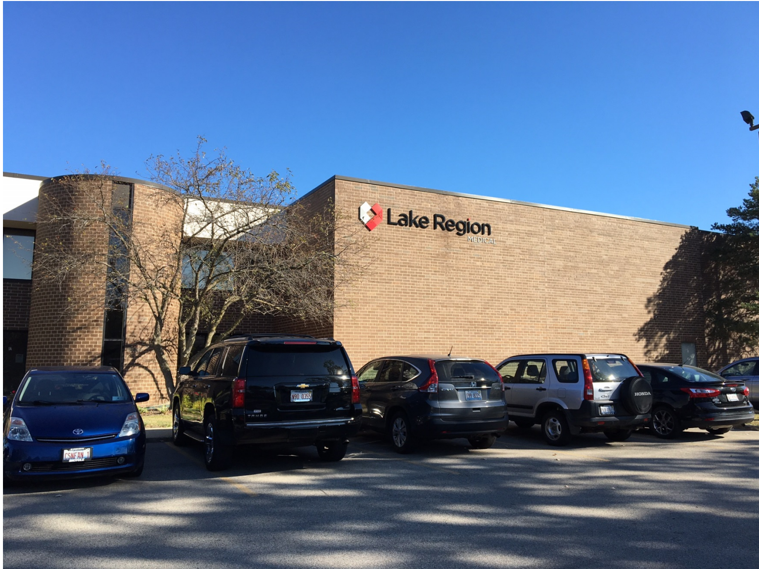
Existing conditions of façade along Hintz Road
