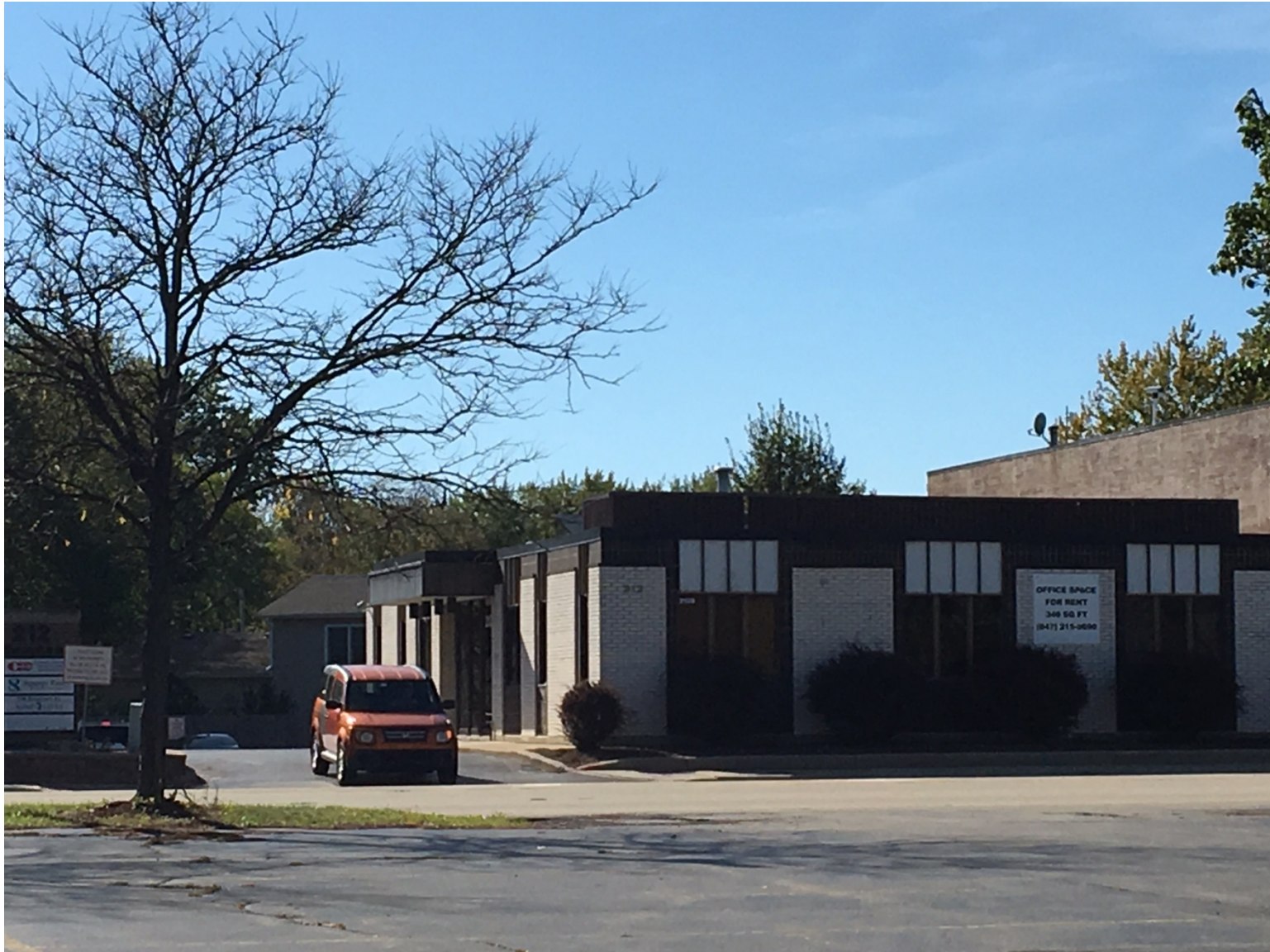
View of 212 S. Milwaukee Avenue building (from the east)
