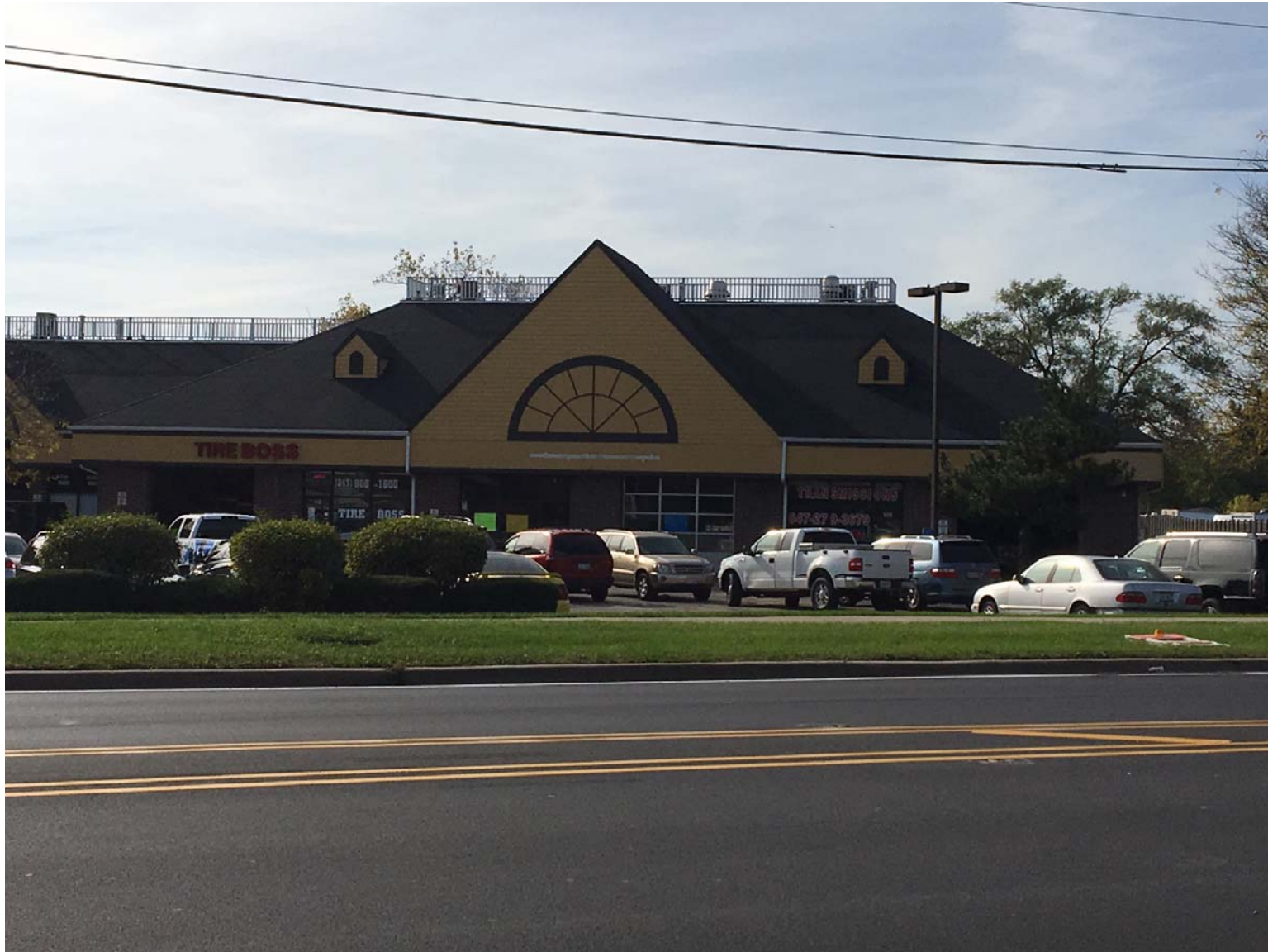
Existing conditions of front façade (looking west)
