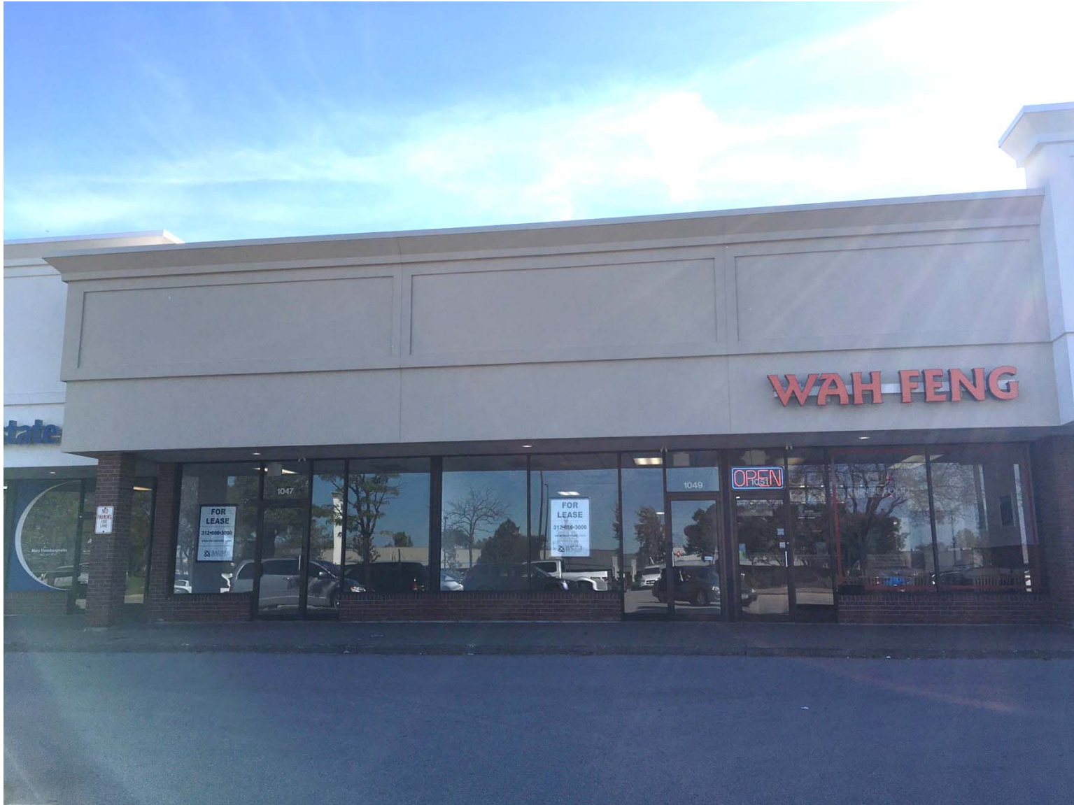
Existing conditions of store front – looking south
