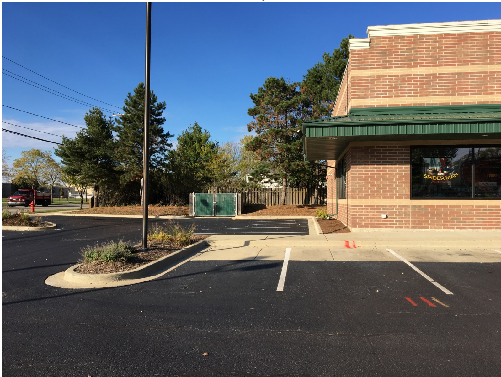
Existing conditions of trash enclosure (looking north)
