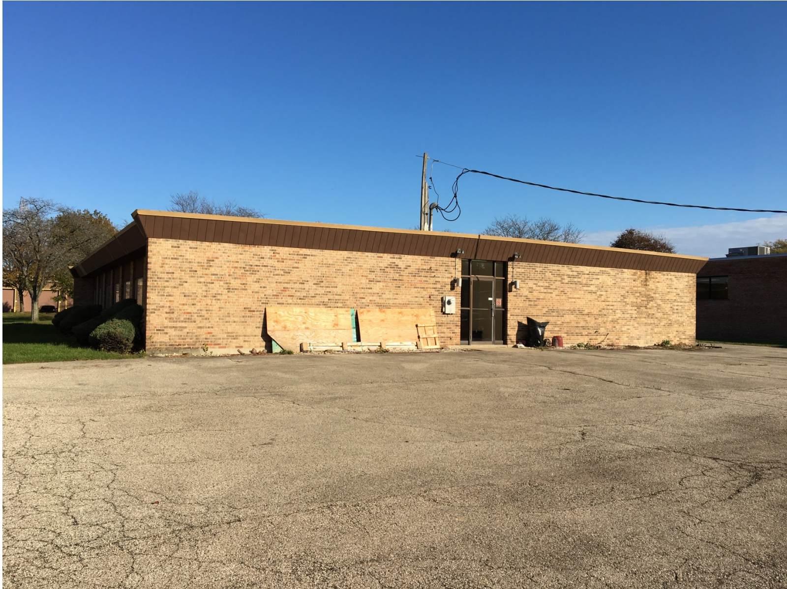
Existing conditions of rear of subject property (looking east)
