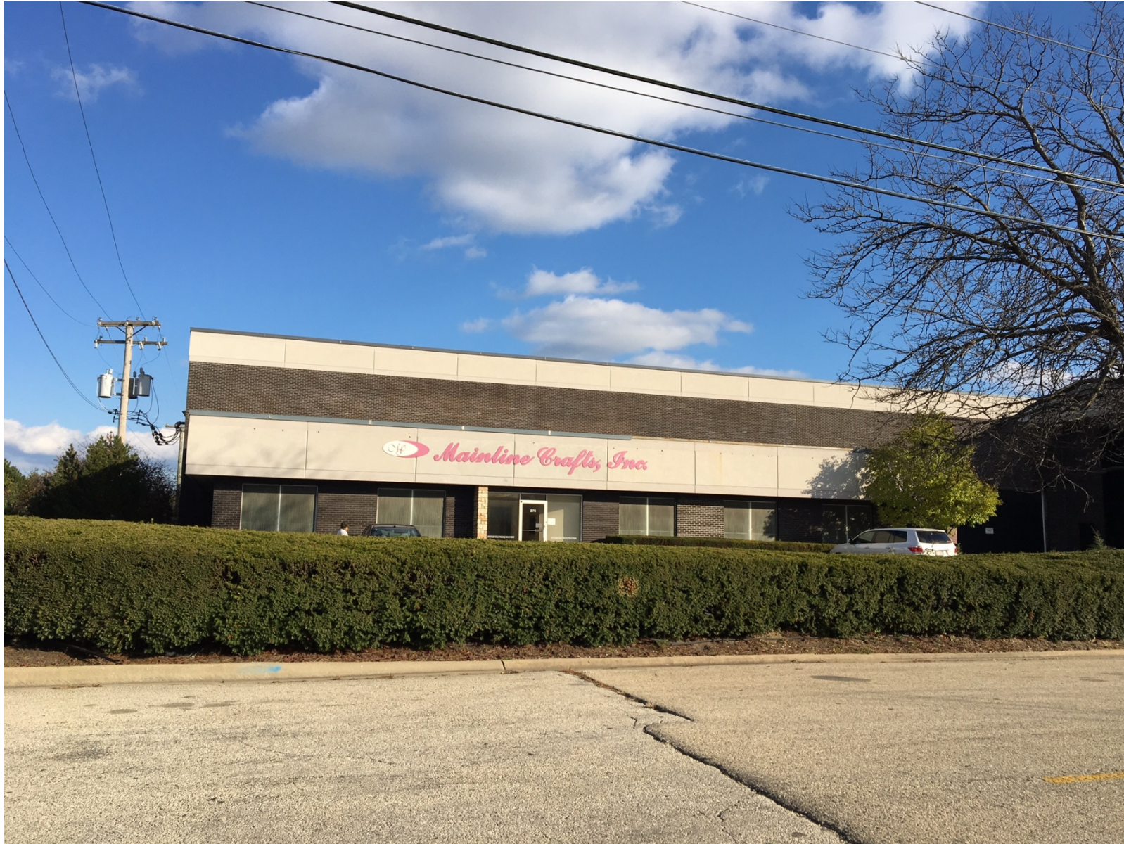
Existing conditions of façade along 12 th Street (looking east)
