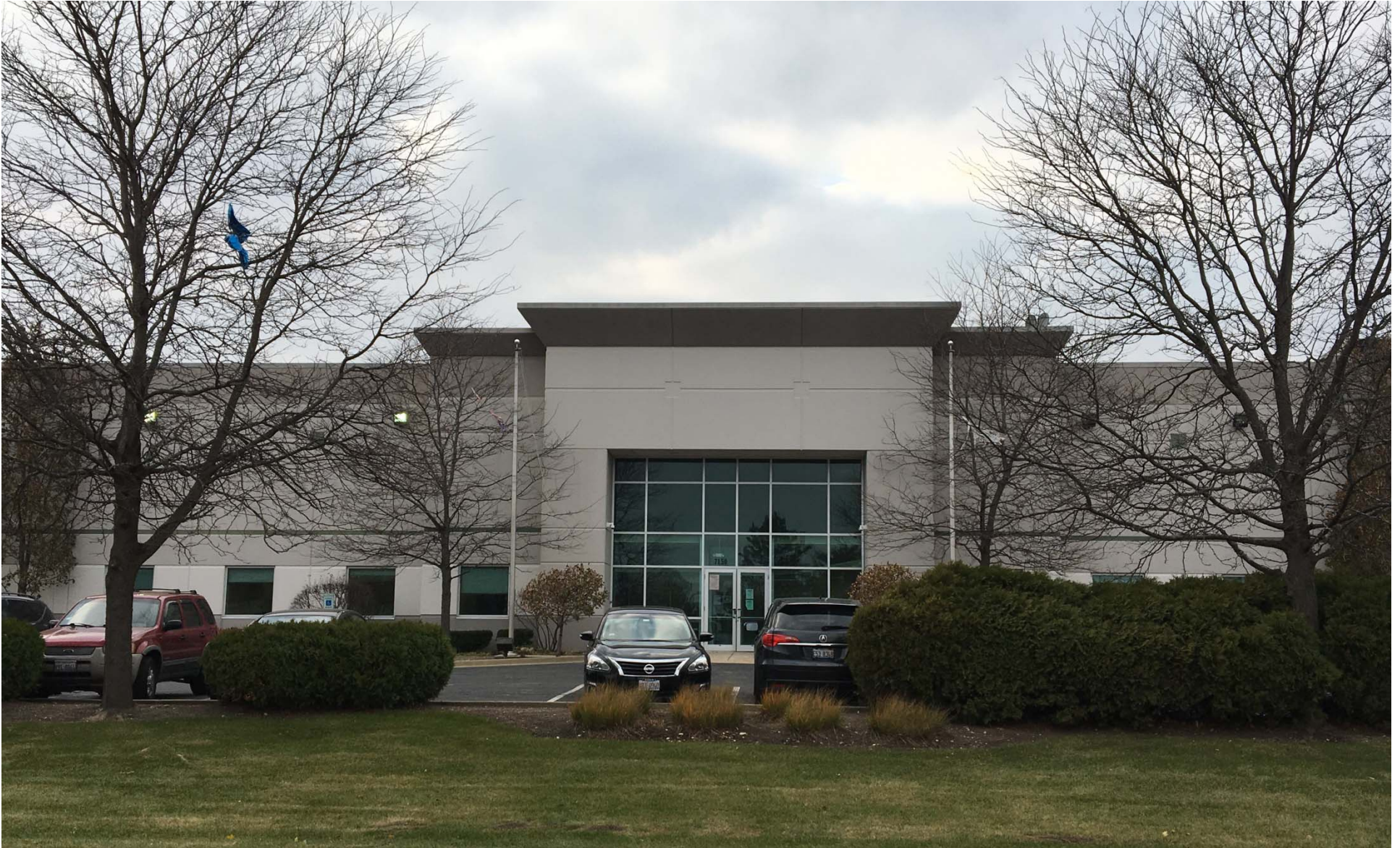
Existing conditions of front façade – looking west
