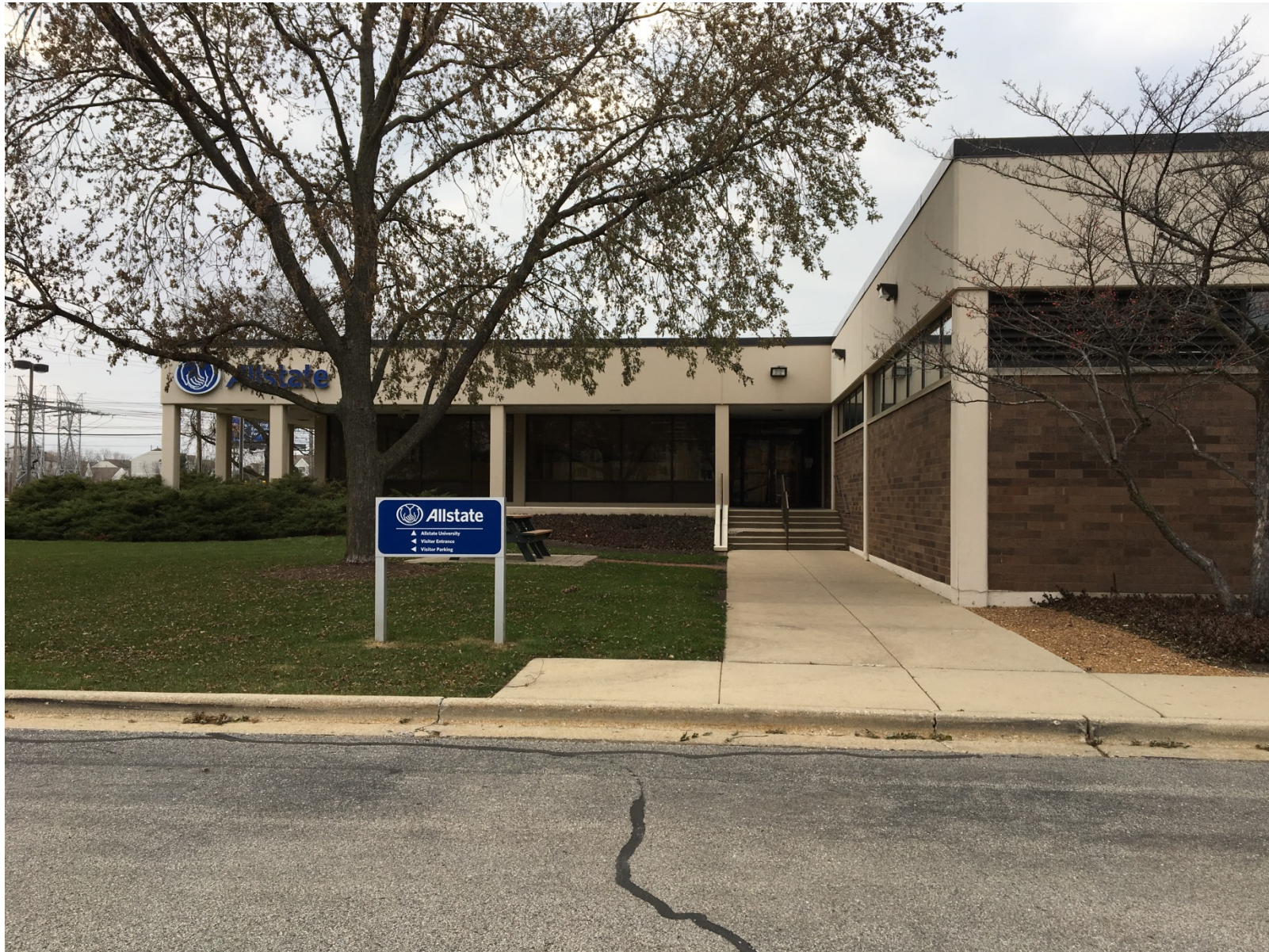
Existing conditions of main entry (looking west)
