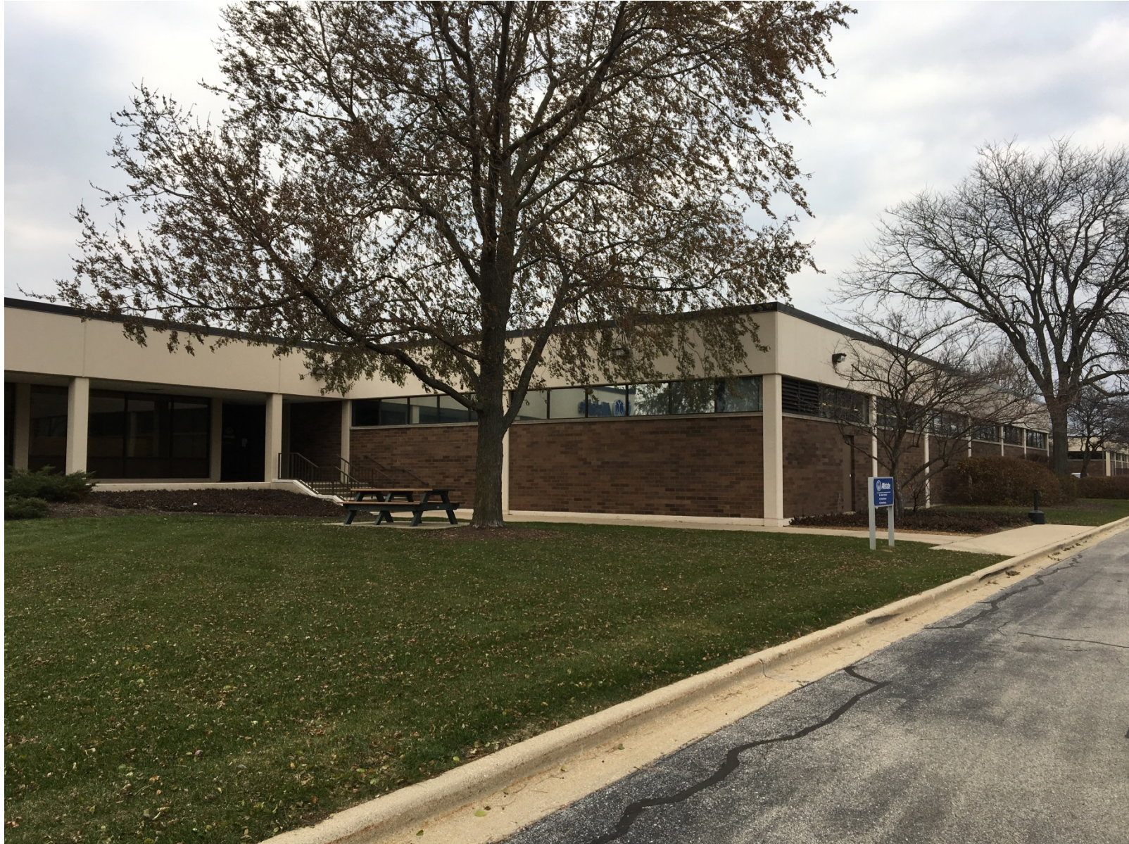
Existing conditions of main entry (looking northwest)
