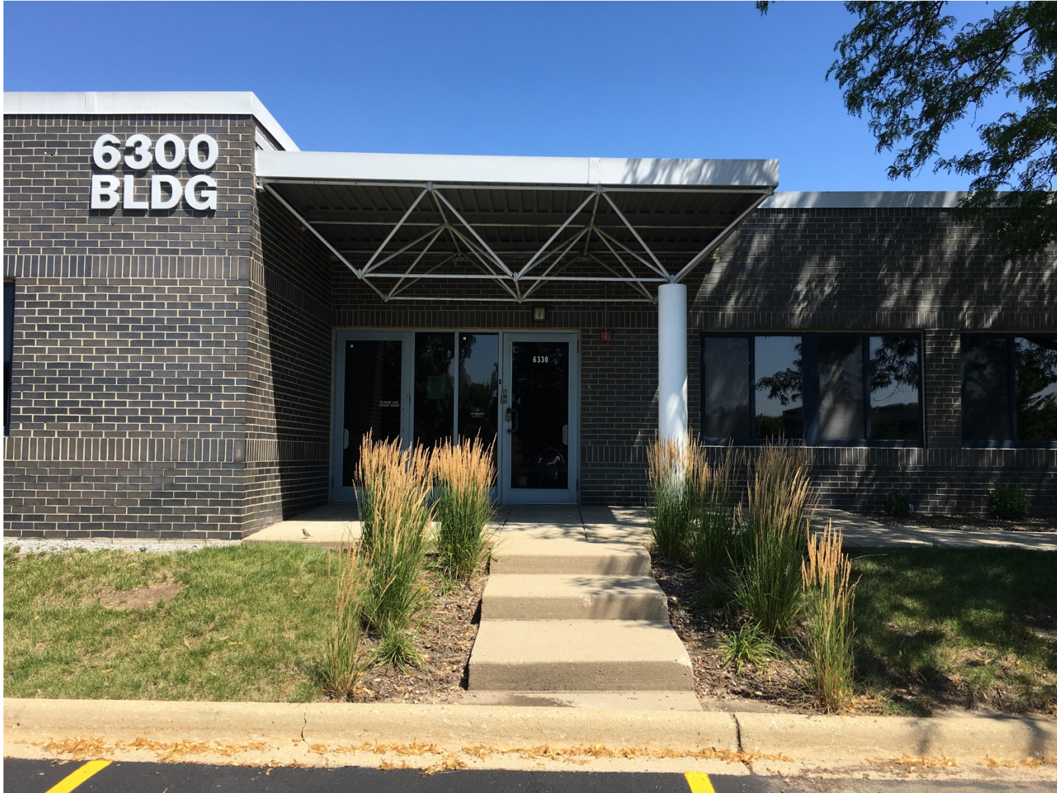
Existing conditions of West Entry (looking north)
