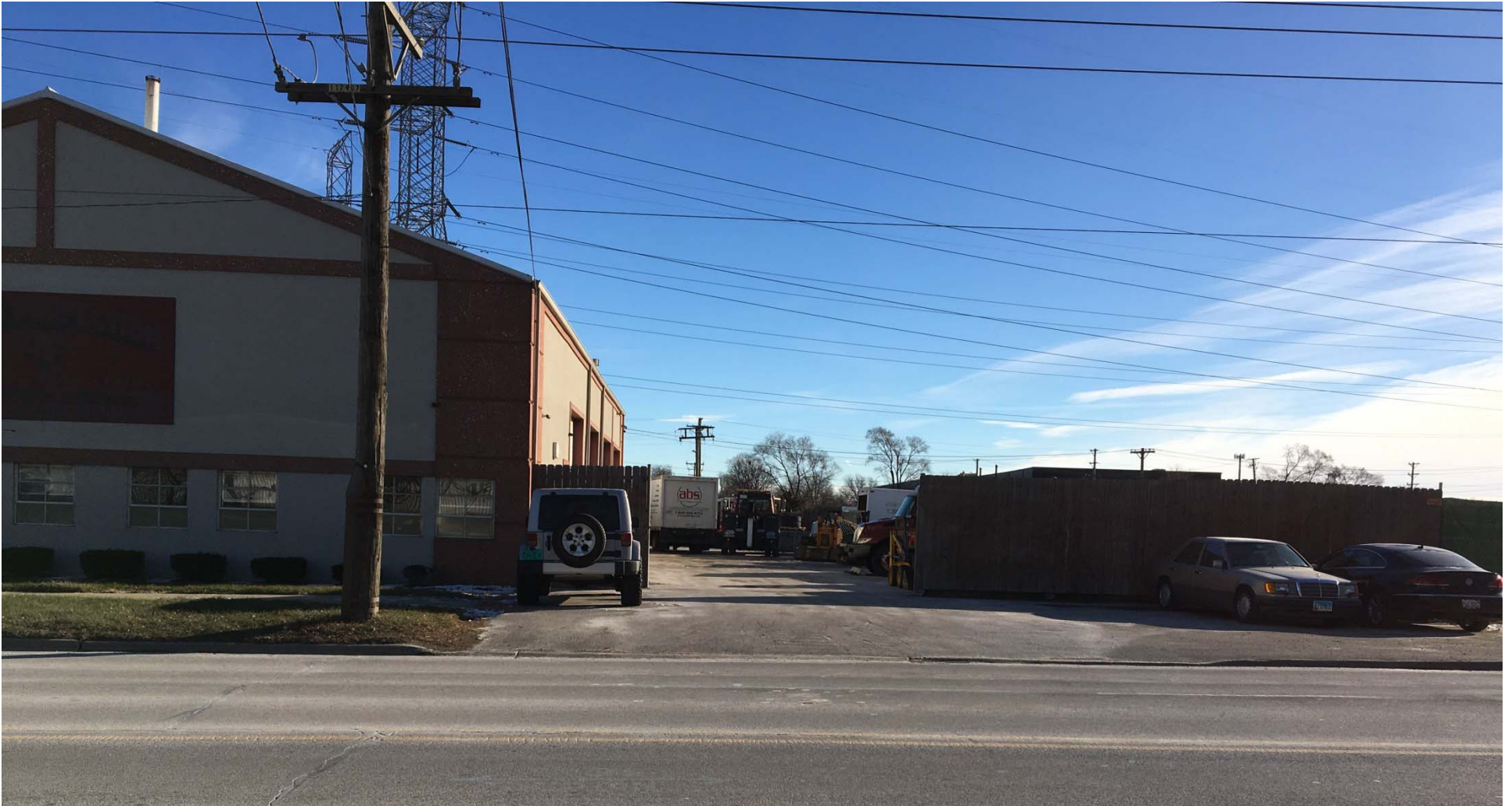
Existing conditions of subject property (looking east)
