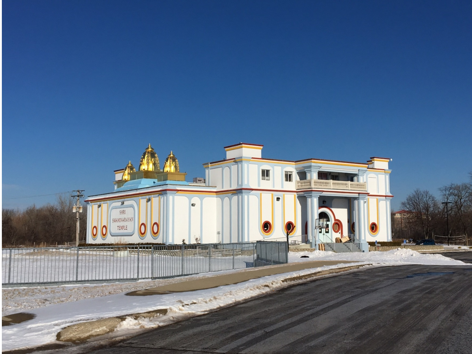
Existing conditions of main entry (looking northeast)
