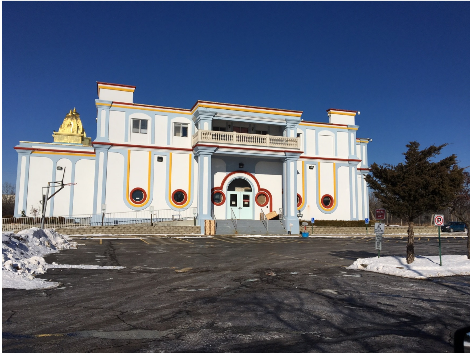
Existing conditions of main entry (looking north)
