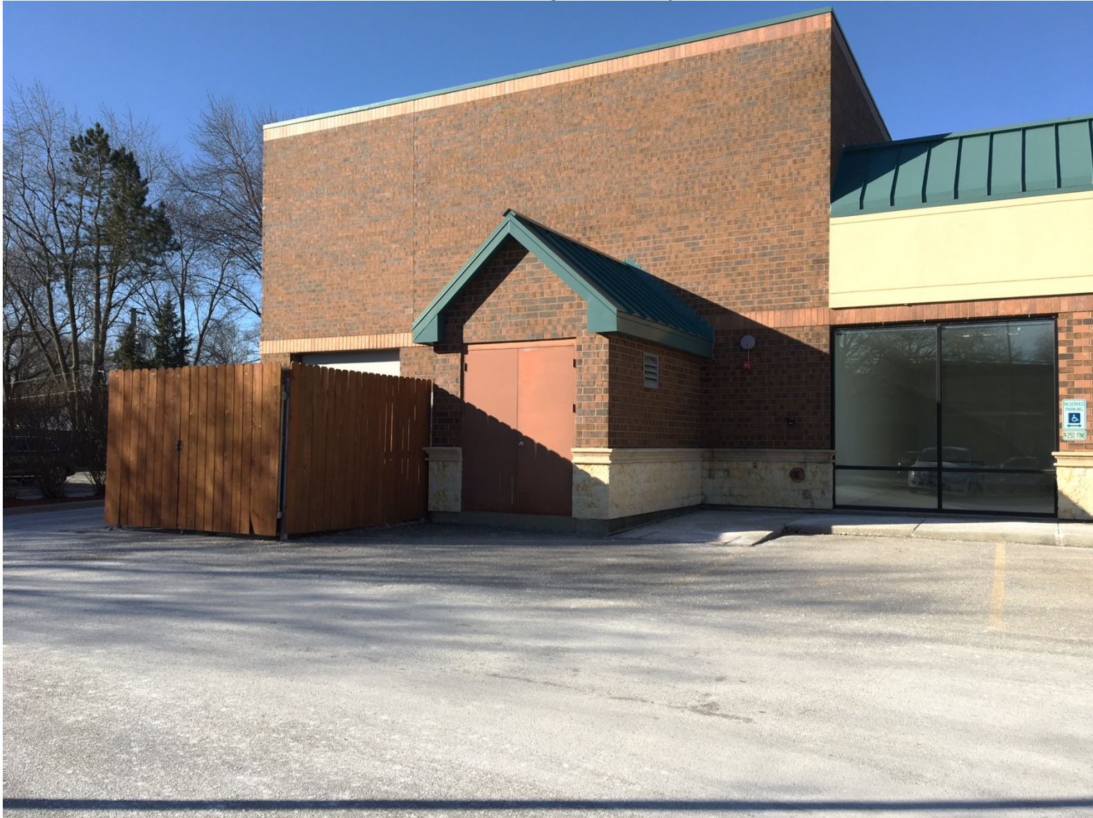
Existing conditions of trash enclosure (looking west)
