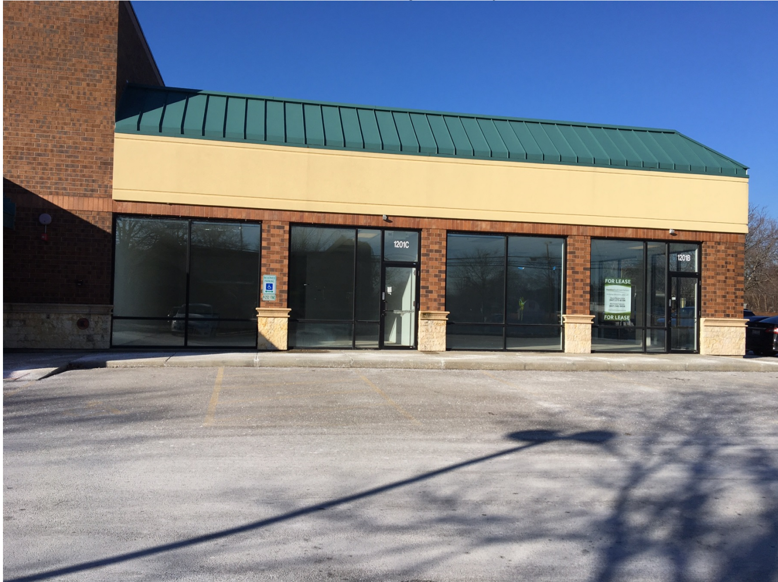
Existing conditions of subject unit (looking west)
