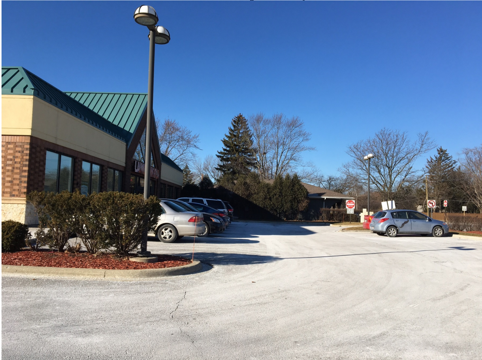
Existing conditions of subject property looking west)
