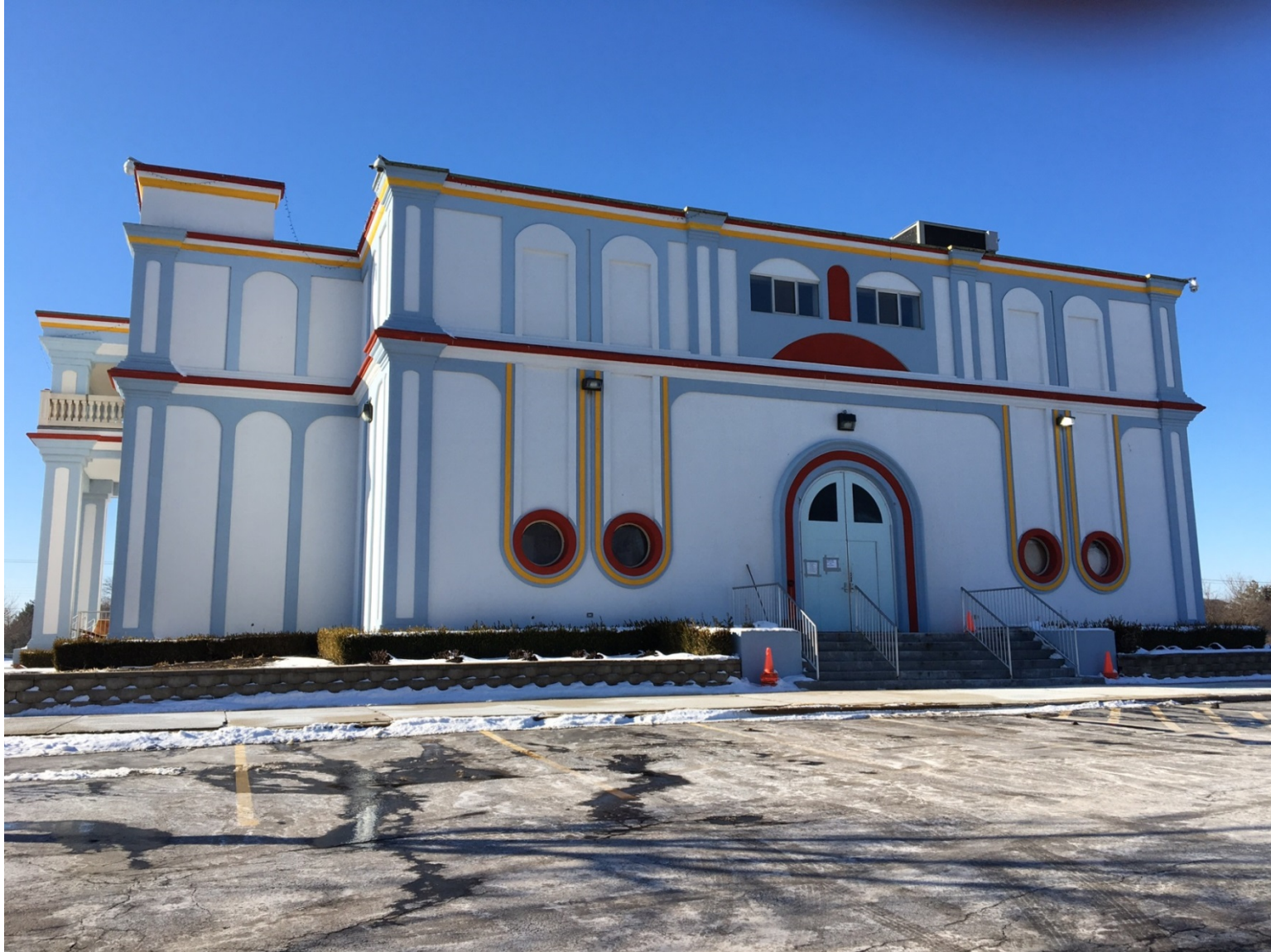
Existing conditions of east façade (looking west)
