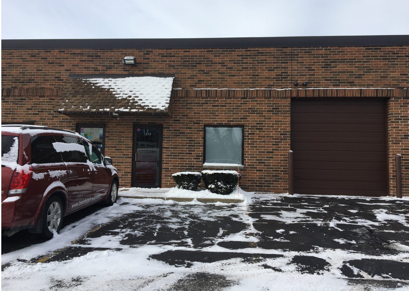
Existing conditions of subject unit (looking west)
