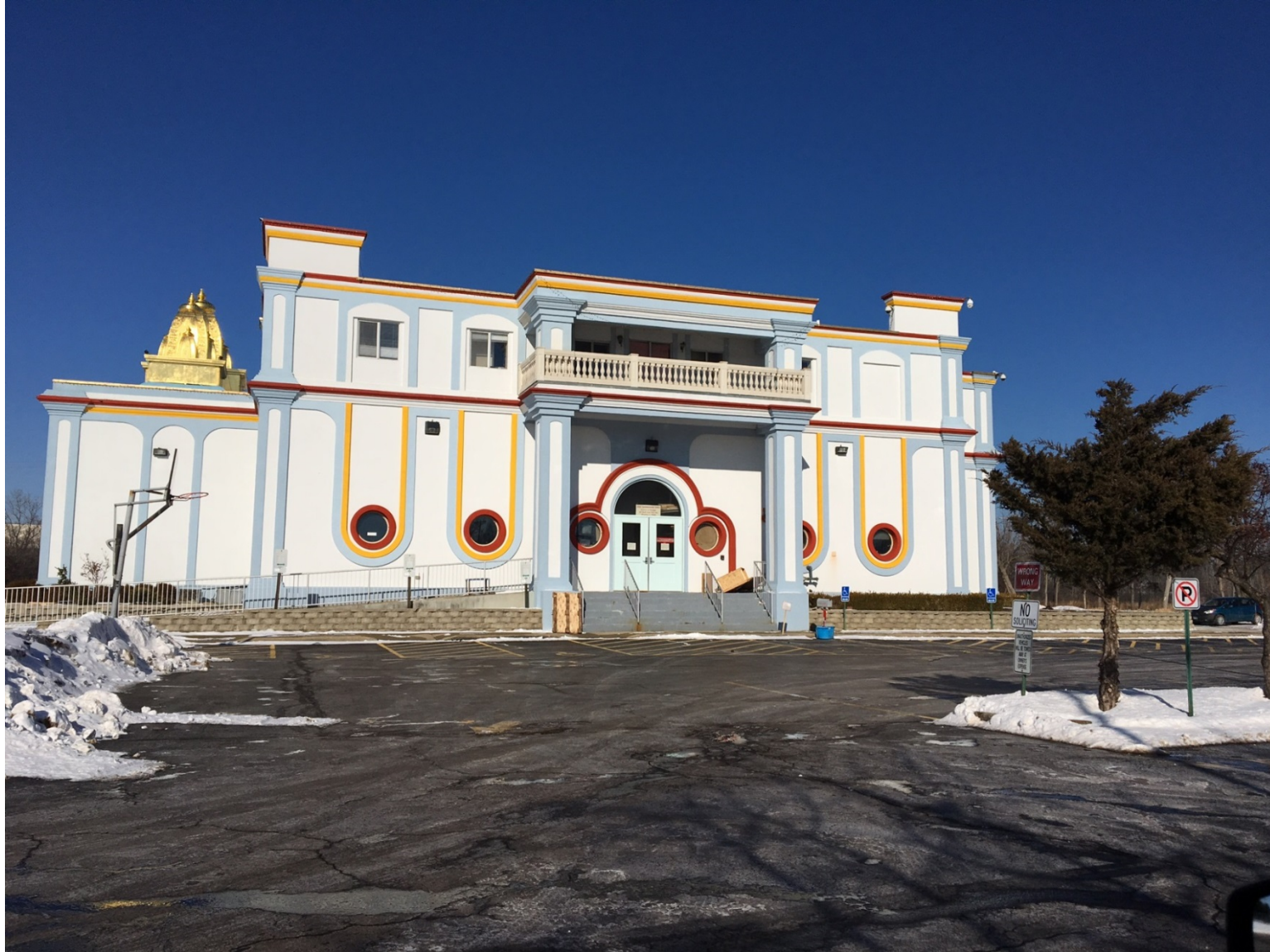
Existing conditions of south façade (looking north)
