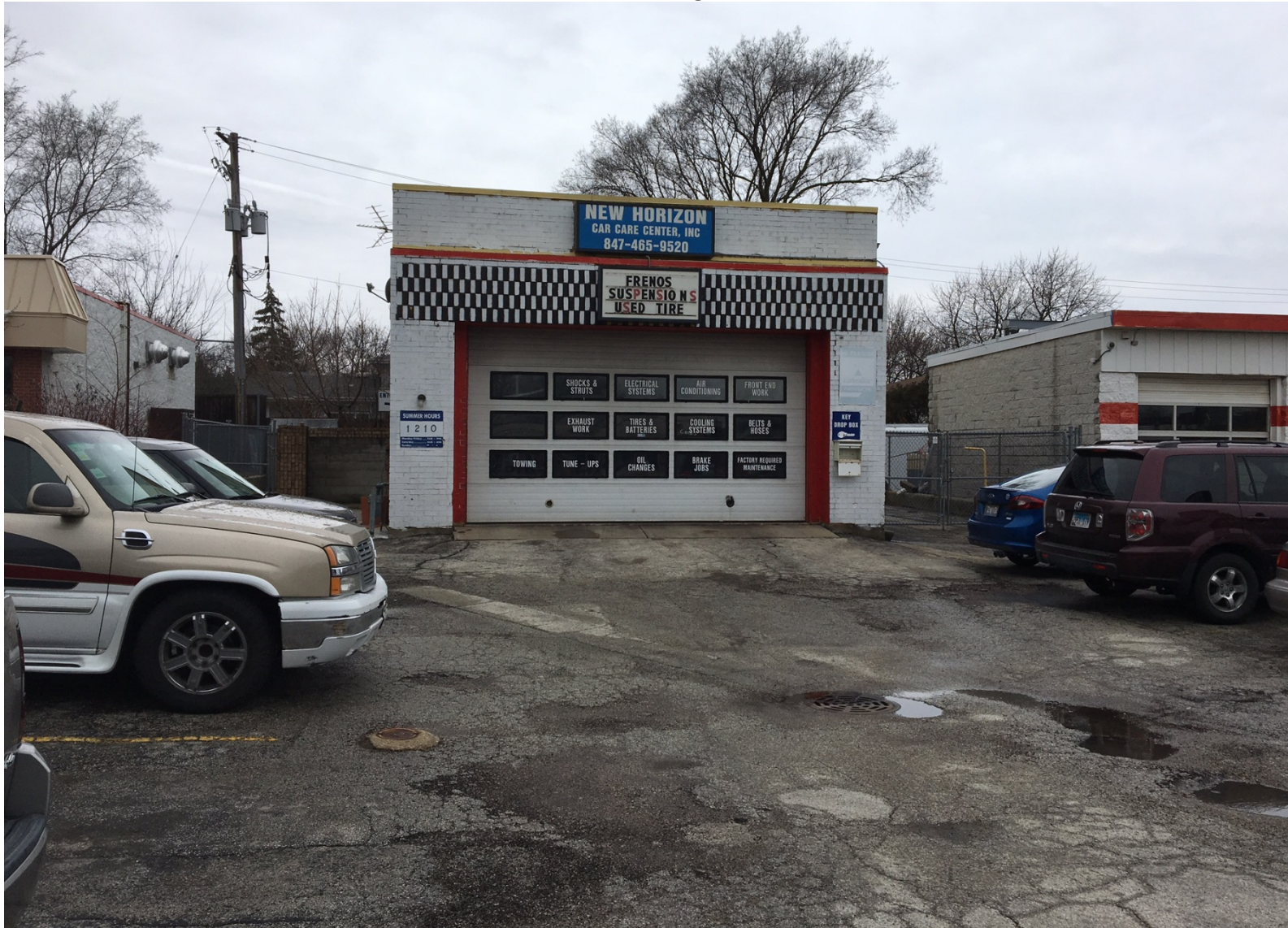
Existing conditions of building front (looking west)
