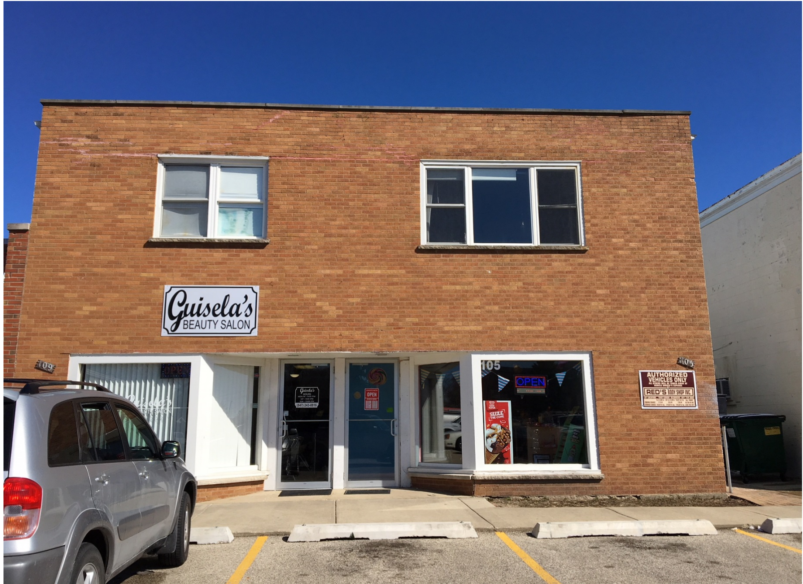
Existing conditions of west facade
