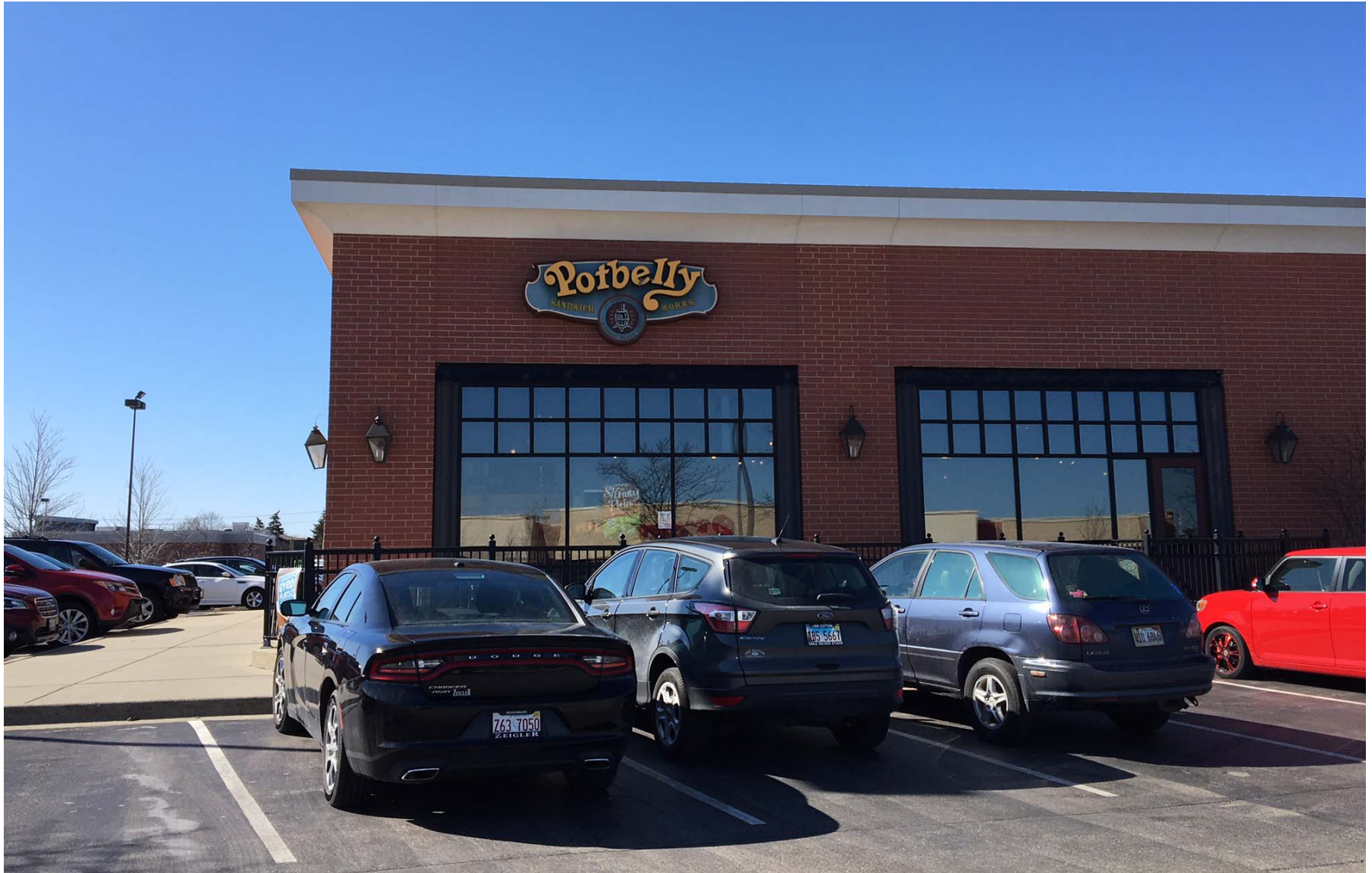
Existing conditions of east facade
