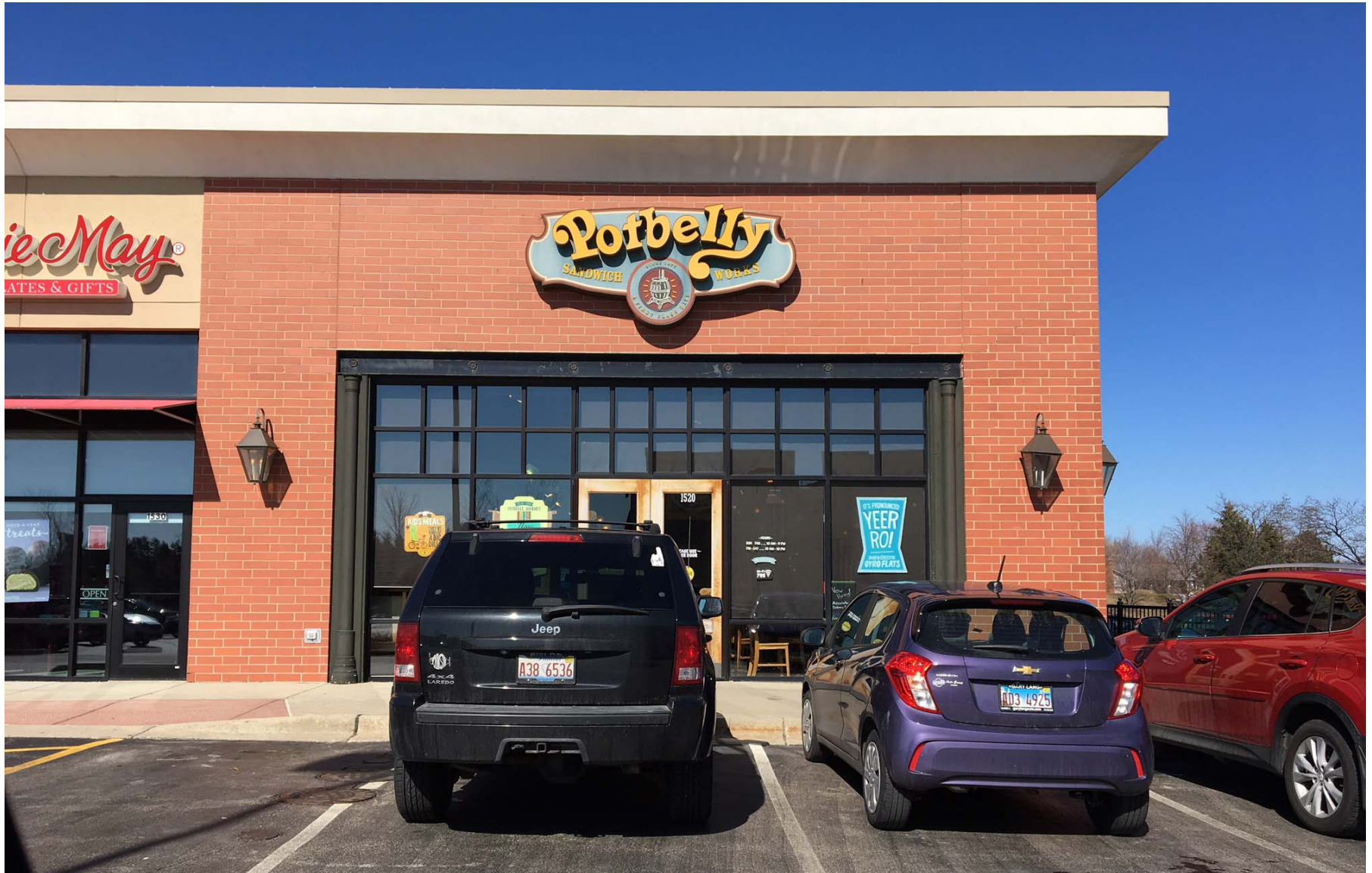
Existing conditions of south facade
