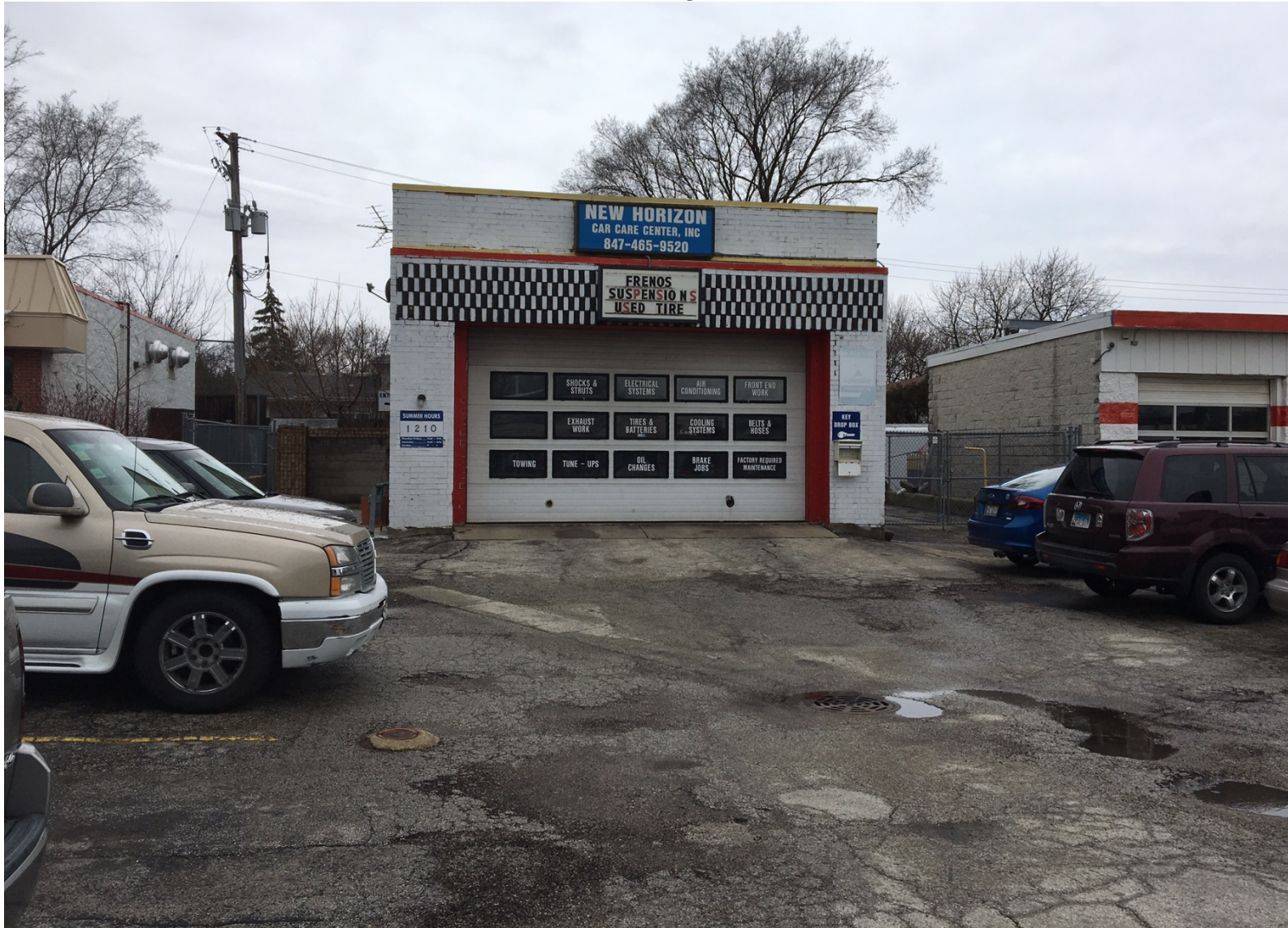
Existing conditions of building front (looking west)
