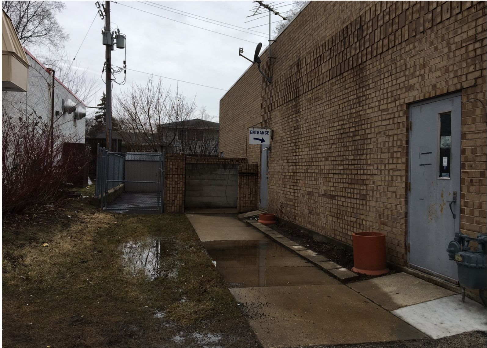
Existing conditions of south side of building (looking west)
