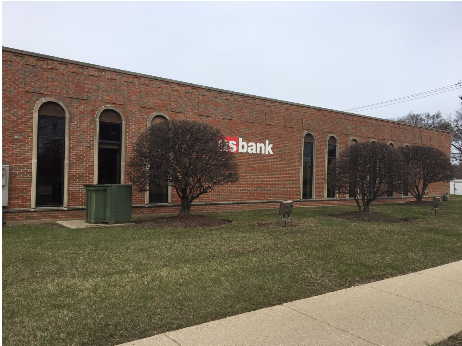
Existing conditions of east façade along Wheeling Road
