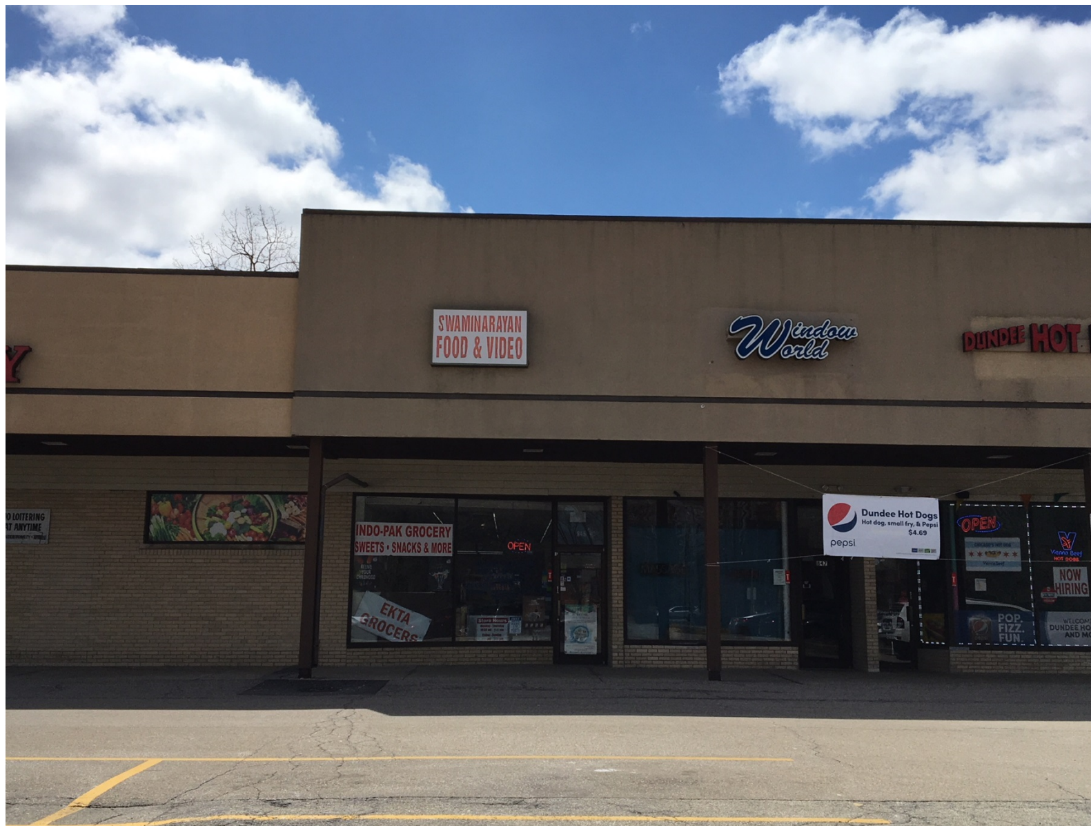
Existing conditions of subject unit (looking south)
