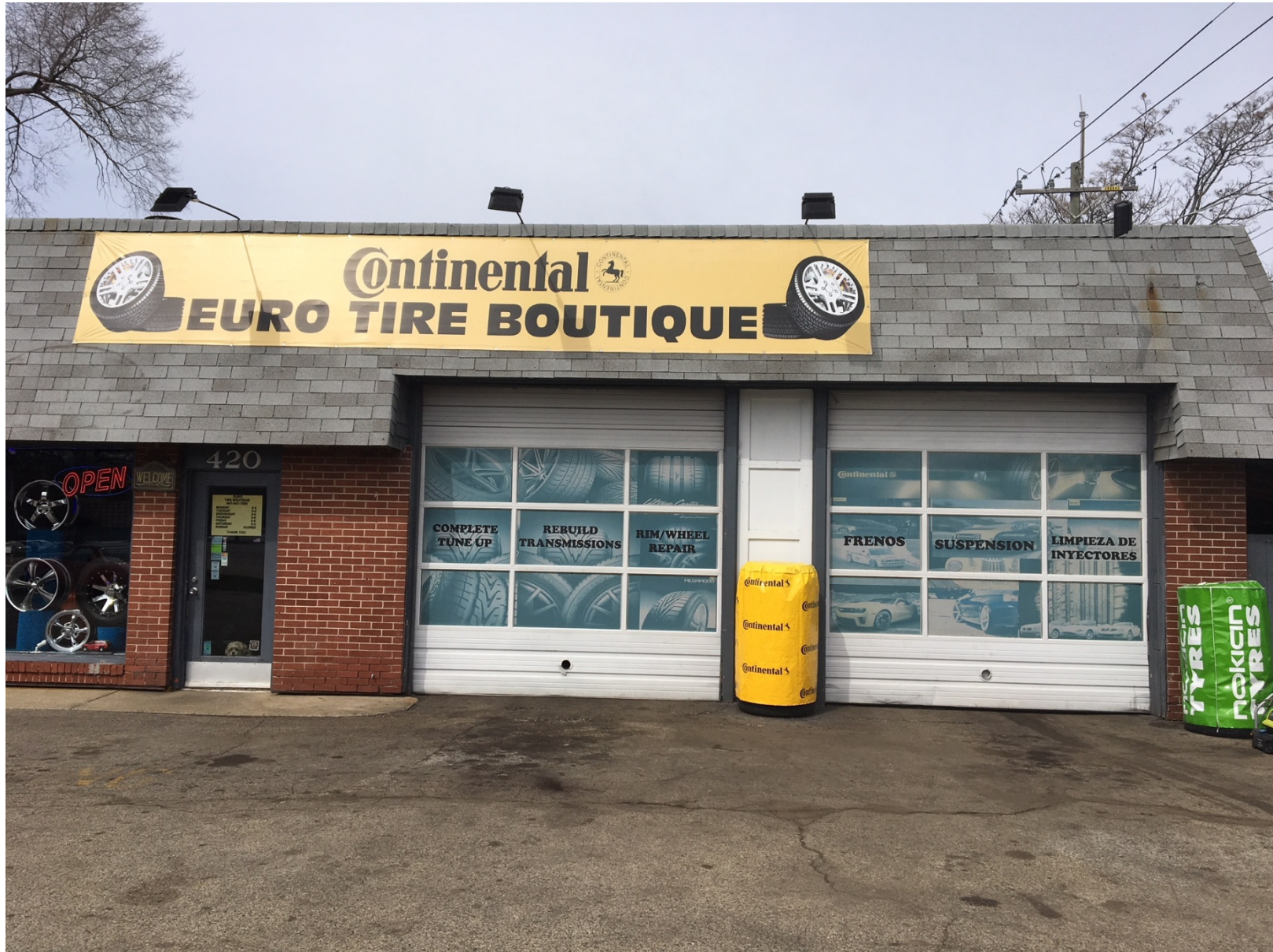
Existing conditions of building – looking west
