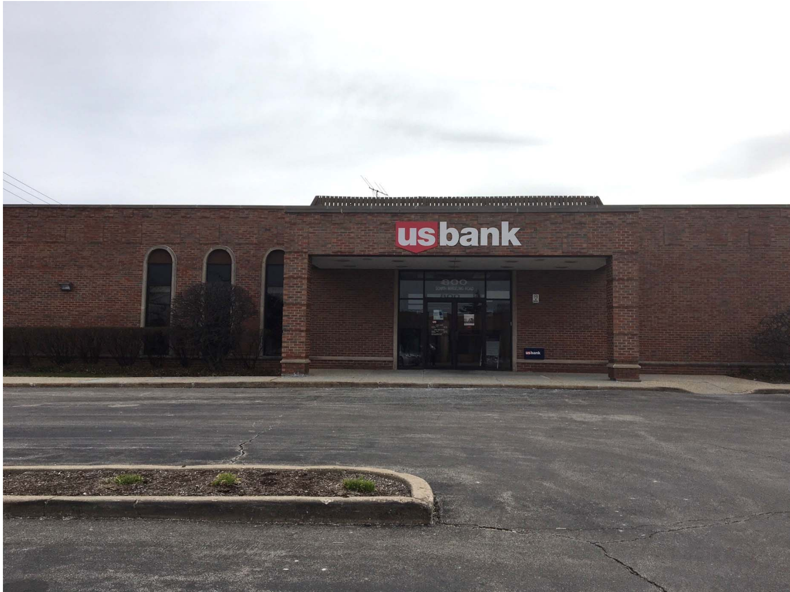
Existing conditions of building entry – west facade
