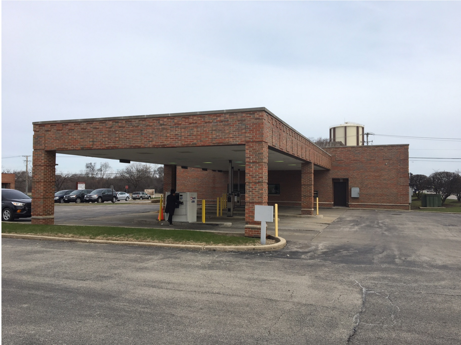
Existing conditions of south façade
