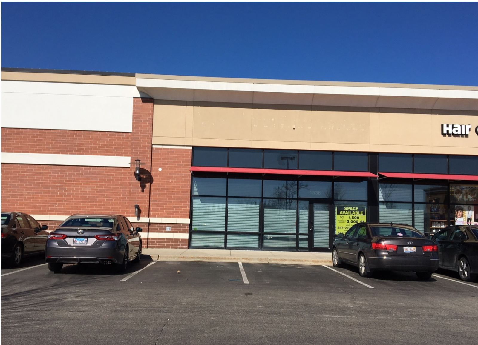
Existing conditions of subject unit (looking north)
