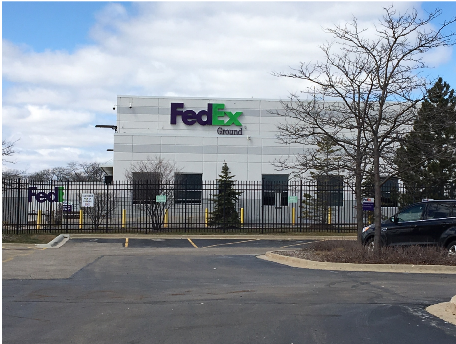
Existing conditions of subject unit (looking west)
