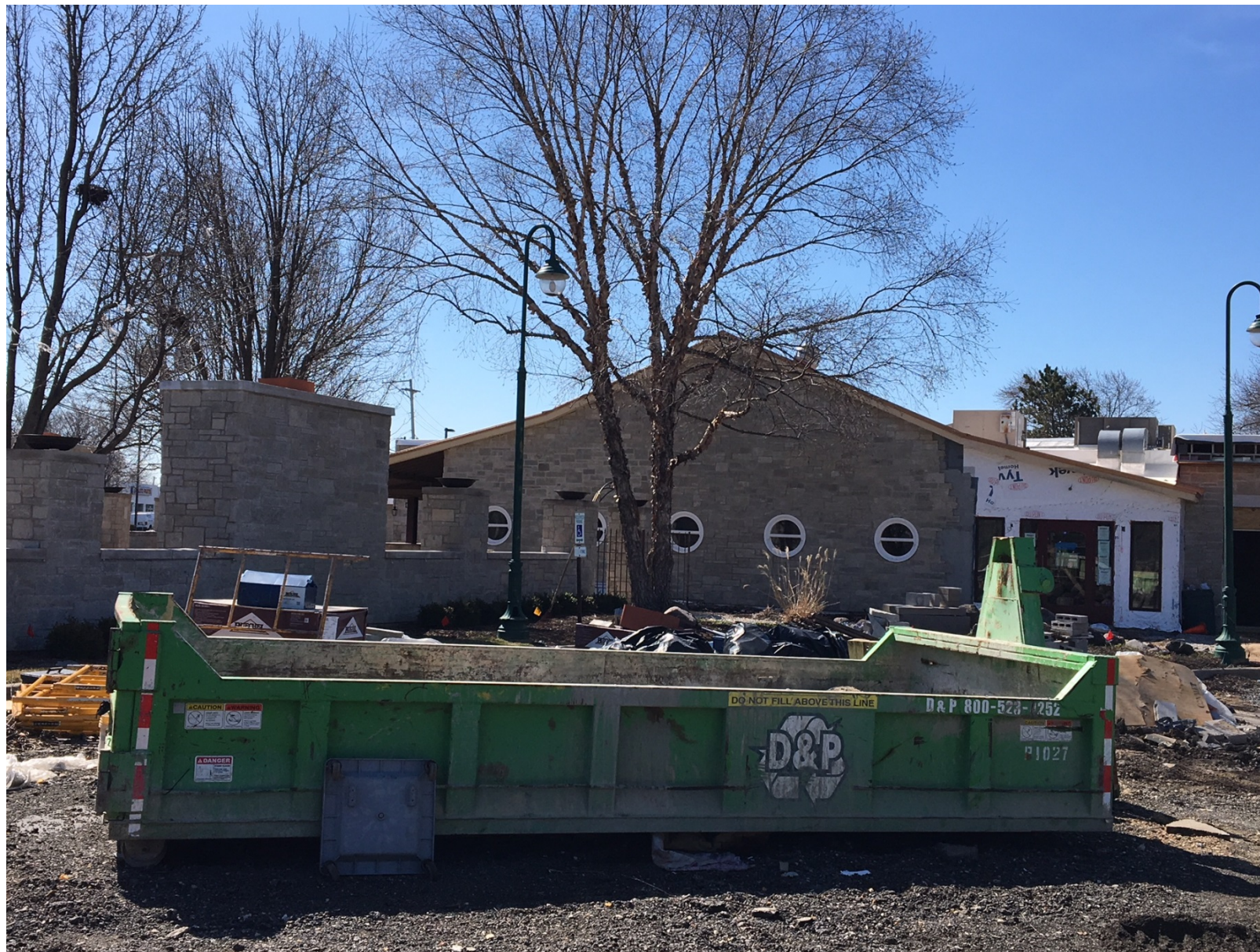
Existing conditions of north facade (taken from parking lot)
