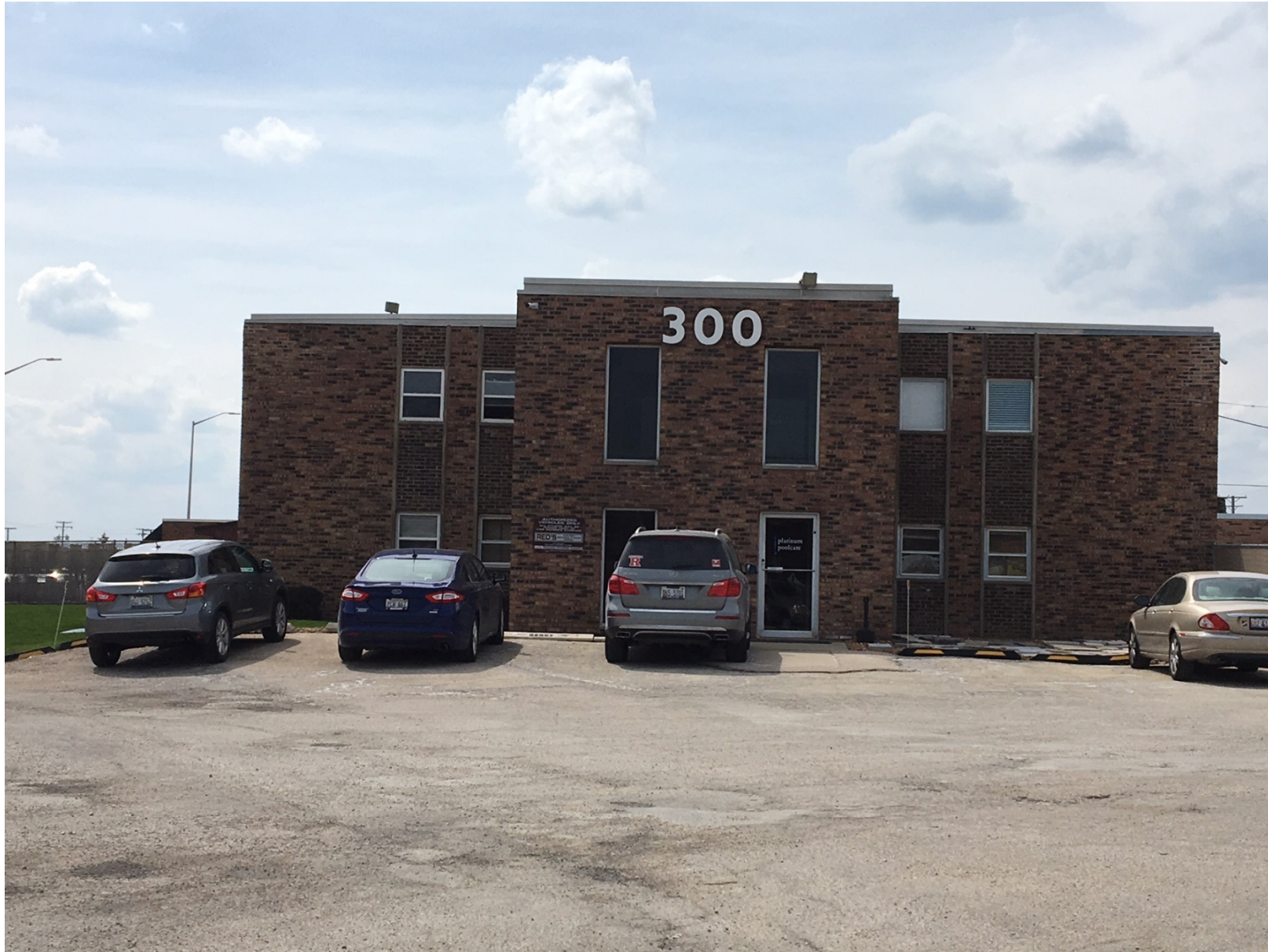
Existing conditions of subject property (looking west)
