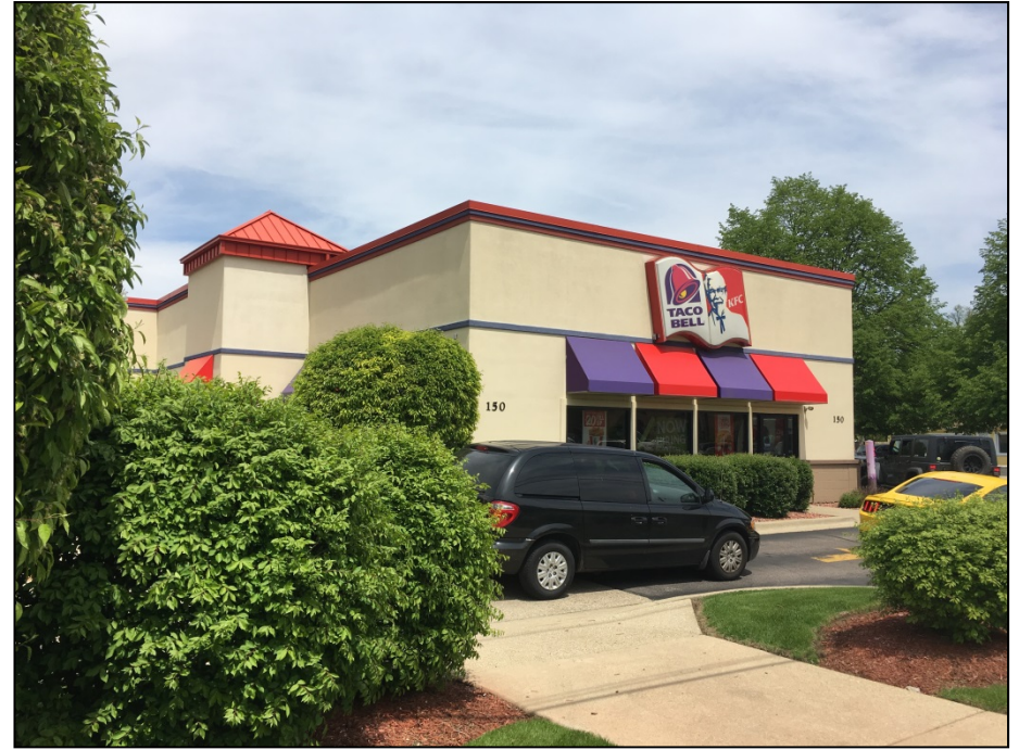
Existing conditions south elevation from southwest
