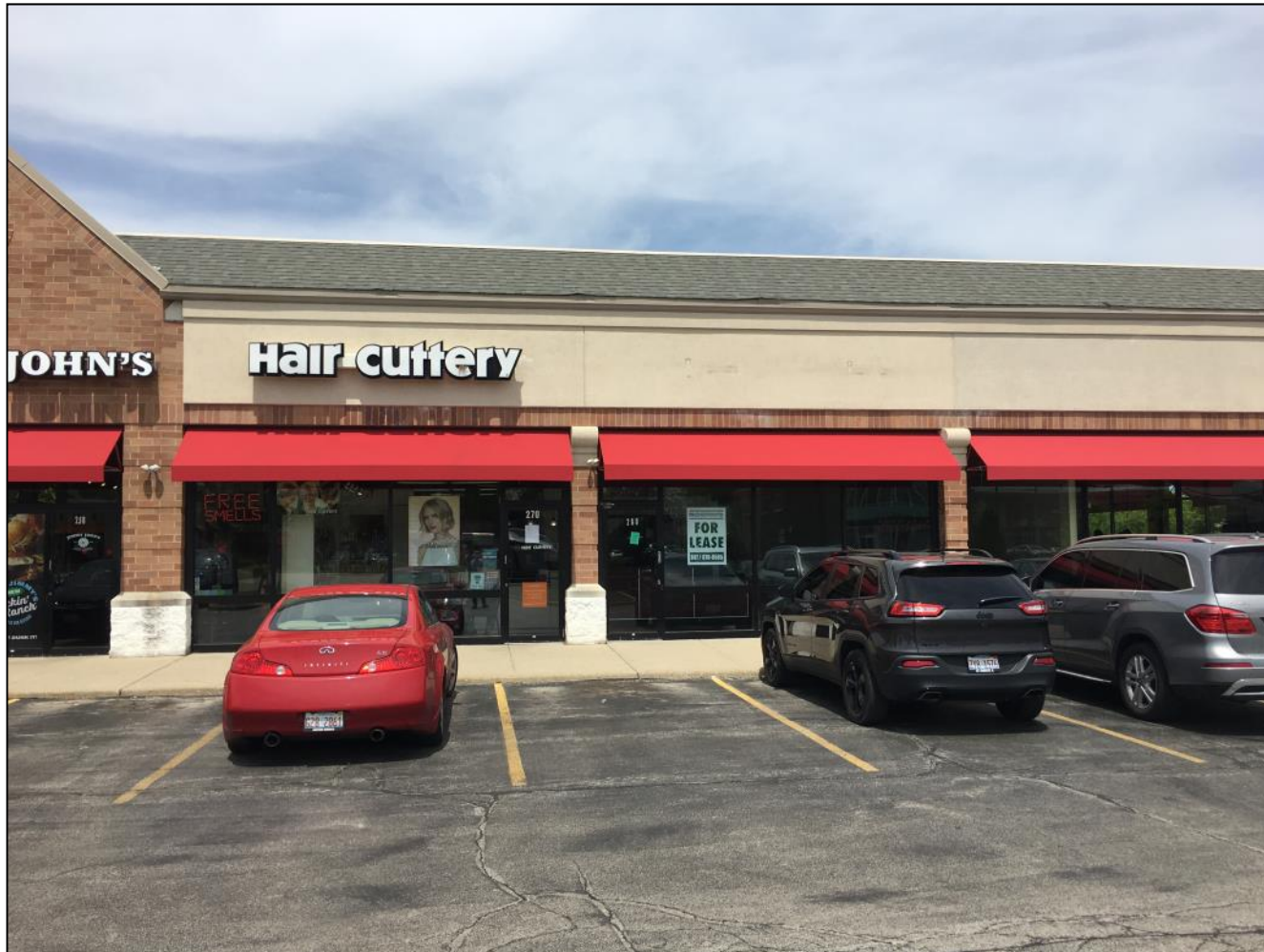
Existing conditions – south elevation
