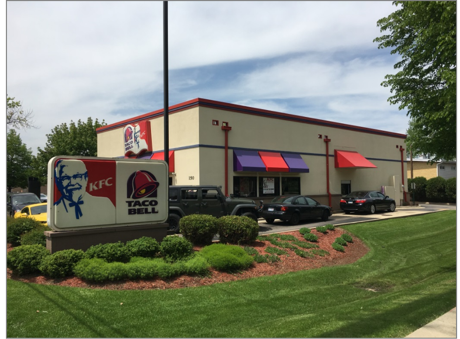
Existing conditions View of west elevation
