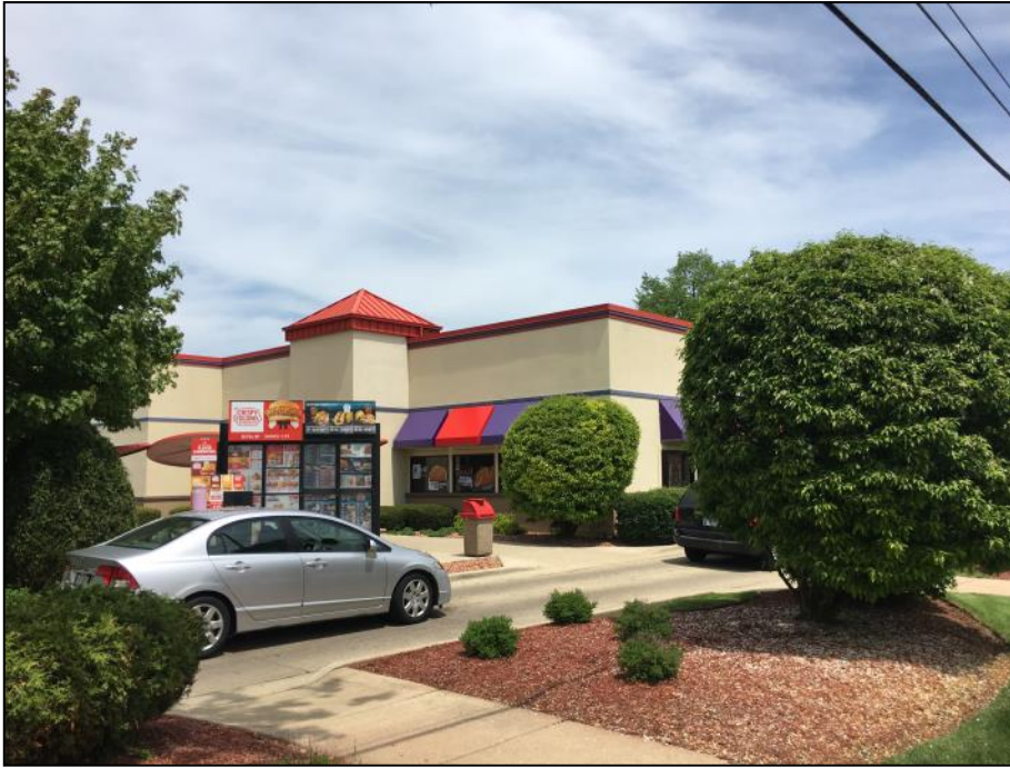
Existing conditions west elevation from southwest
