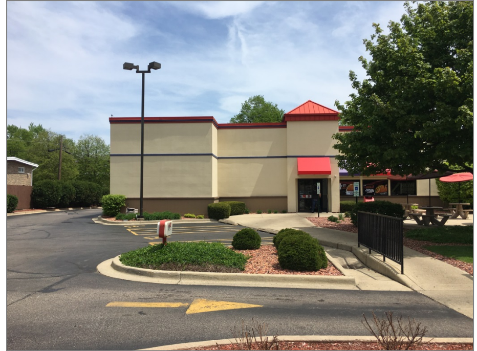
Existing conditions View of west elevation
