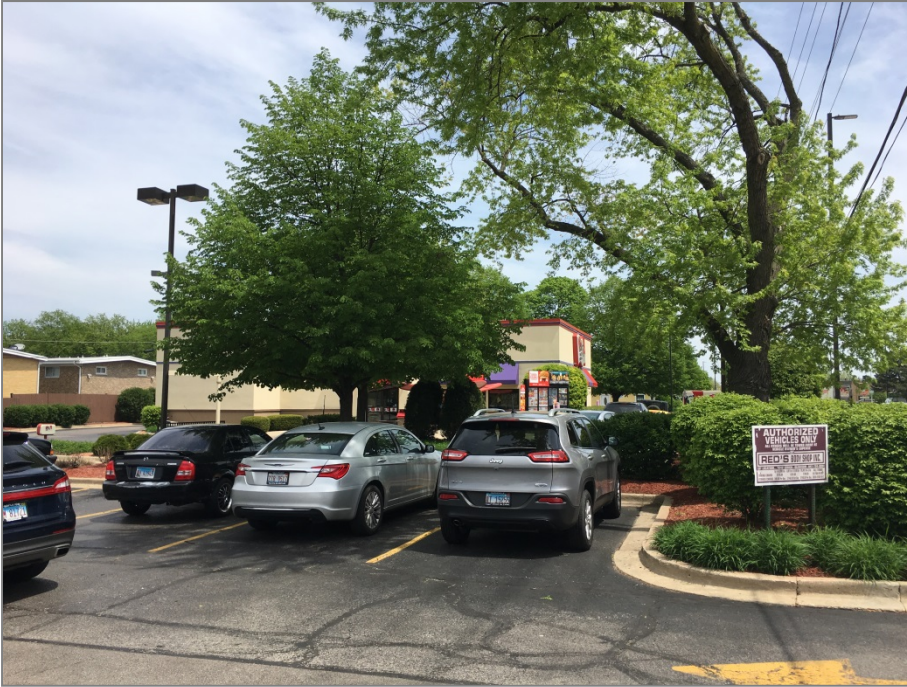
Existing conditions View of west elevation (from northwest)
