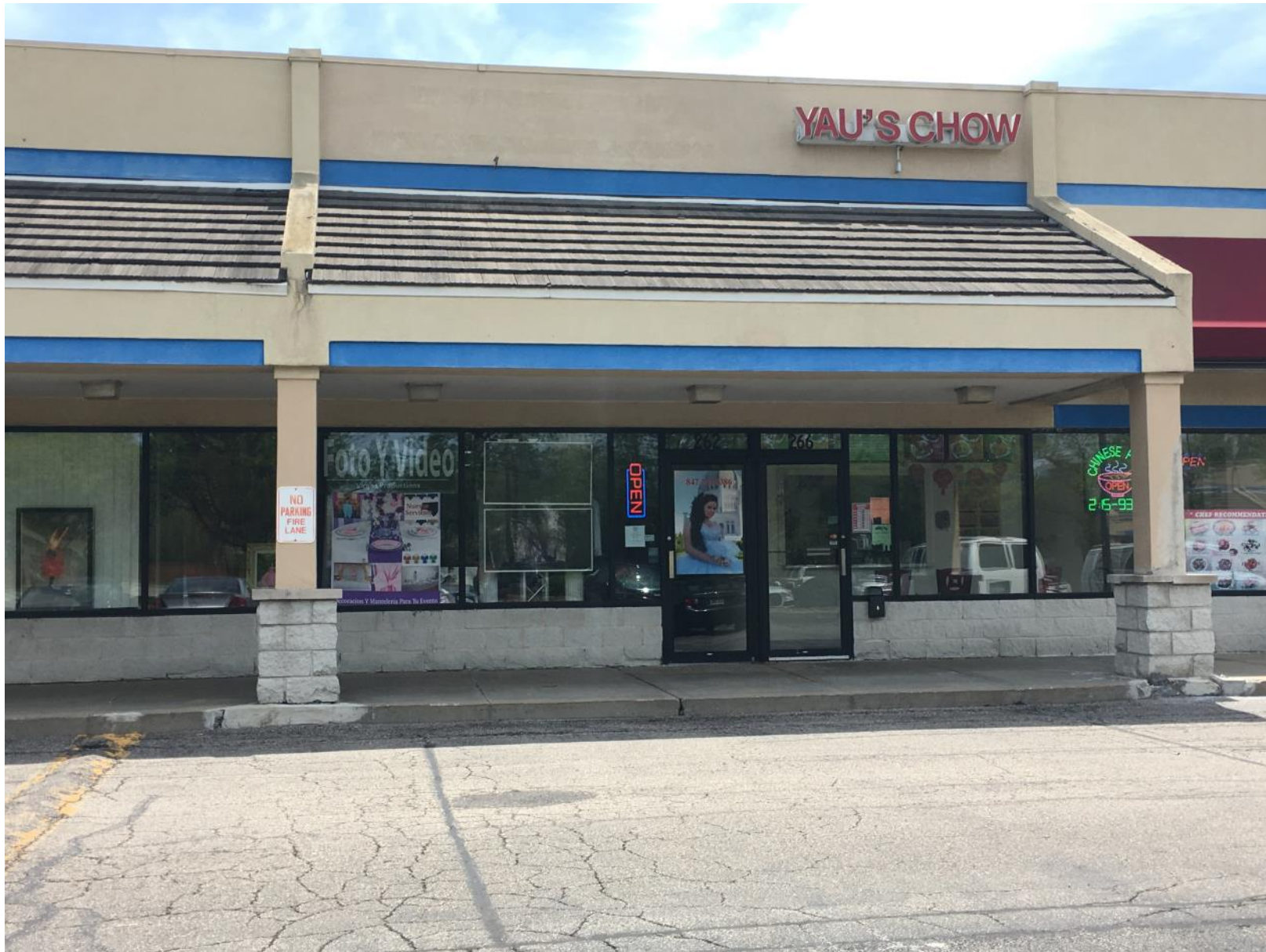
Existing conditions of subject property (looking southwest)
