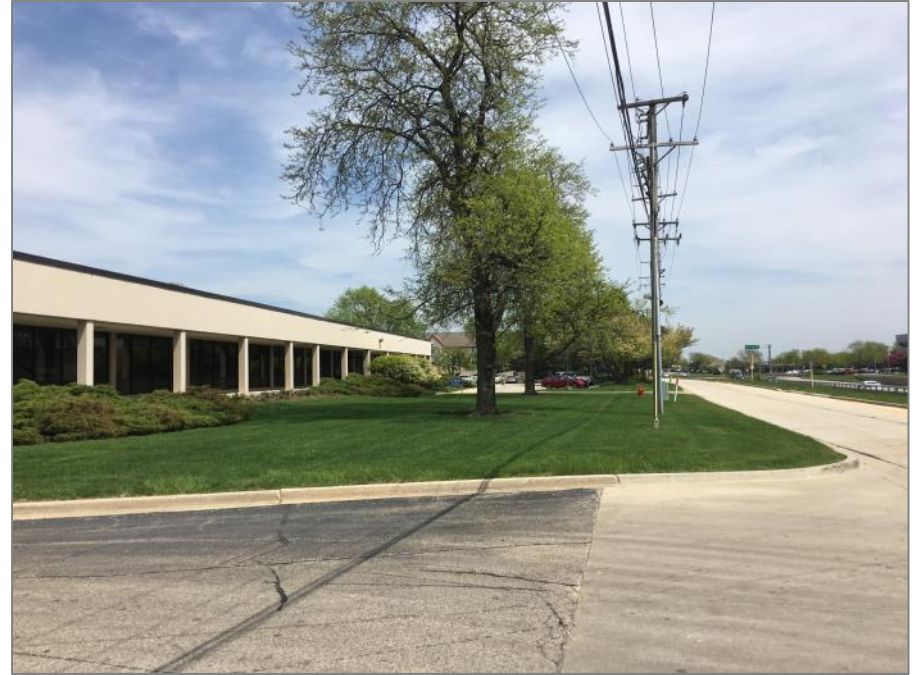
Existing conditions – view from eastbound frontage road (one way street, west)
