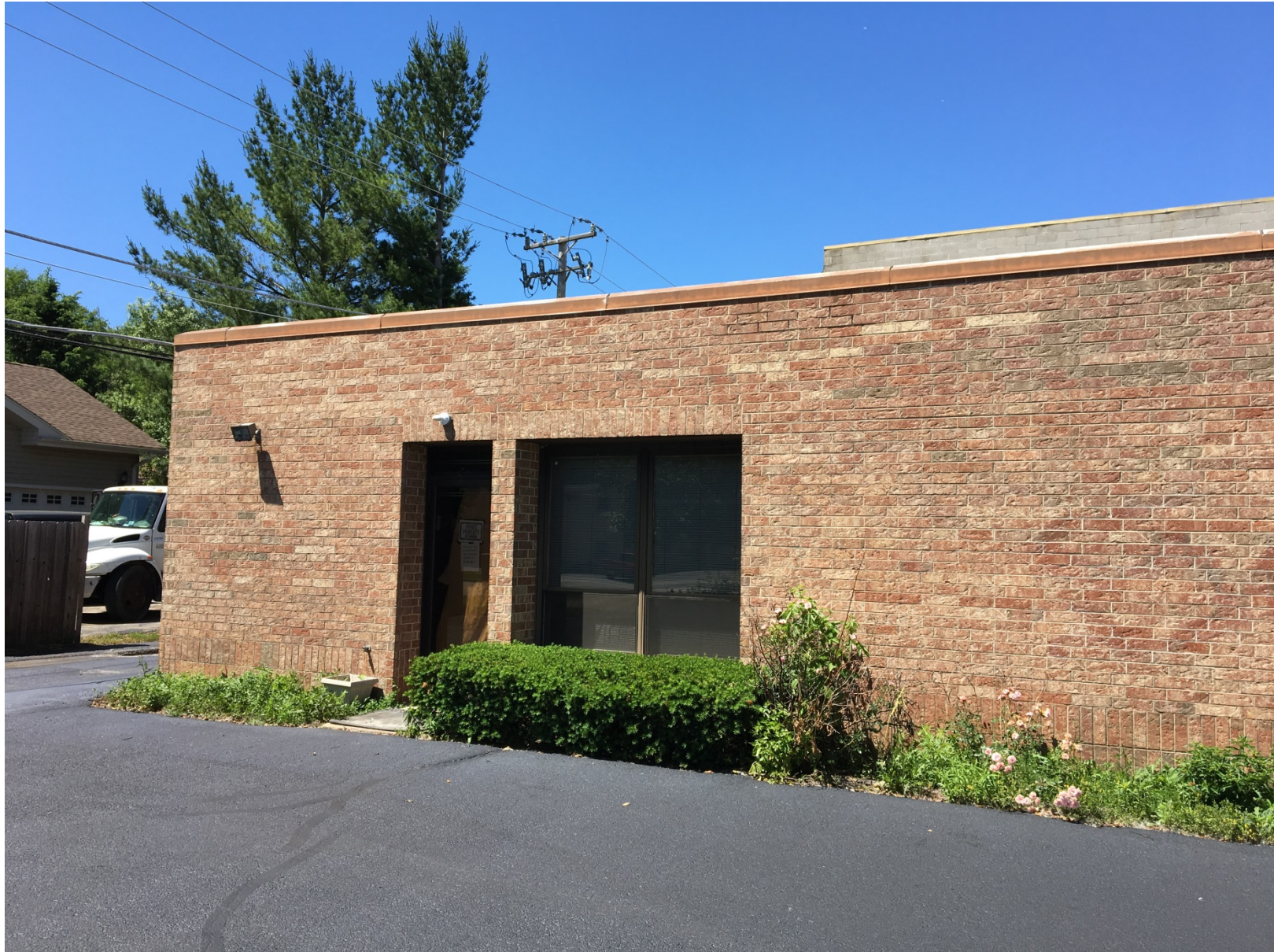
Existing conditions of south facade of subject property (looking north)
