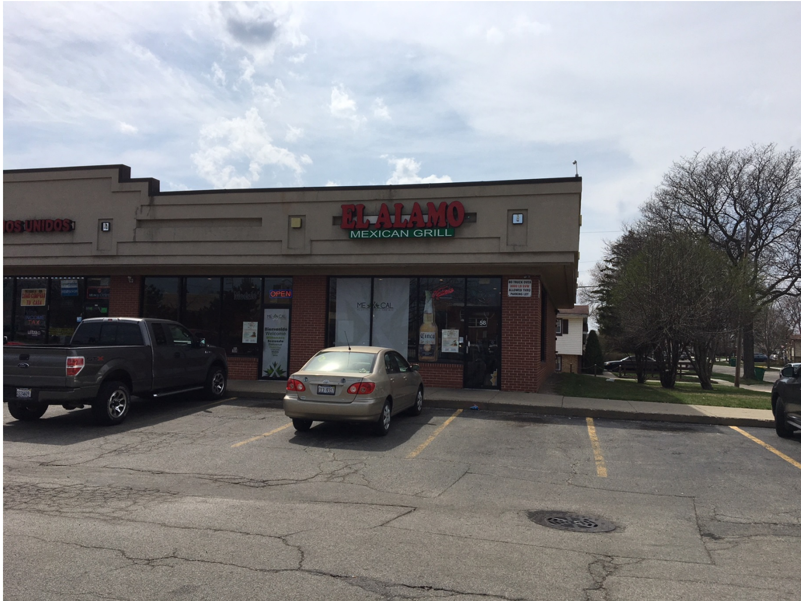
Existing conditions of subject unit (looking west)
