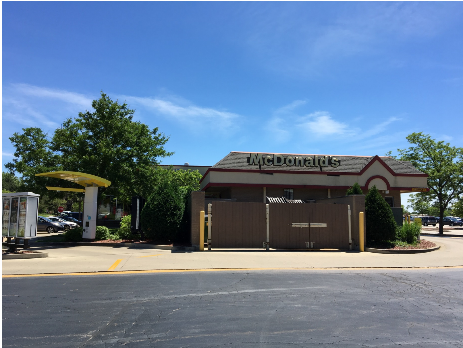
Existing conditions of property looking south
