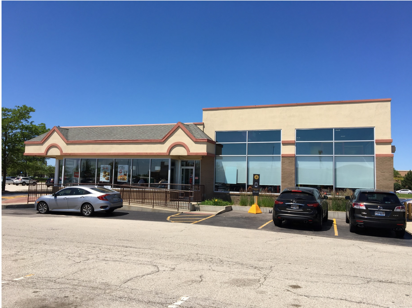
Existing conditions of property looking north
