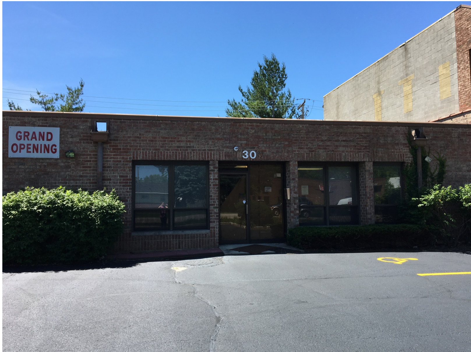
Existing conditions of east facade of subject property (looking west)
