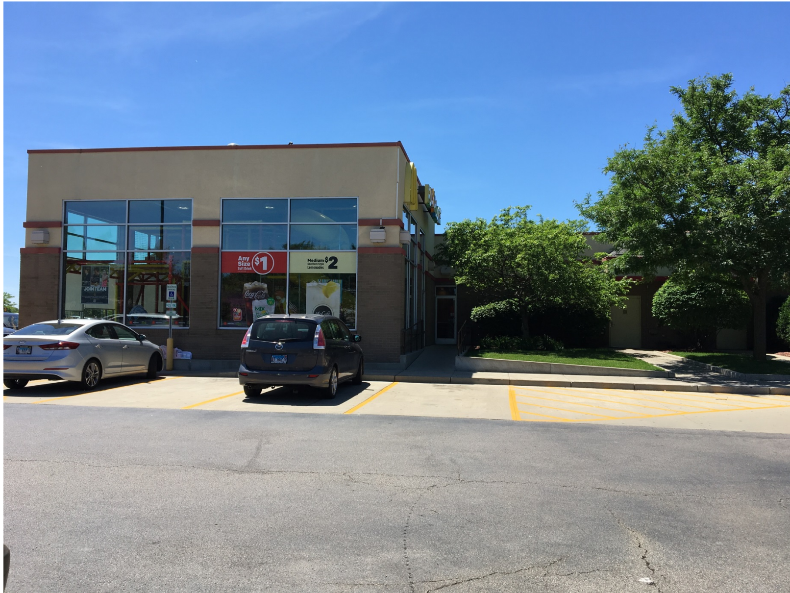
Existing conditions of property looking west
