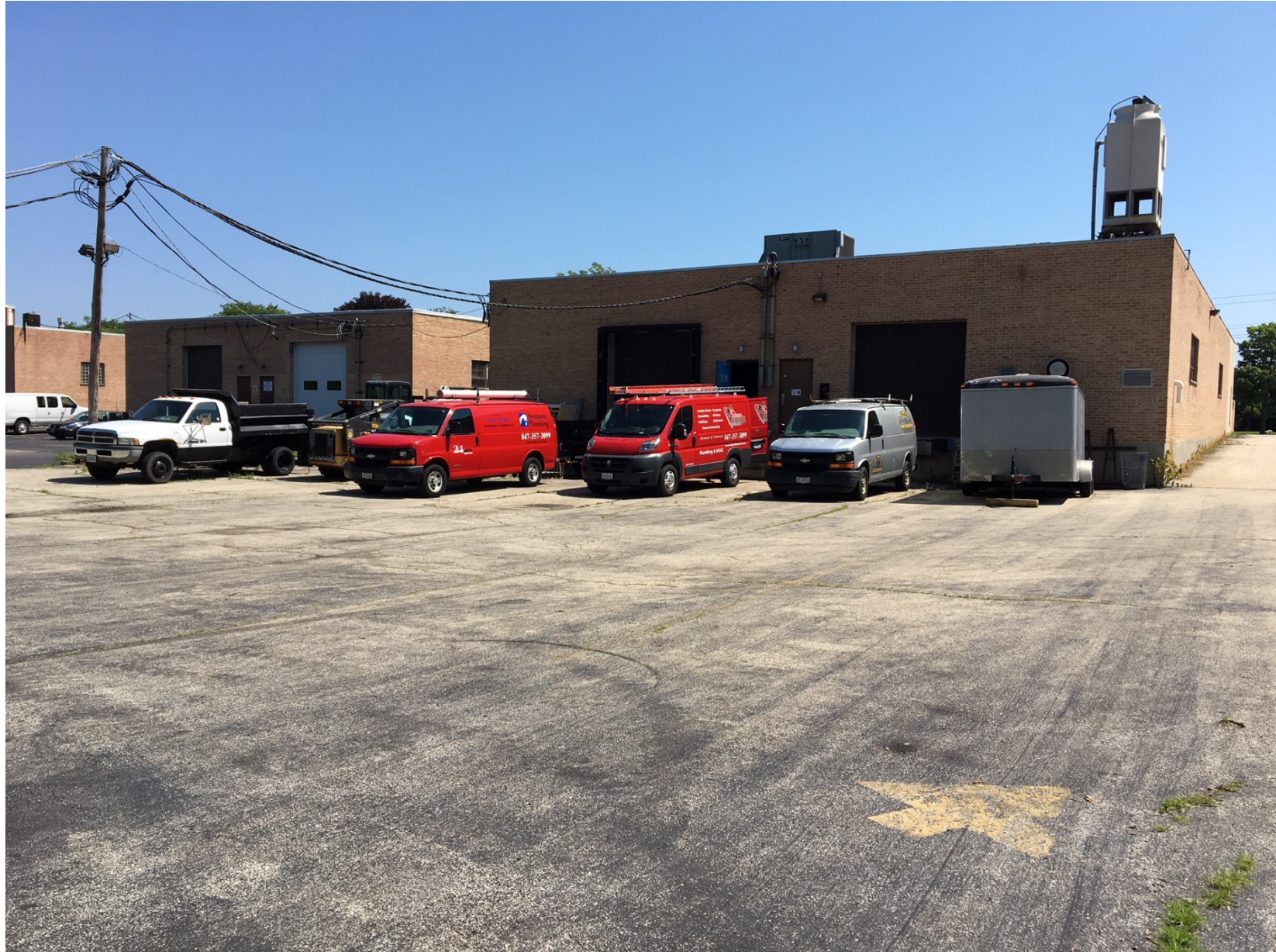
Existing conditions of rear of building
