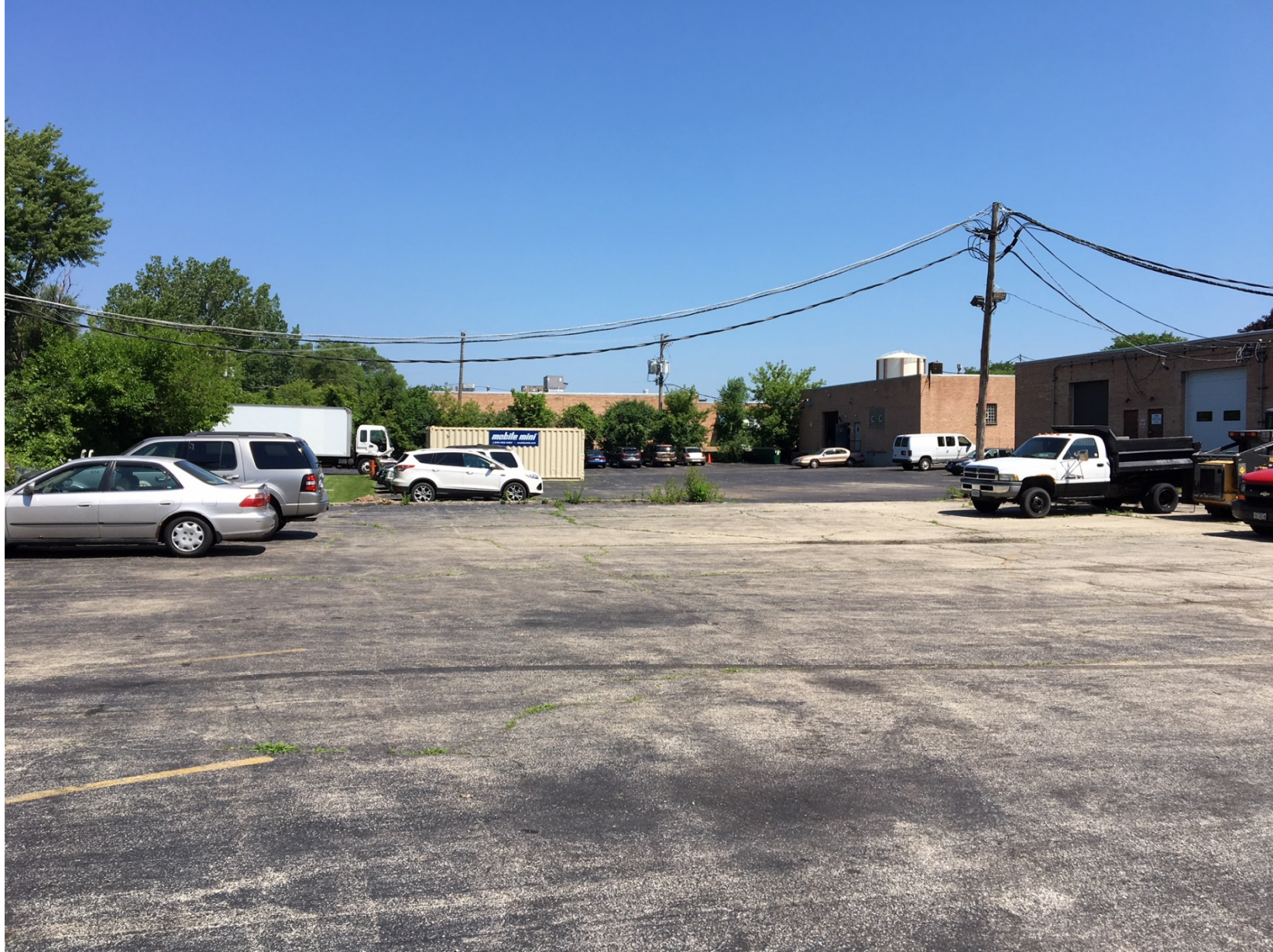
Existing conditions of rear parking lot – looking north
