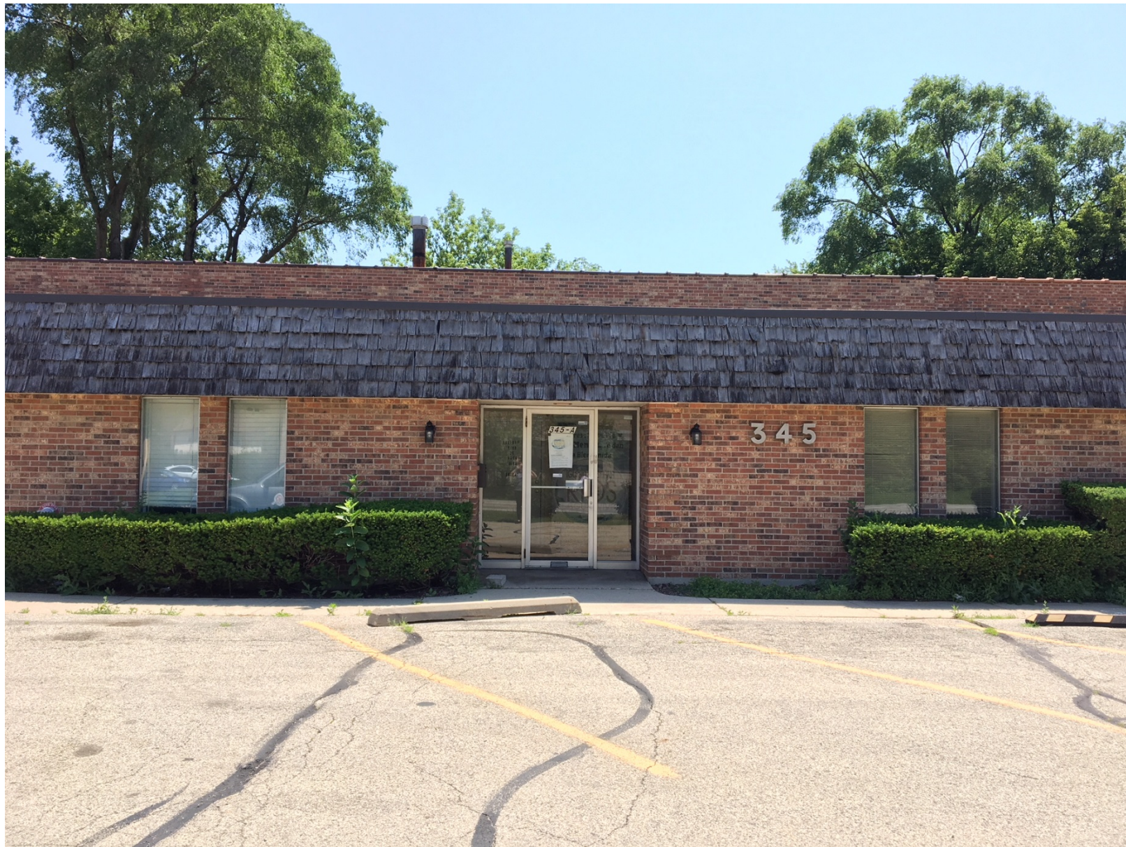
Existing conditions of building entry (looking east)
