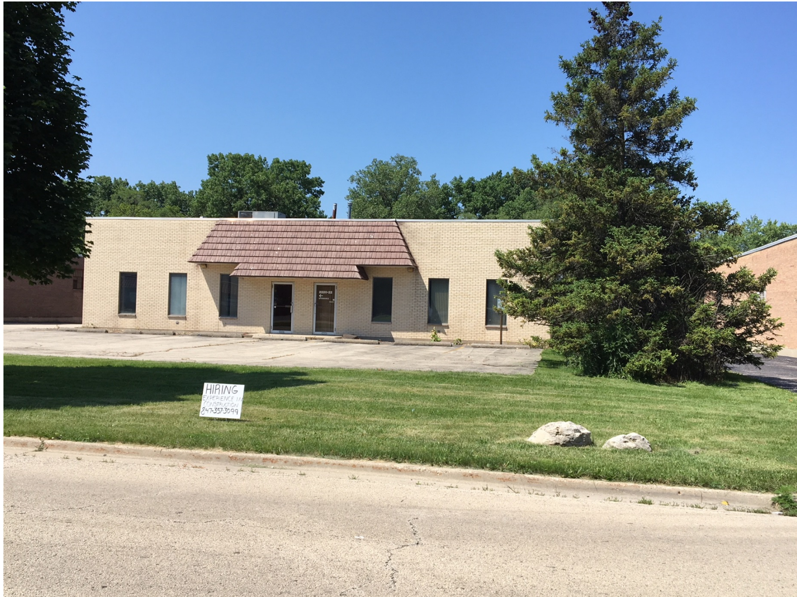
Existing conditions – east elevation
