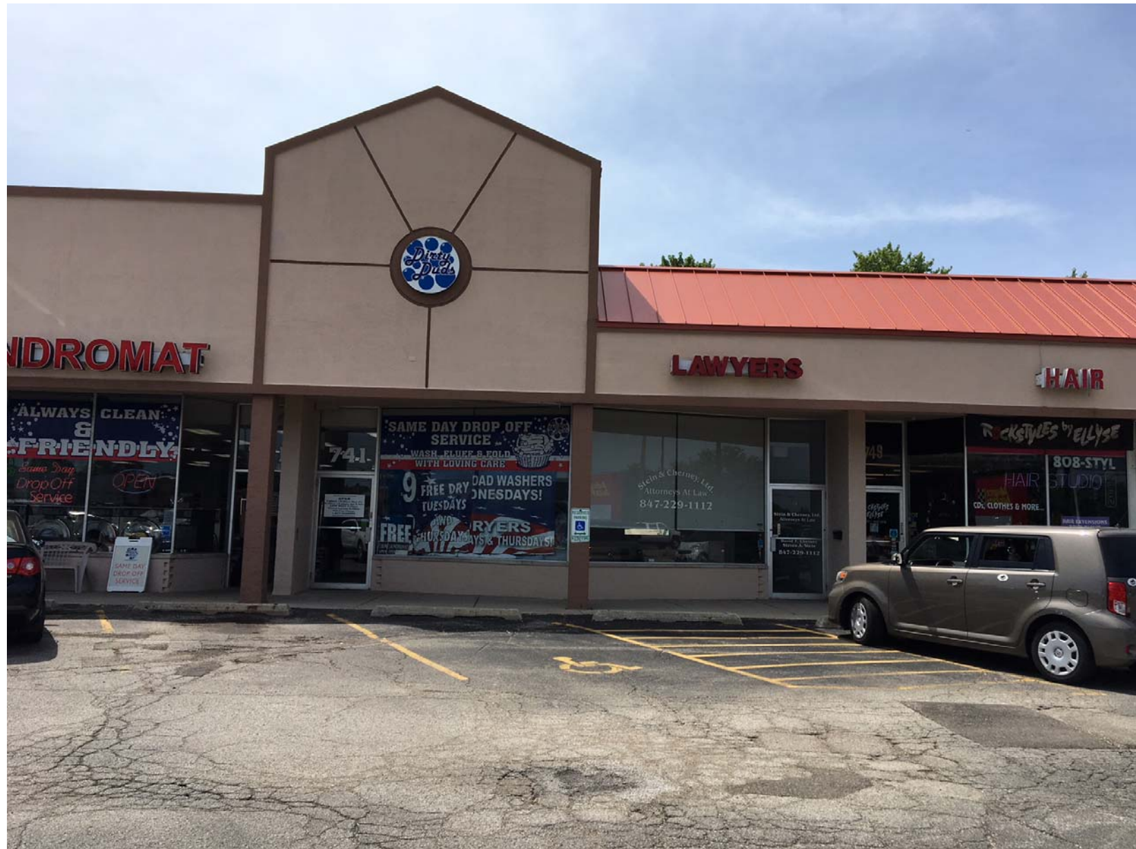
Existing conditions of subject unit (looking south)
