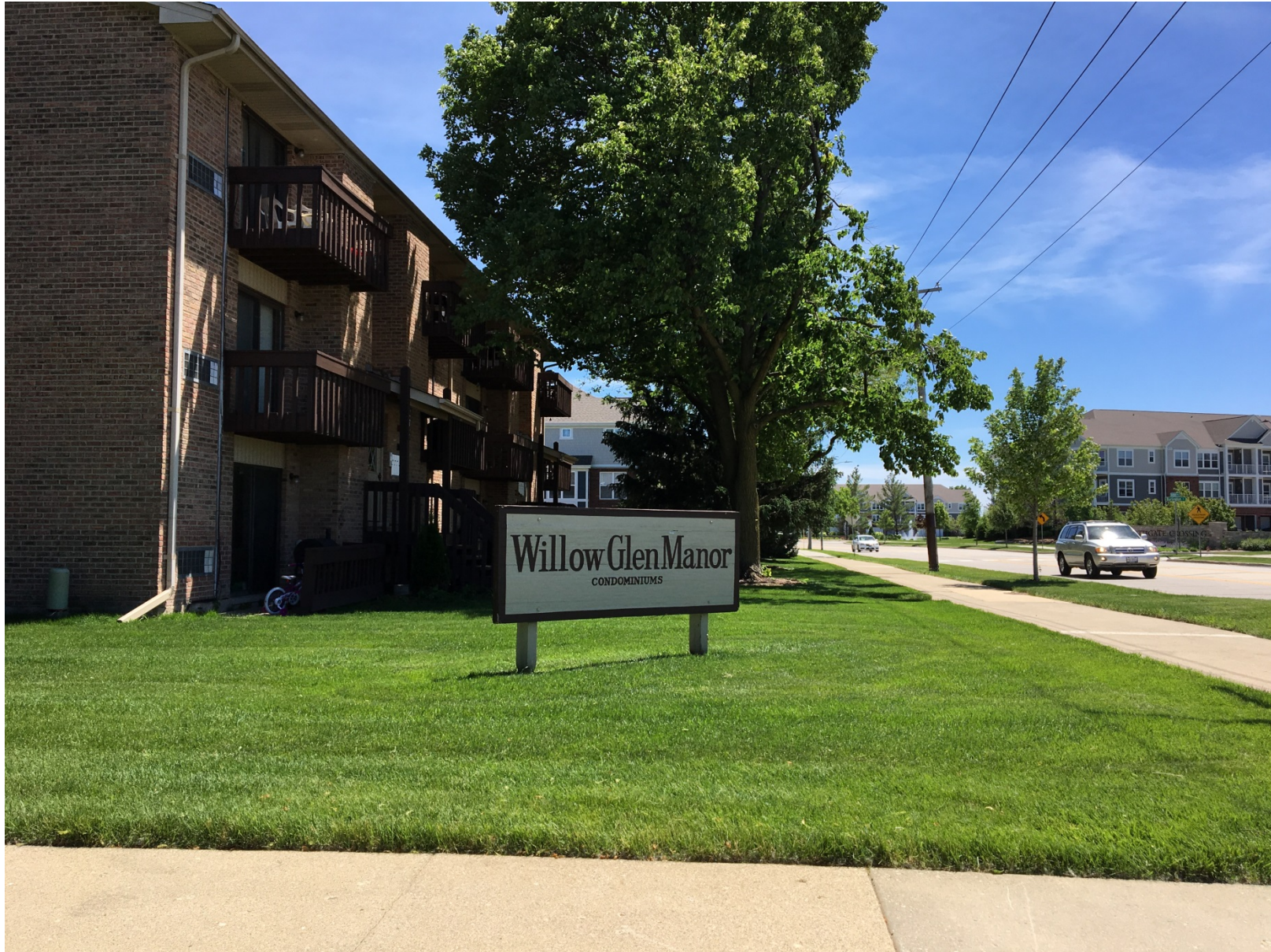
Existing conditions of sign (looking south)
