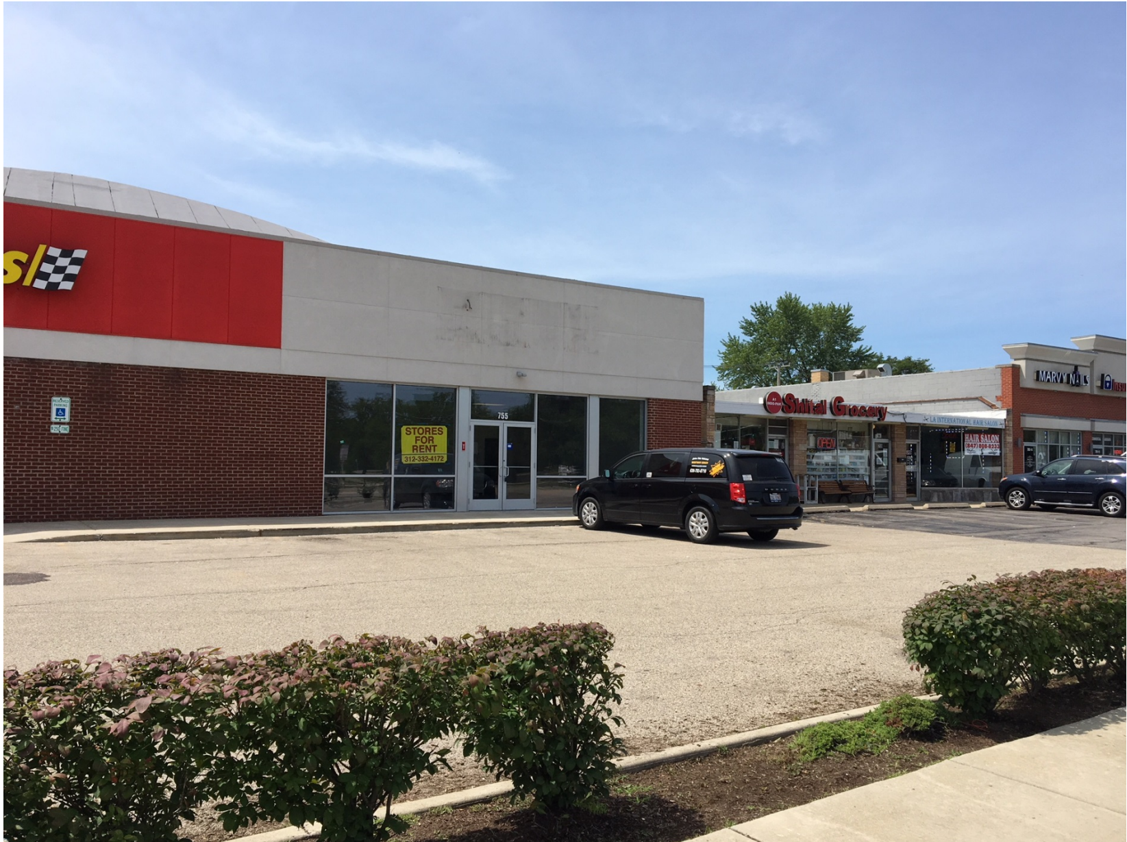
Existing conditions of subject unit (looking southwest)
