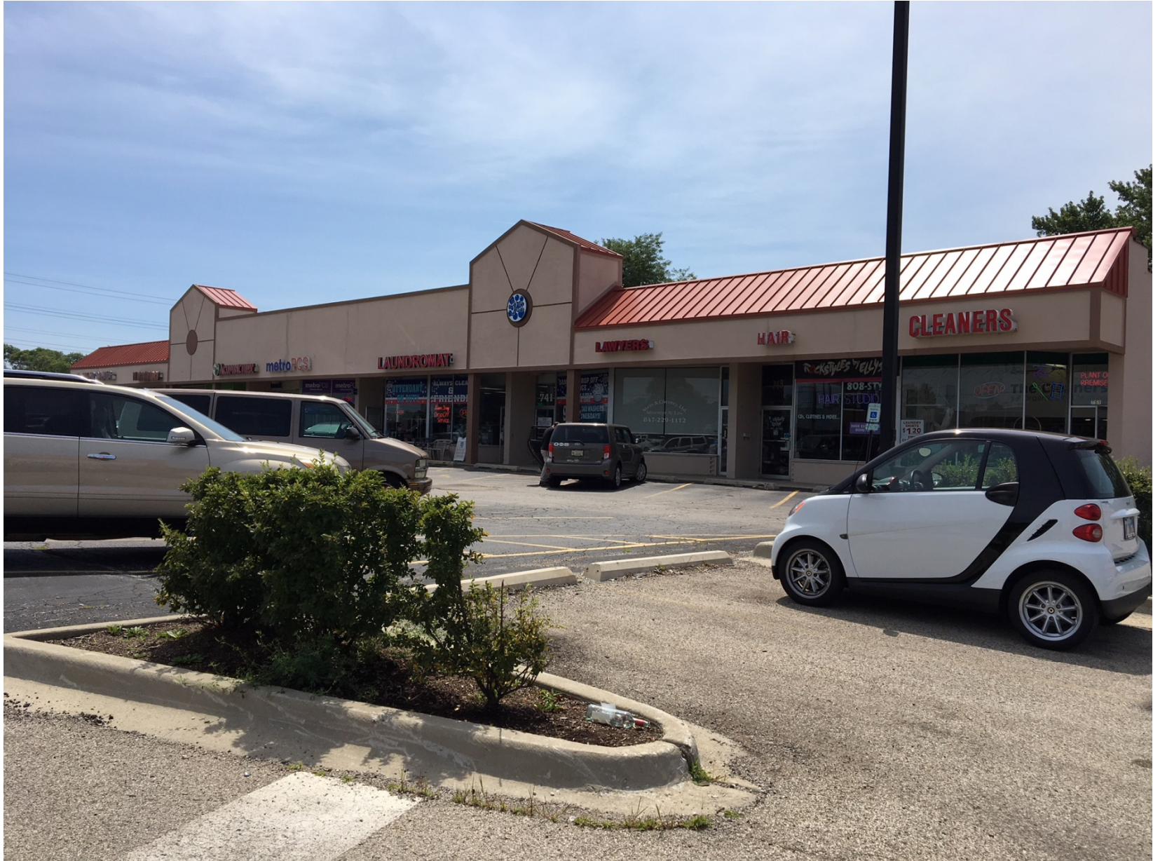
Existing conditions of a portion of parking on subject property (looking southeast)
