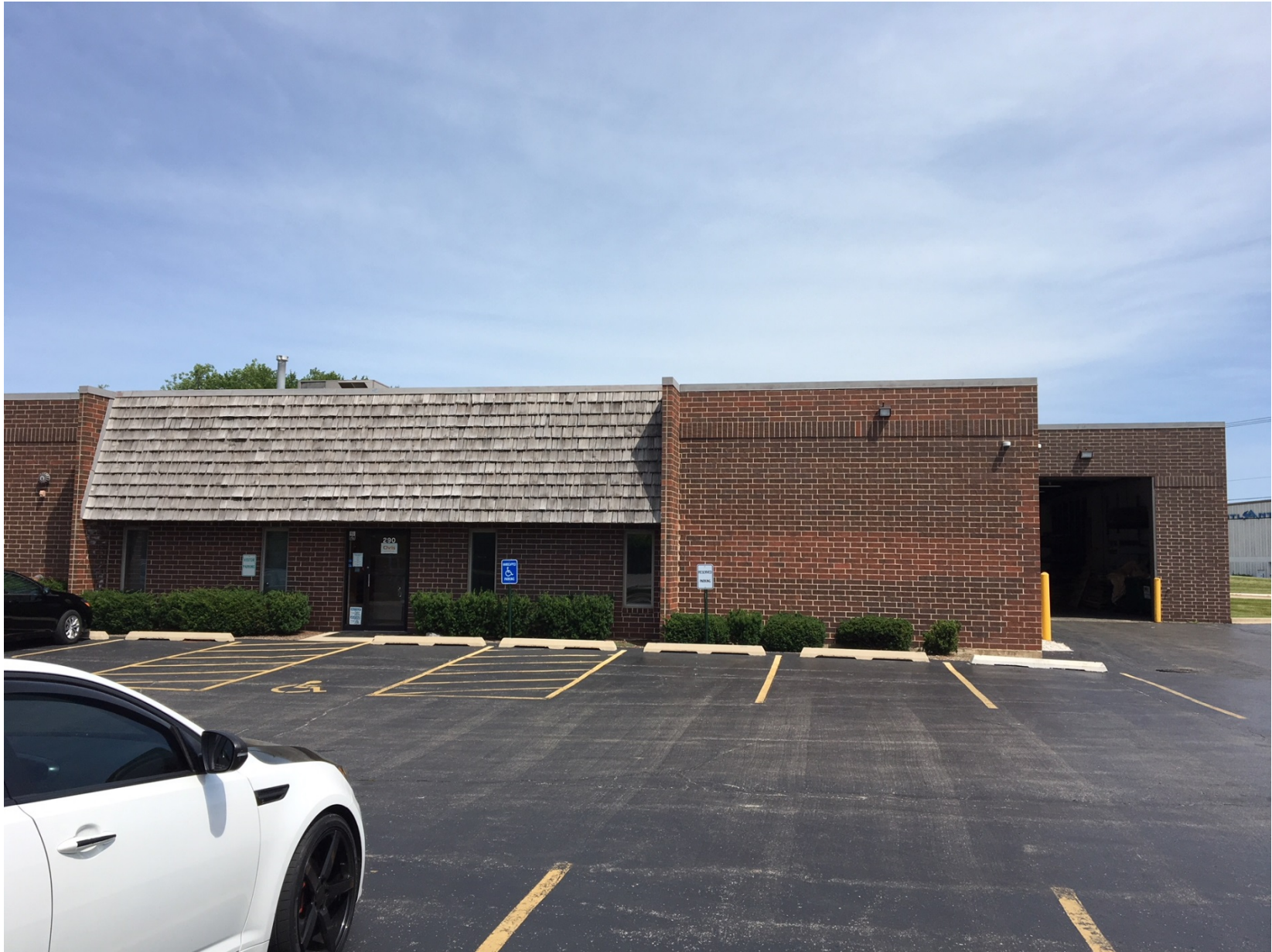
Existing conditions of subject property (looking north)
