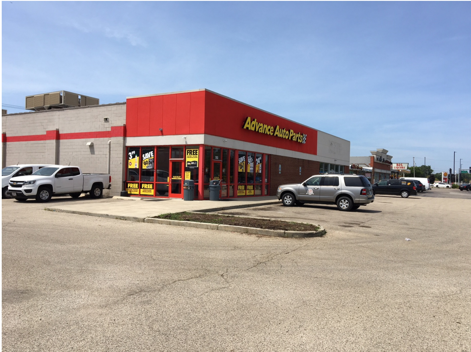
Existing conditions of subject property (looking west)
