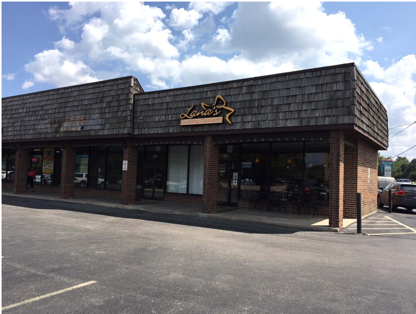
Existing conditions of subject units (looking south)
