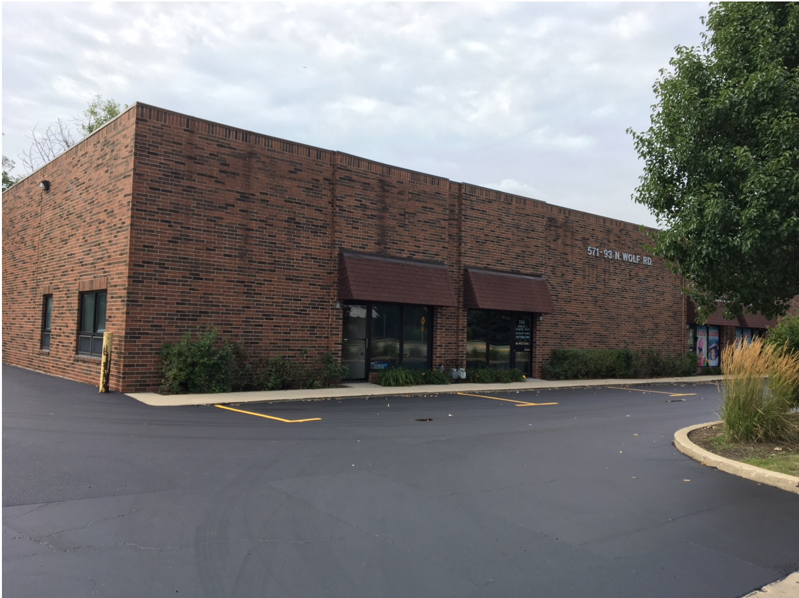
Existing conditions of subject unit (looking south)
