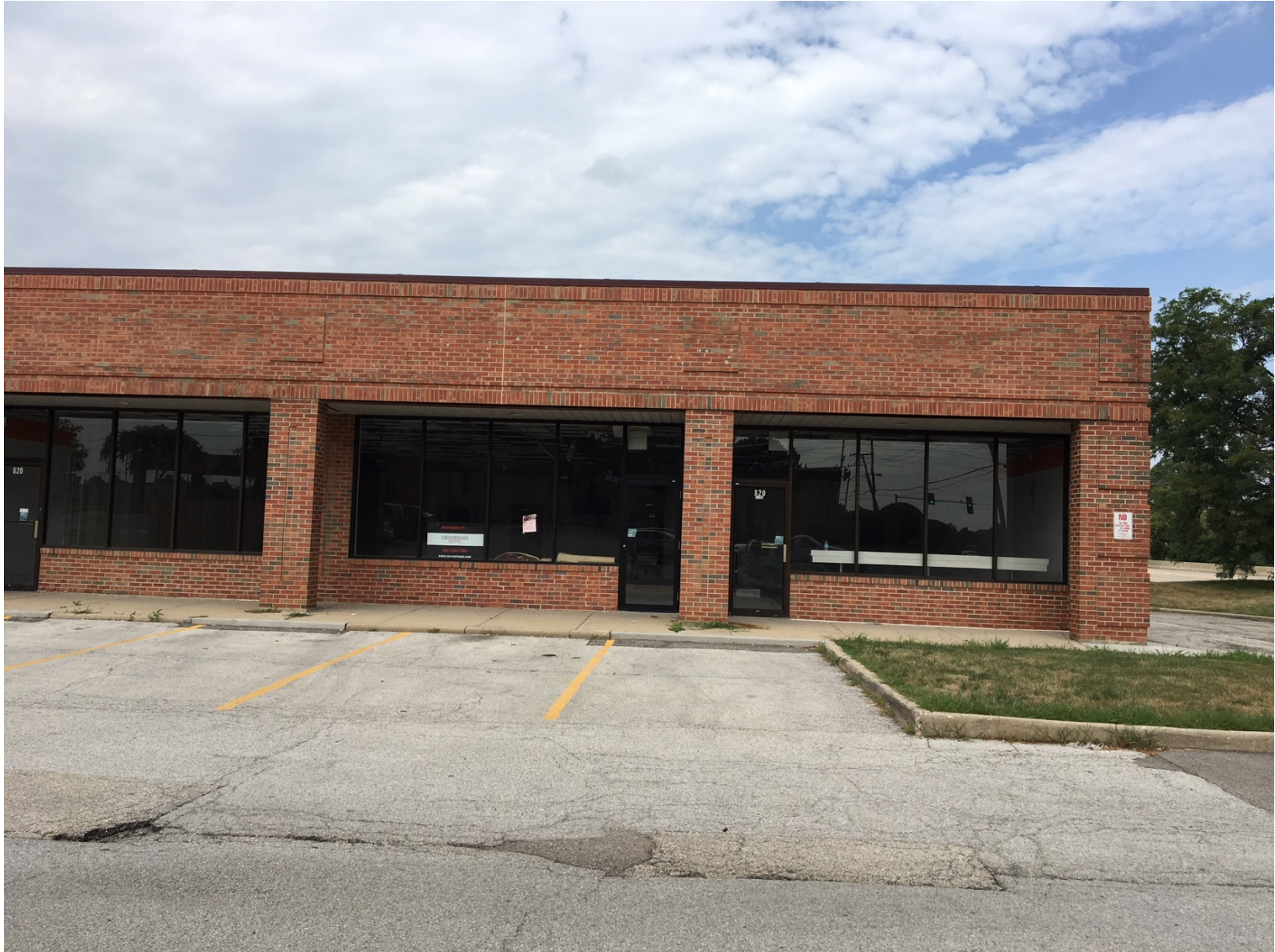
Existing conditions of subject unit (looking west)
