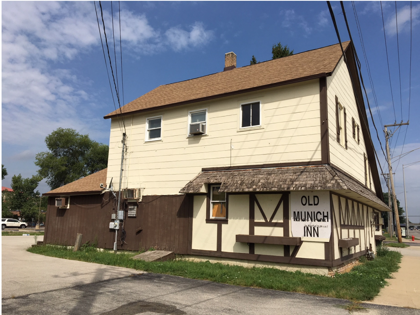
Existing conditions of south side (looking north)
