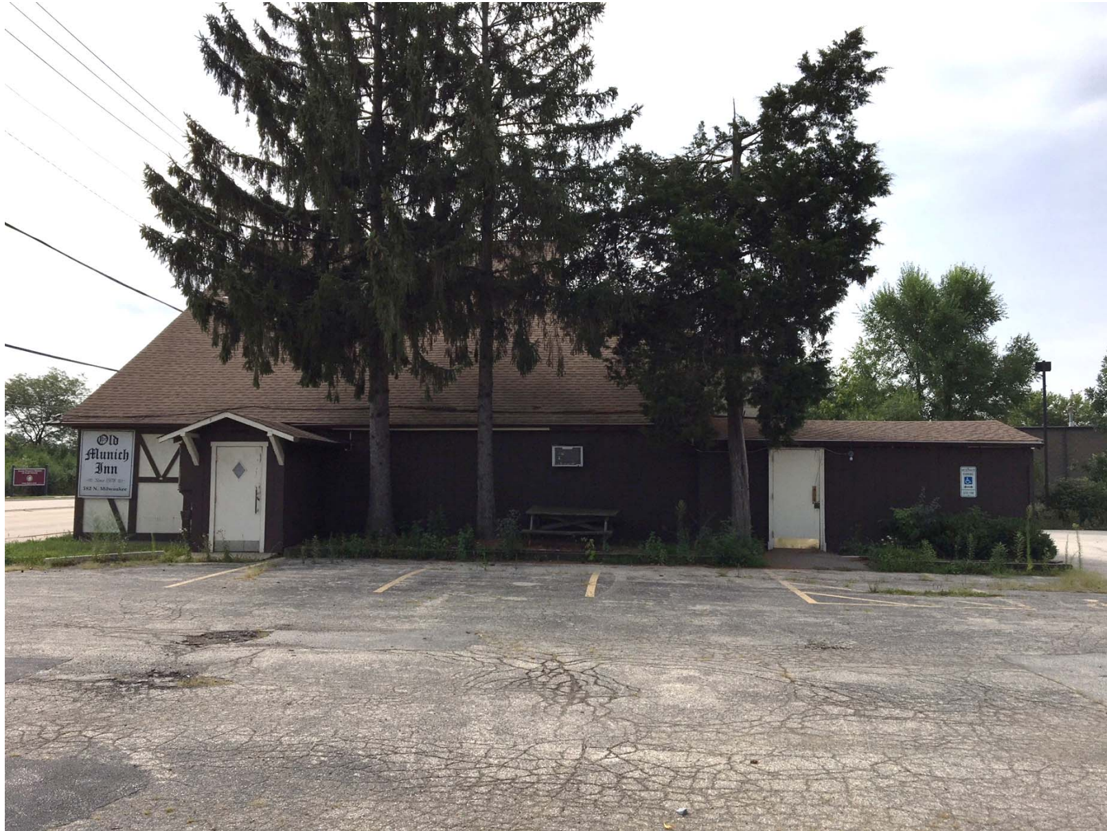
Existing conditions of north side (looking south)
