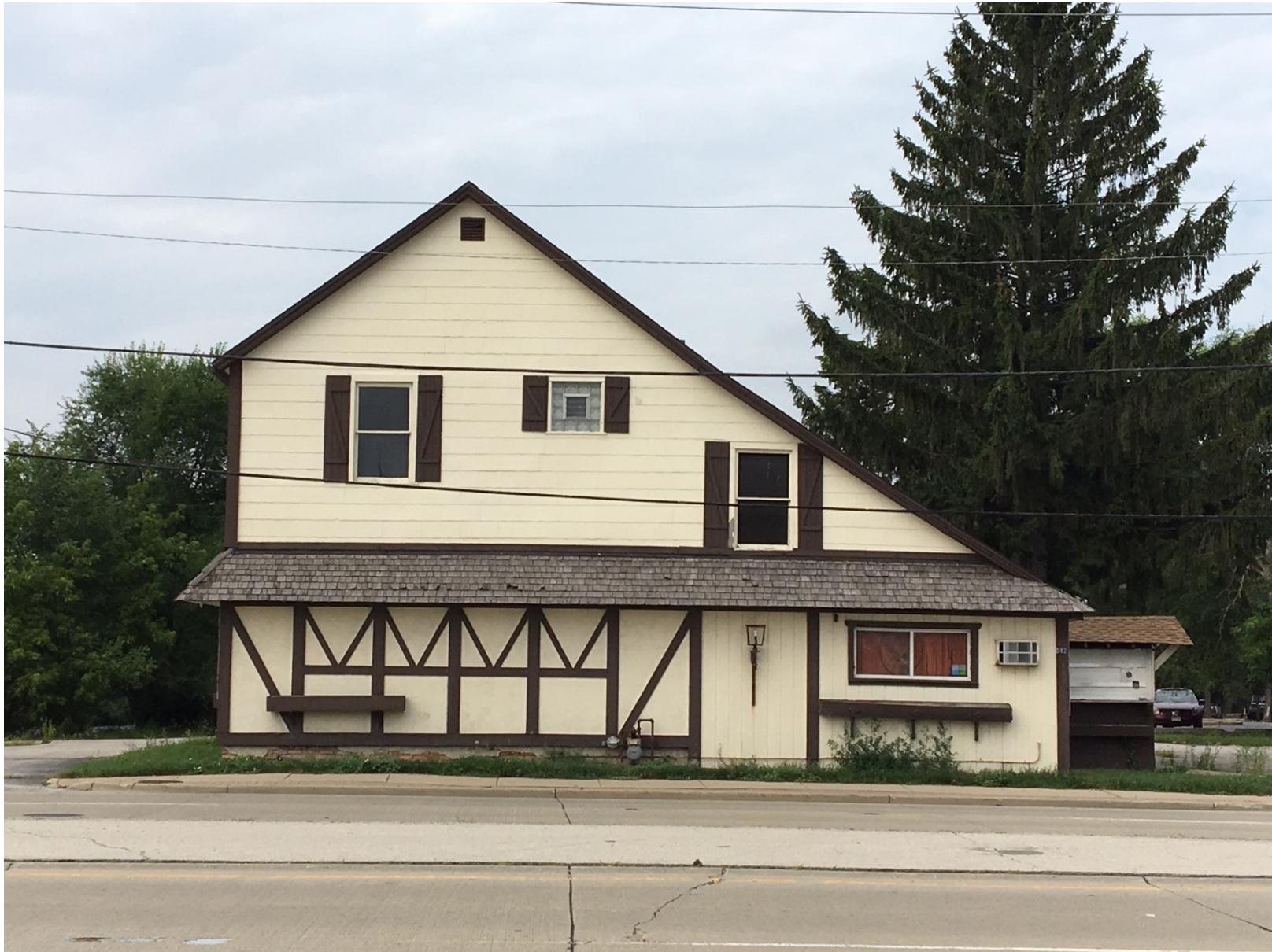
Existing conditions of front façade (looking west)
