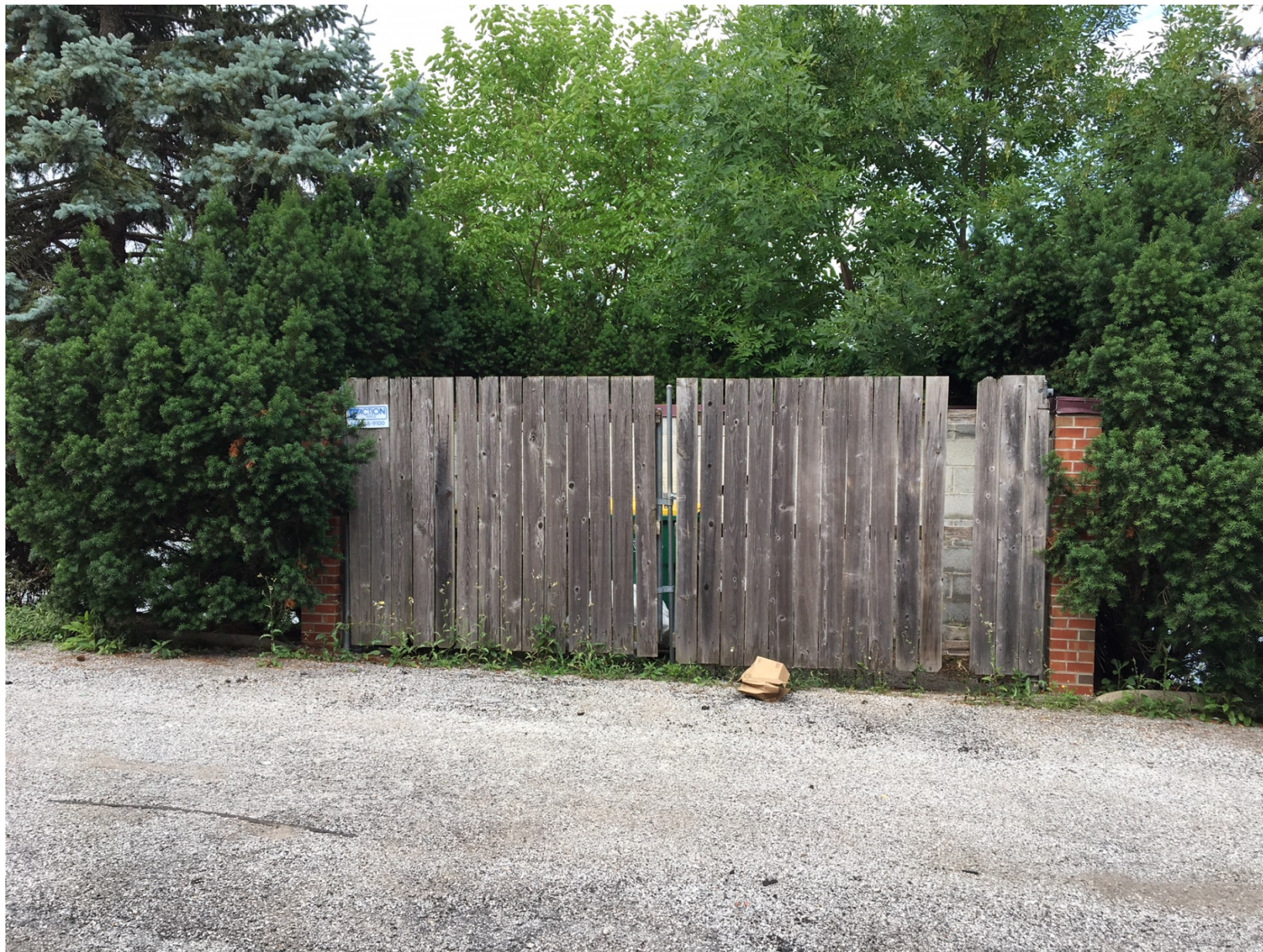
Existing conditions of trash enclosure in service alley behind subject unit (looking west)
