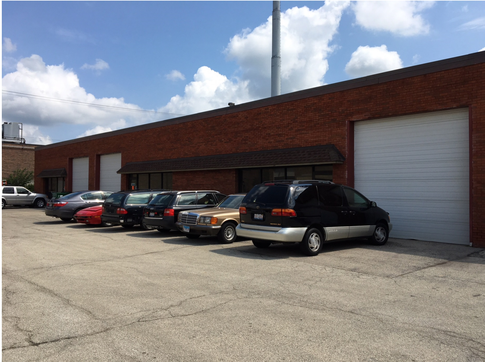
Existing conditions of west side of subject unit (looking northeast)
