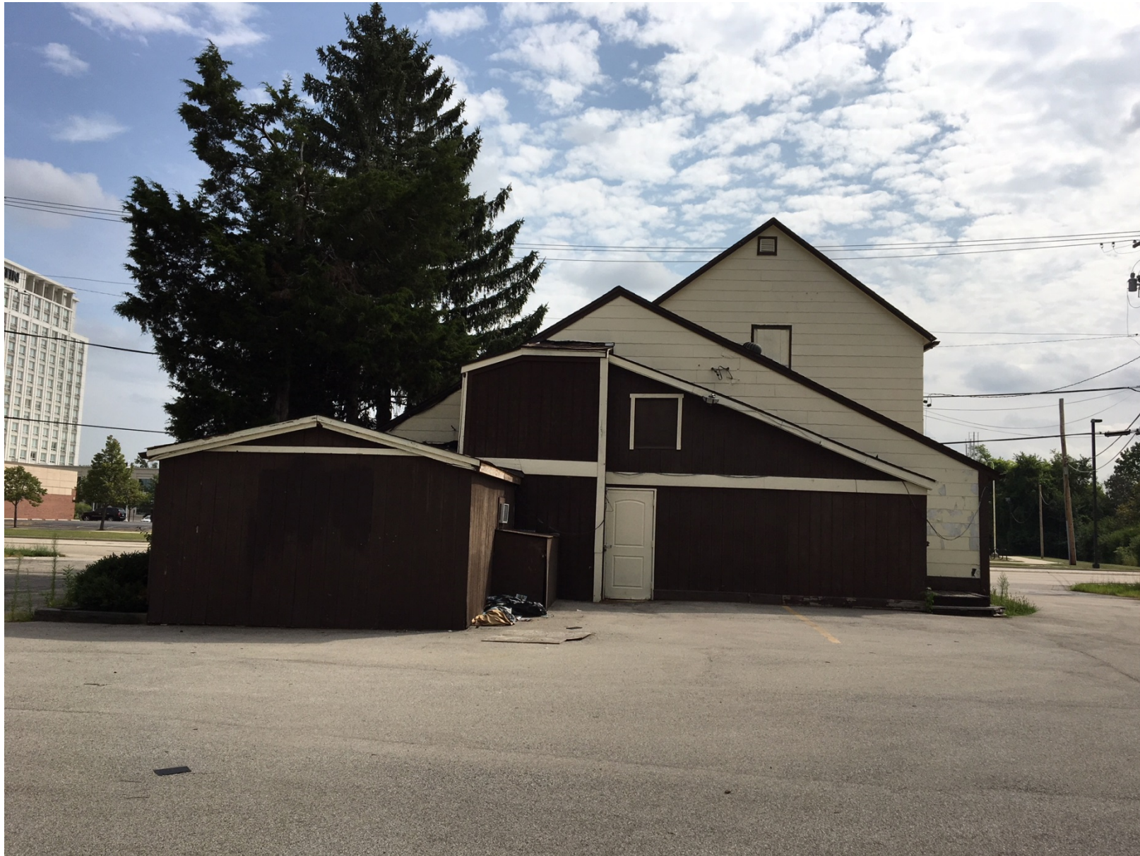
Existing conditions of rear façade (looking east)
