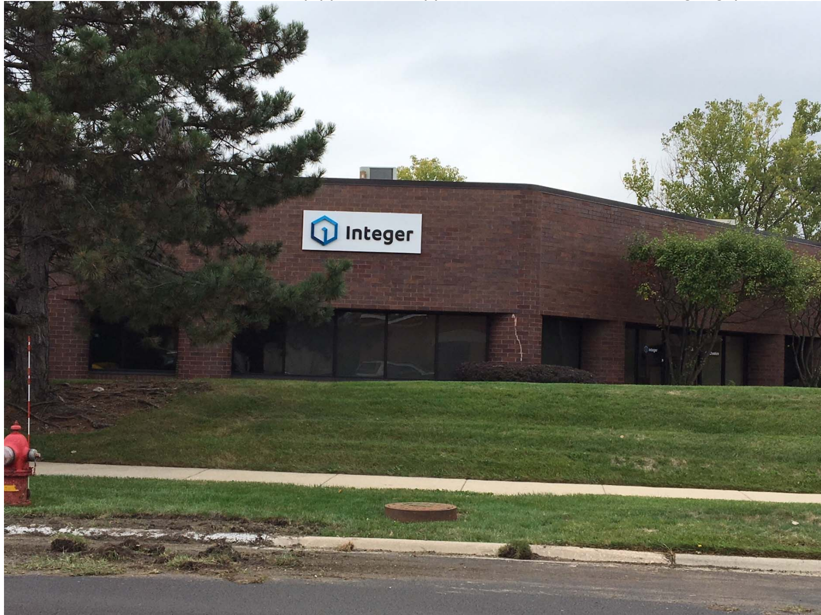
Existing conditions of façade along Chaddick Drive (looking west)
