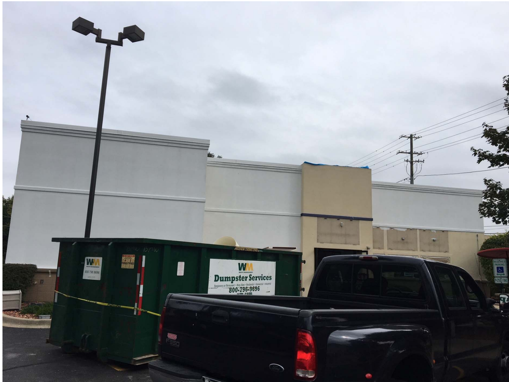
Existing conditions of side façade – looking east
