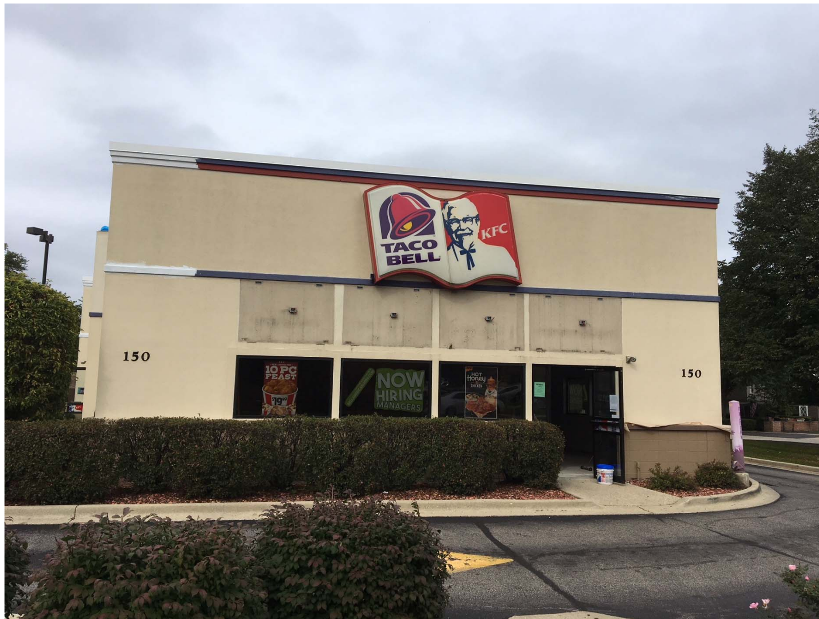
Existing conditions of front façade – looking north
