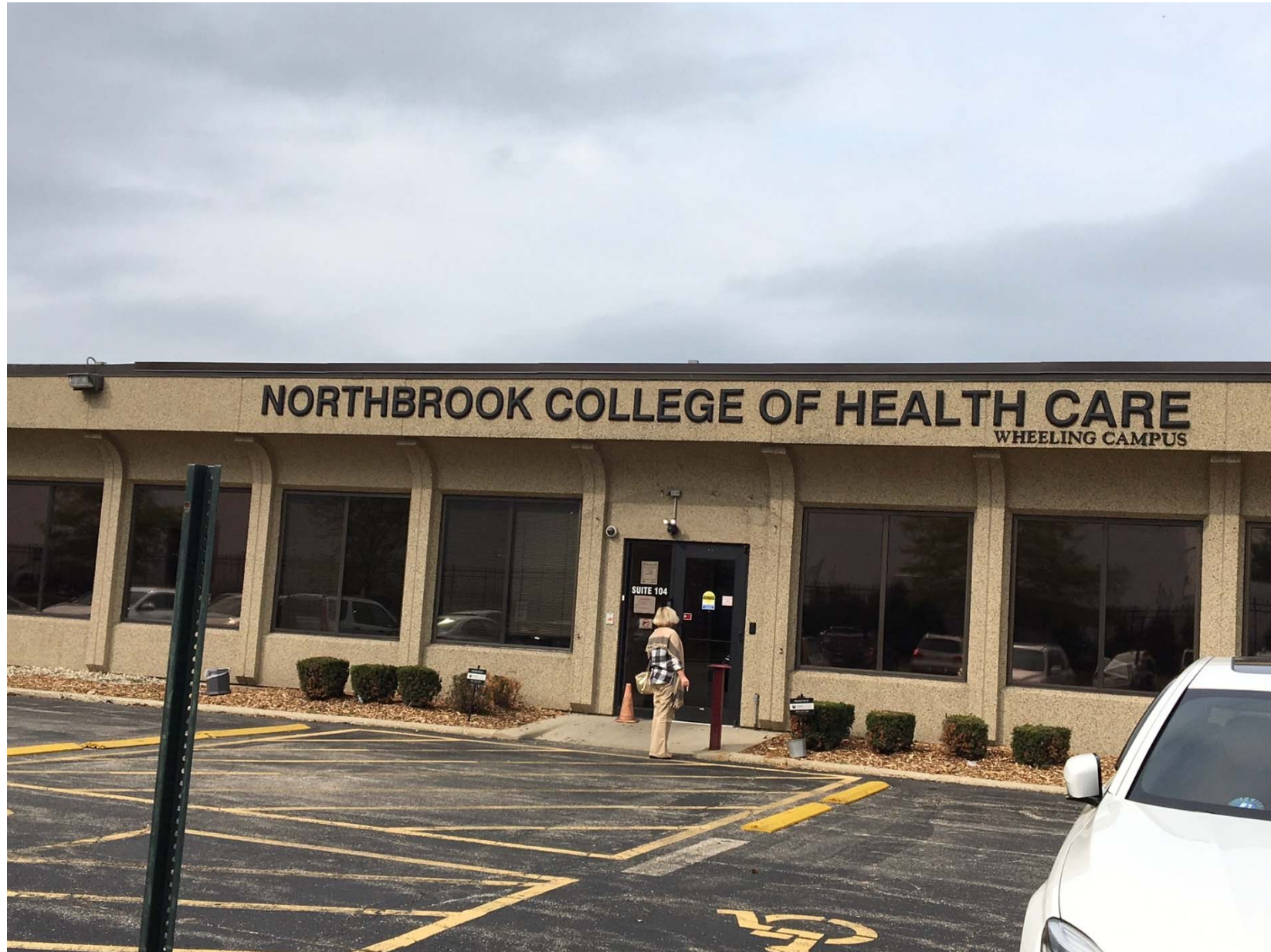
Existing conditions of subject unit (looking north)
