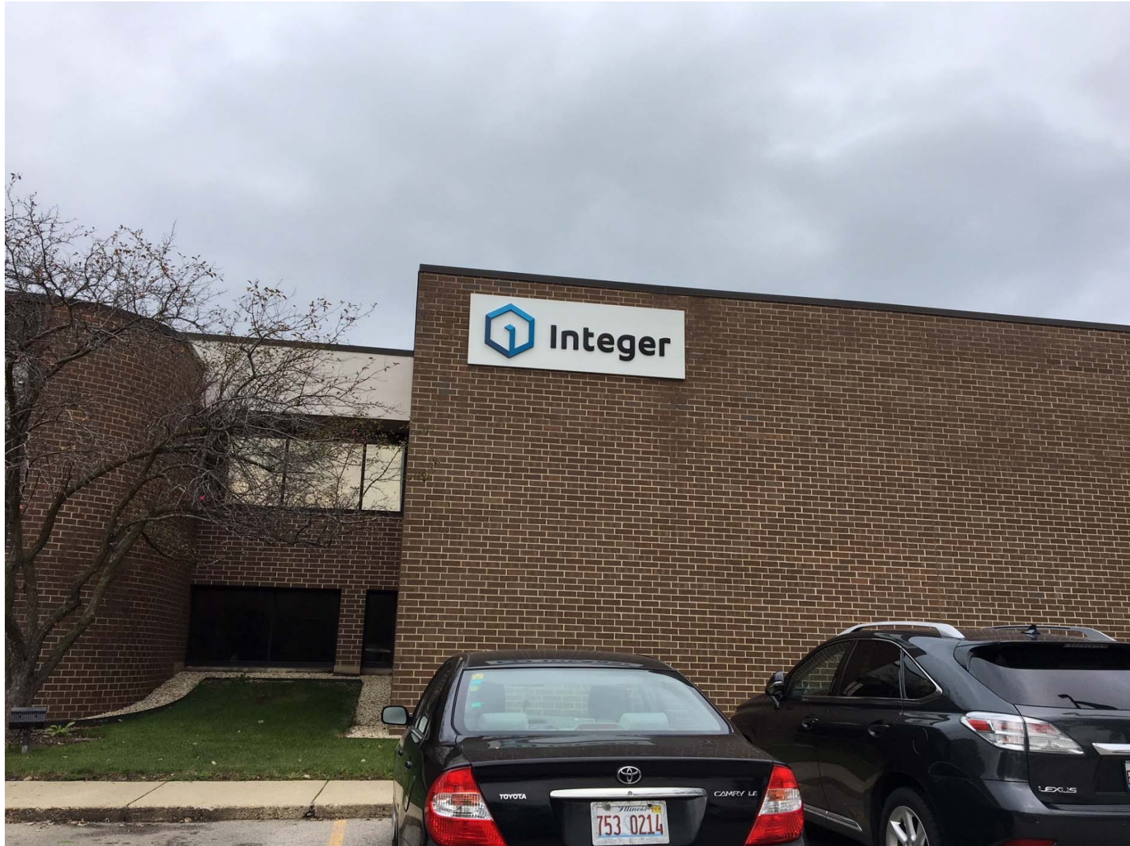
Existing conditions of façade along Hintz Road
