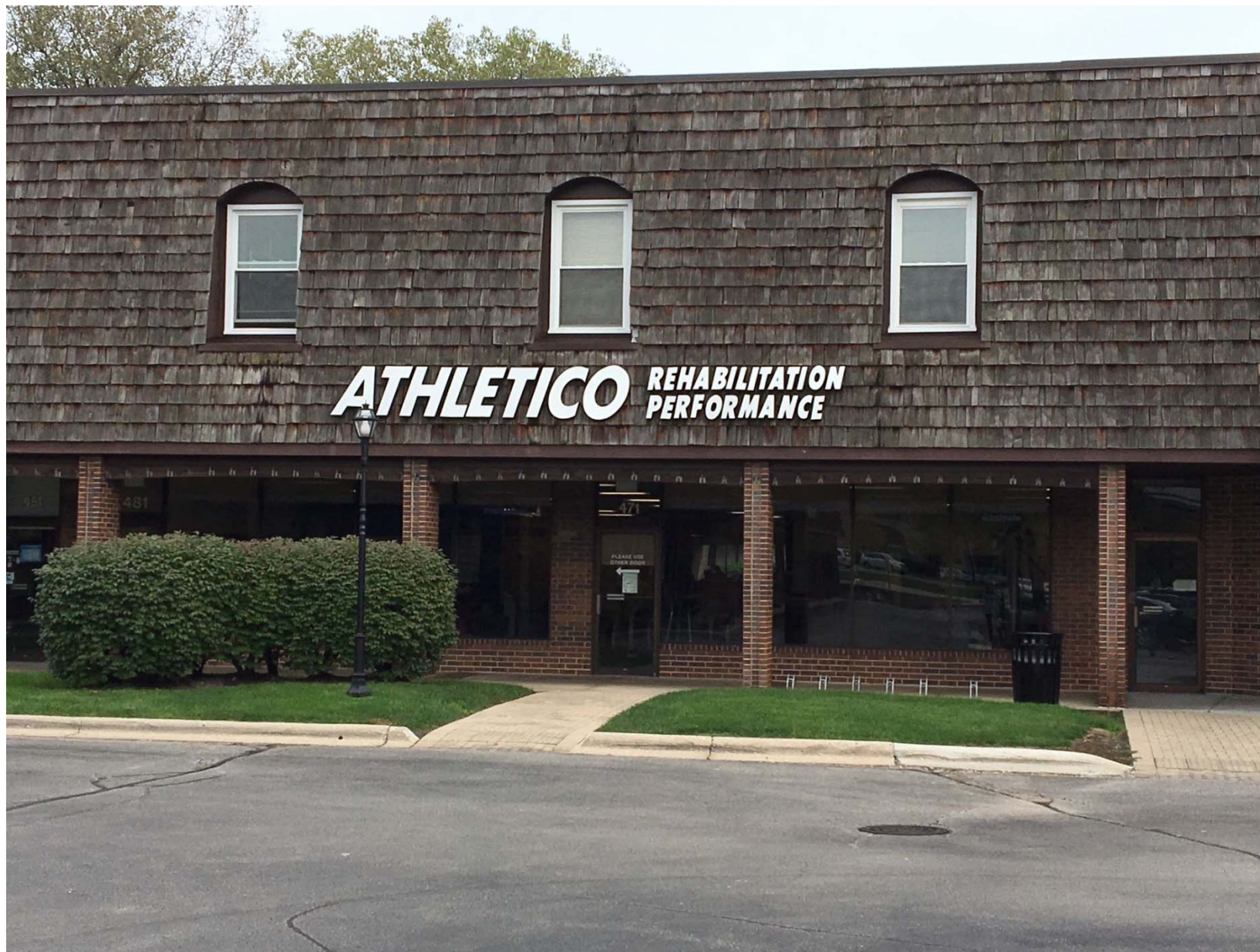
Existing conditions of subject unit (looking east)
