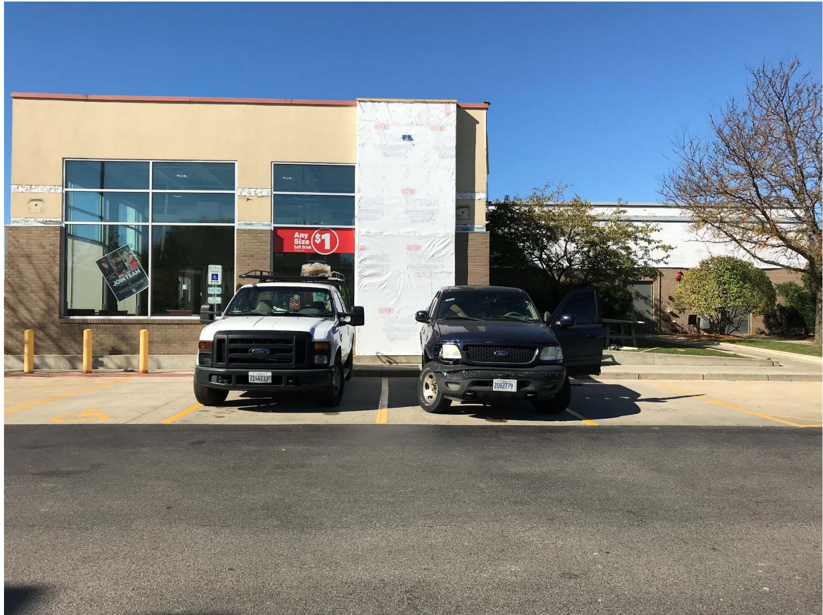
Existing conditions of property – looking west
