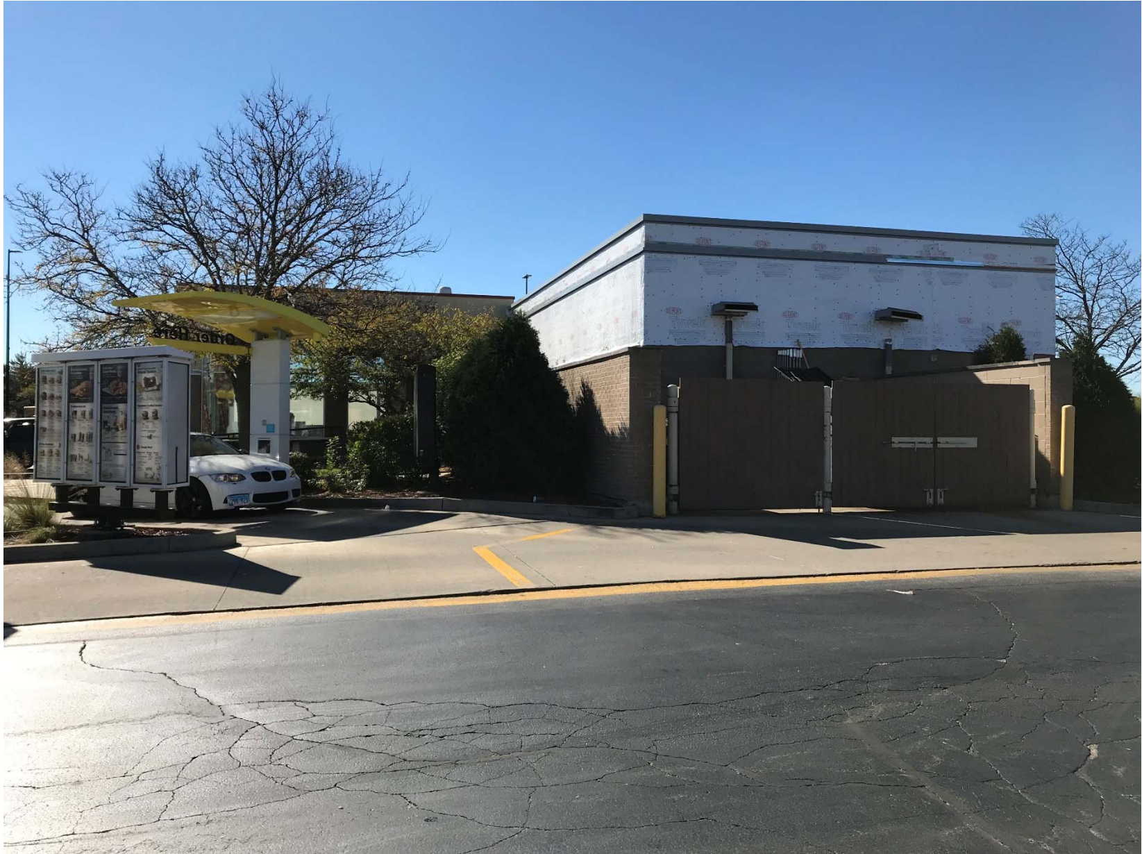
Existing conditions of property – looking south
