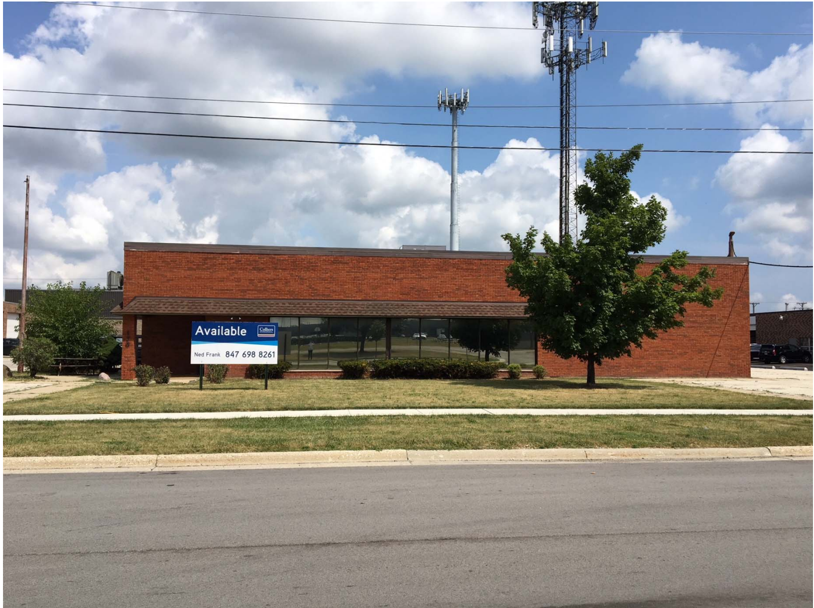
Existing conditions of property along Shepard Ave. (looking north)
