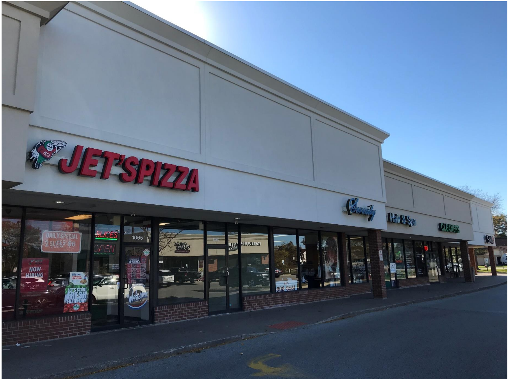
Existing conditions of subject unit (looking south)
