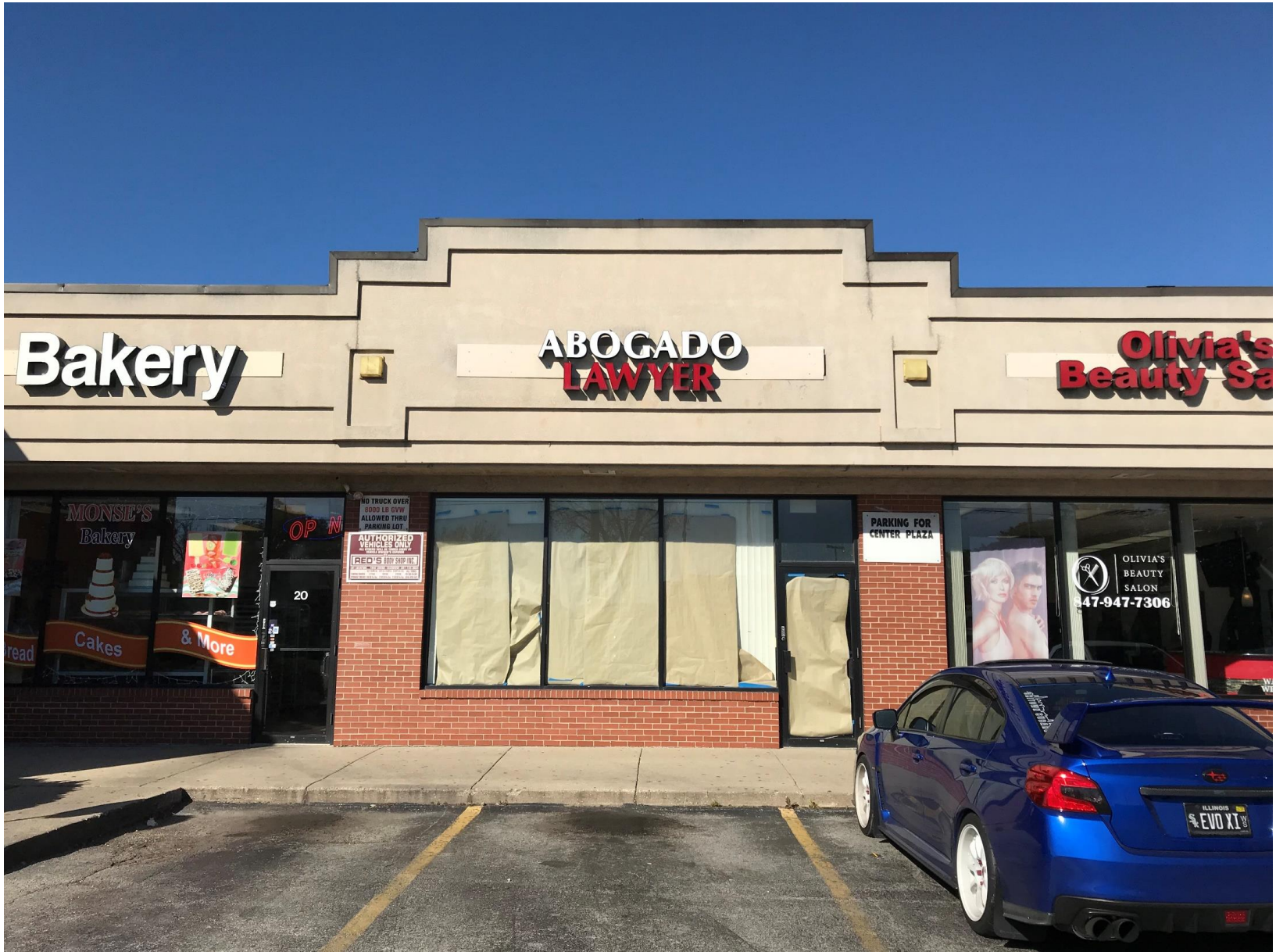
Existing conditions of subject unit (looking north)
