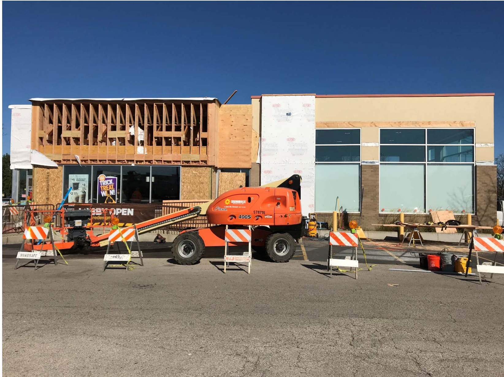
Existing conditions of property – looking north
