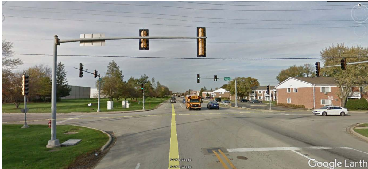
PHOTO 1: S. WOLF ROAD AT OLD WILLOW ROAD
