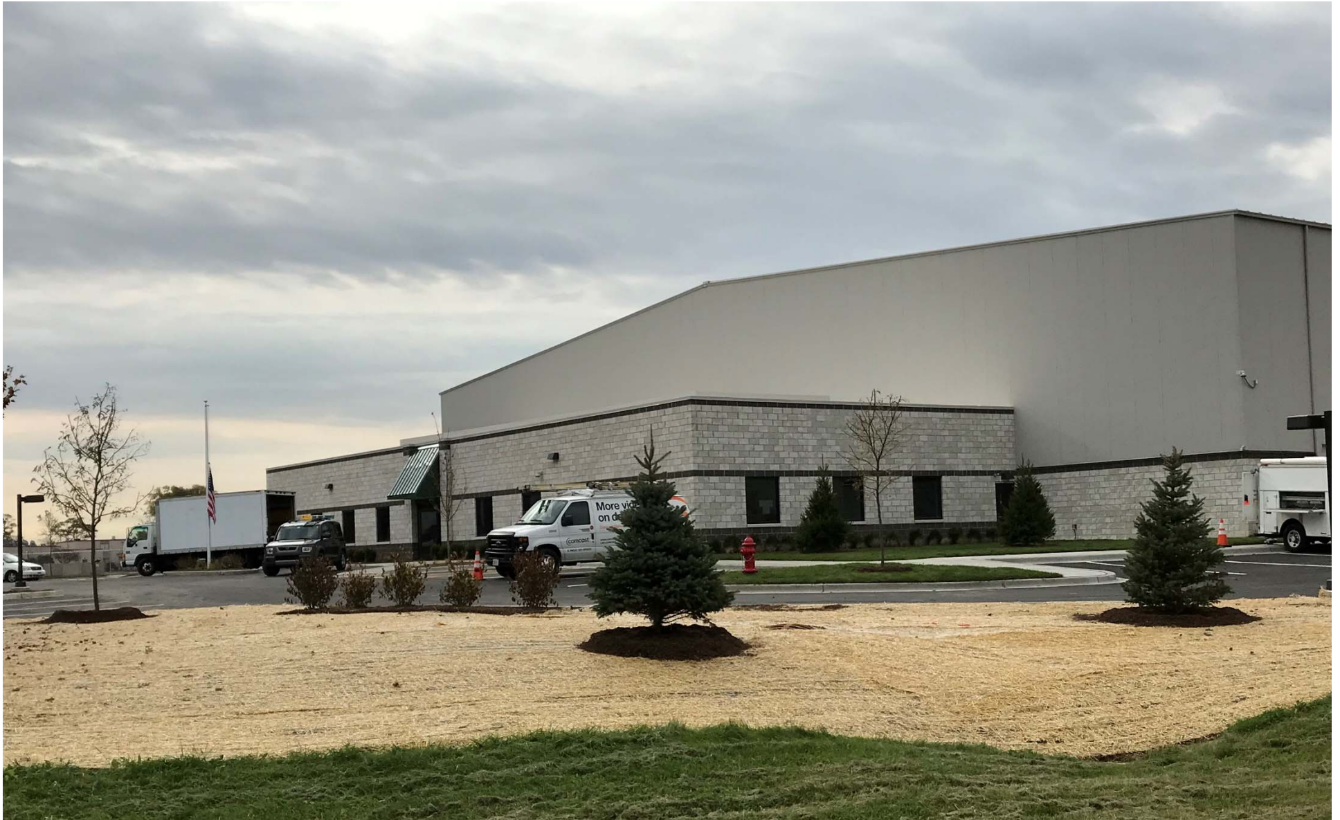
Existing conditions of east (front) building facade
