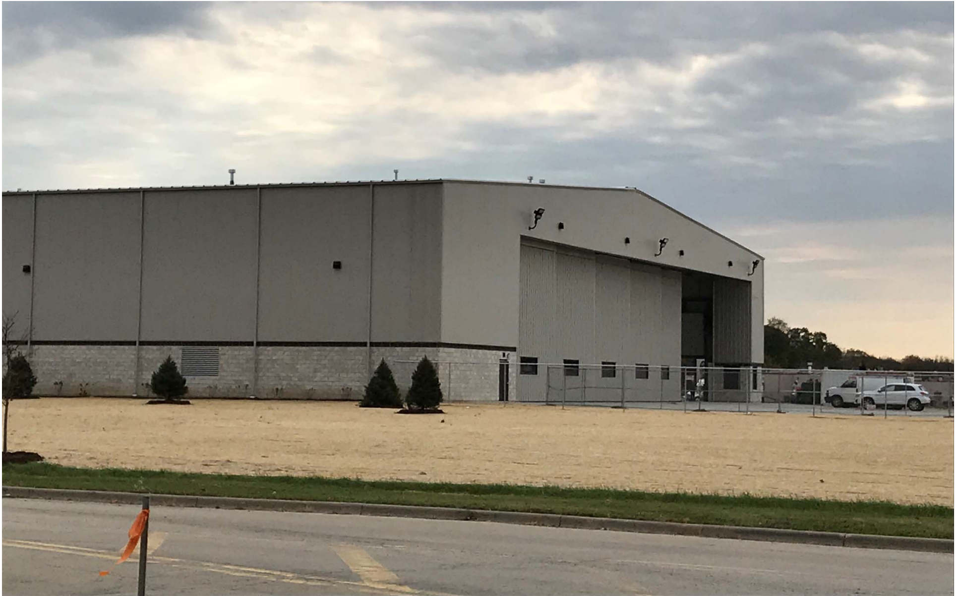
Existing conditions of west (airport side) building facade
