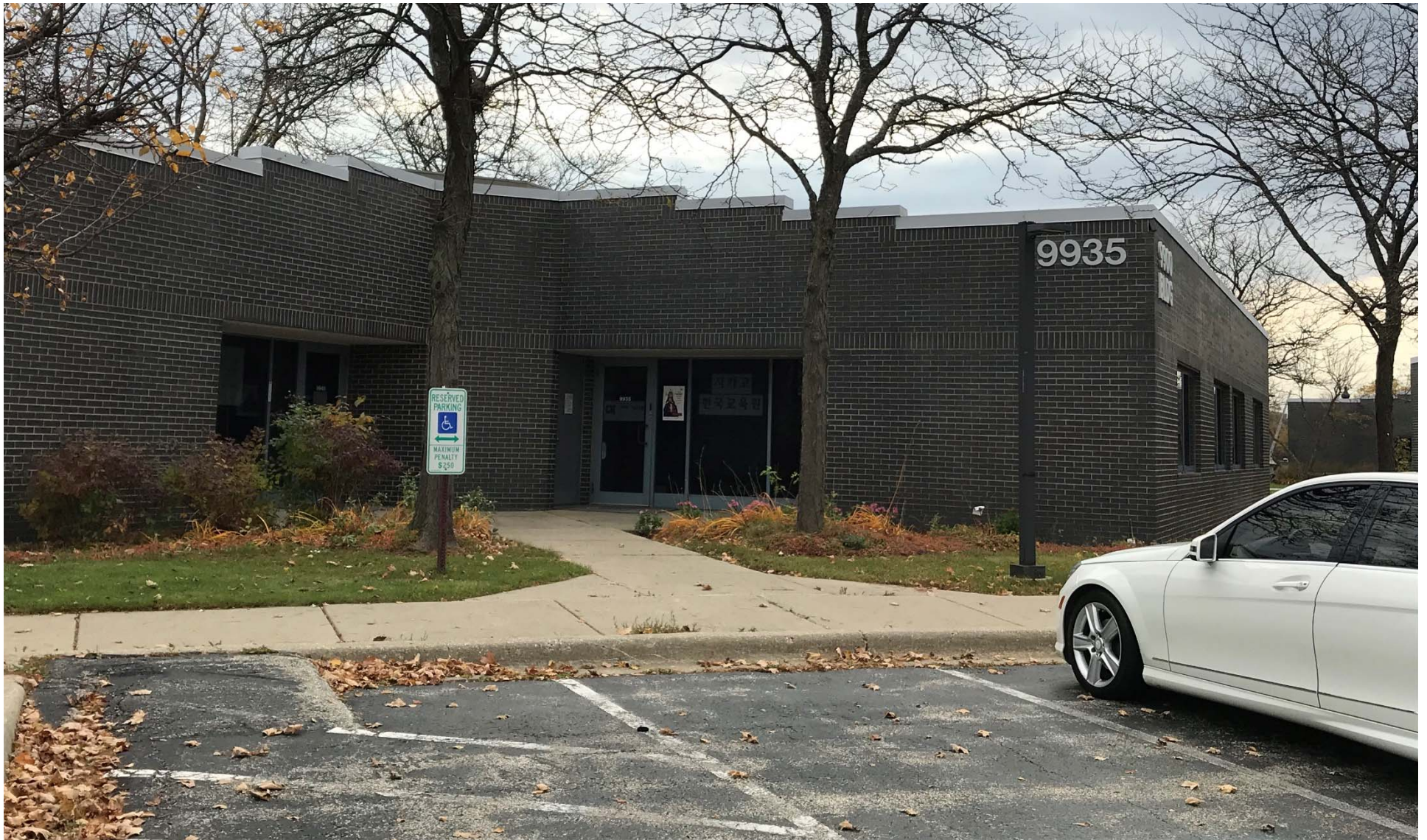
Existing conditions of north (front) building facade
