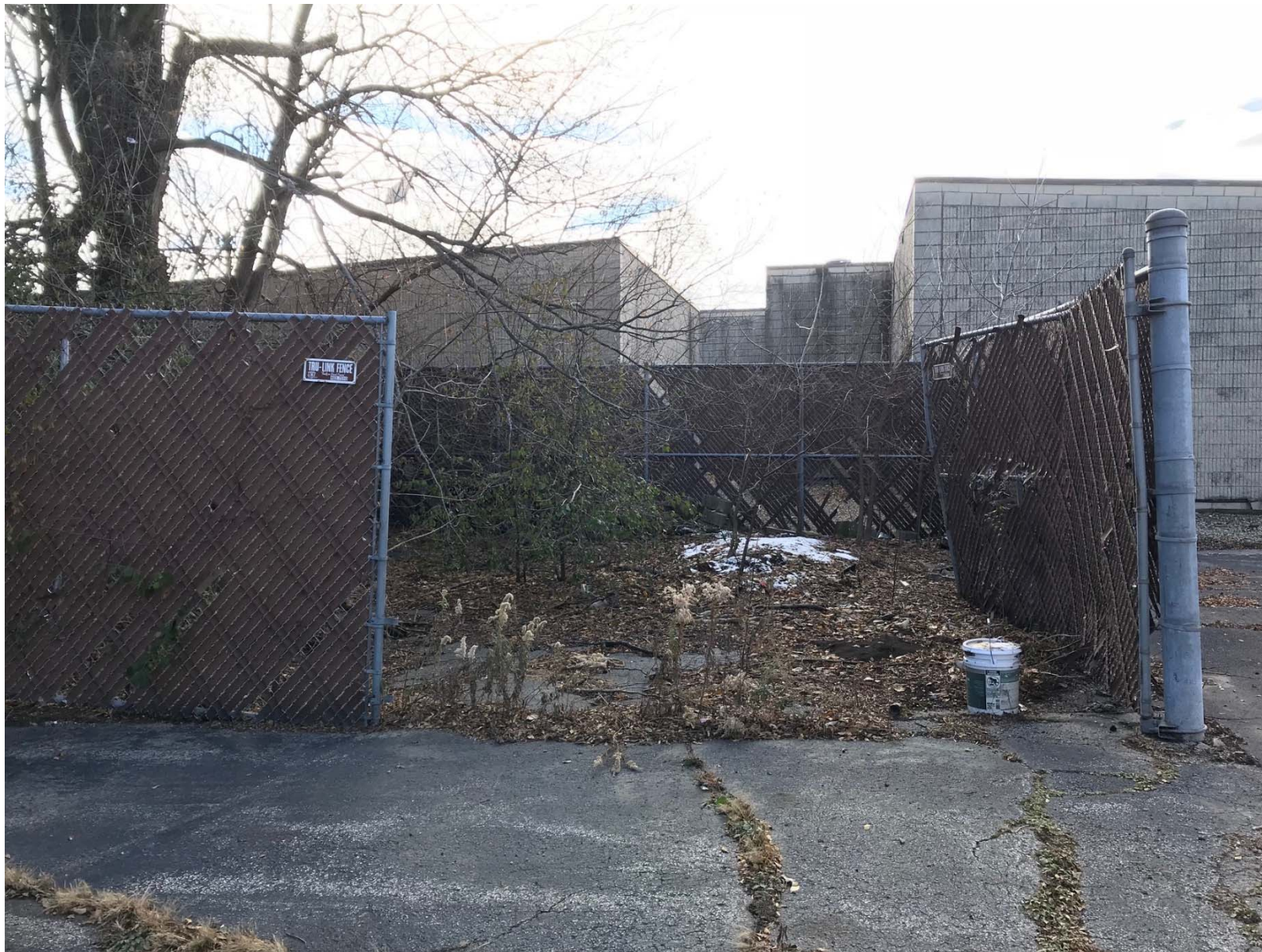
Existing conditions of trash enclosure – looking south
