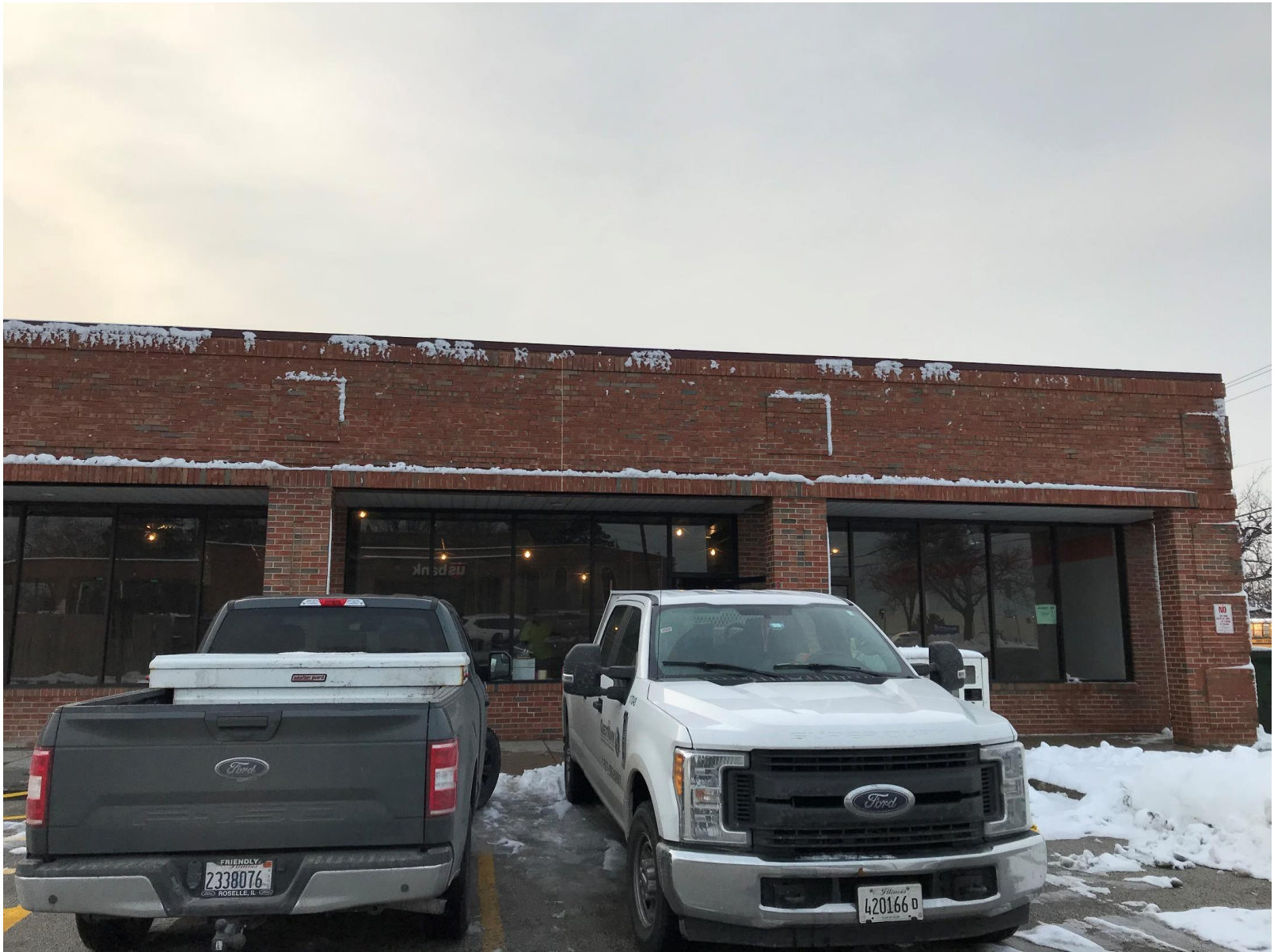
Existing conditions of subject unit (looking west)
