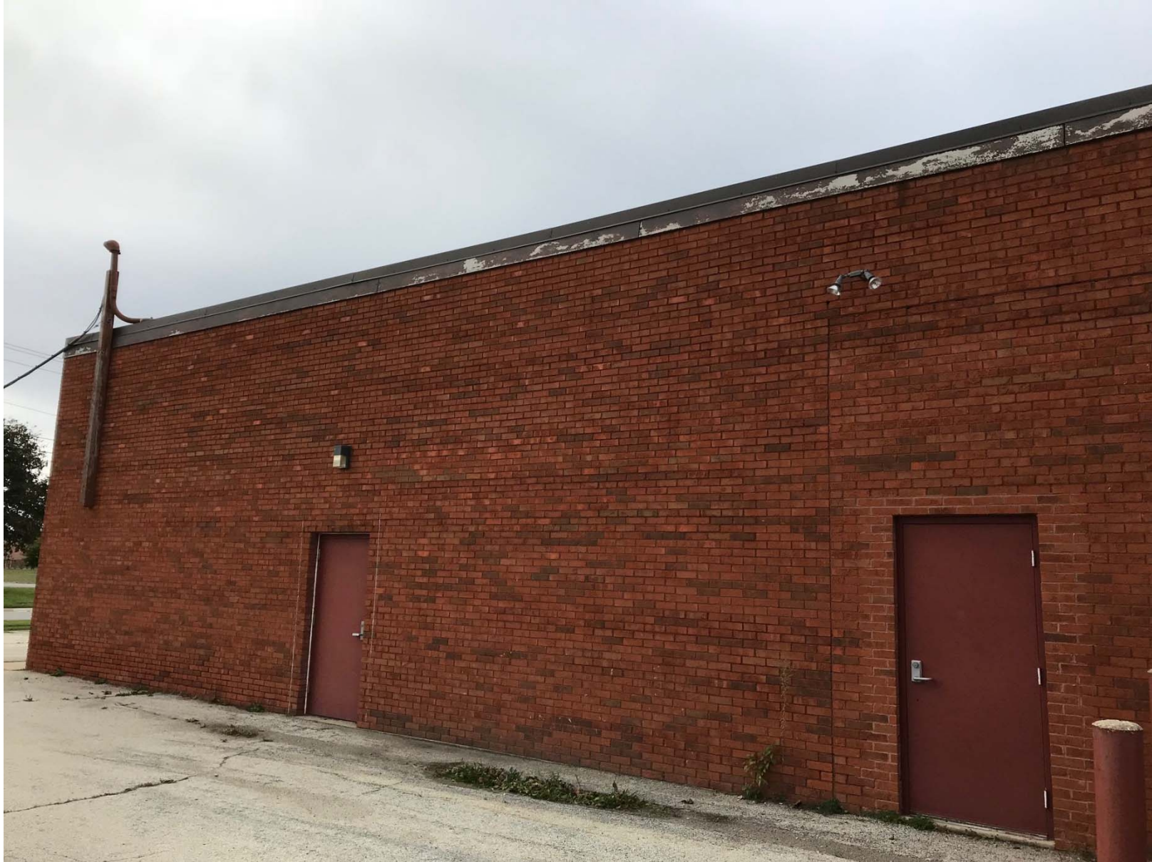
Existing conditions of east side of subject unit (looking southwest)
