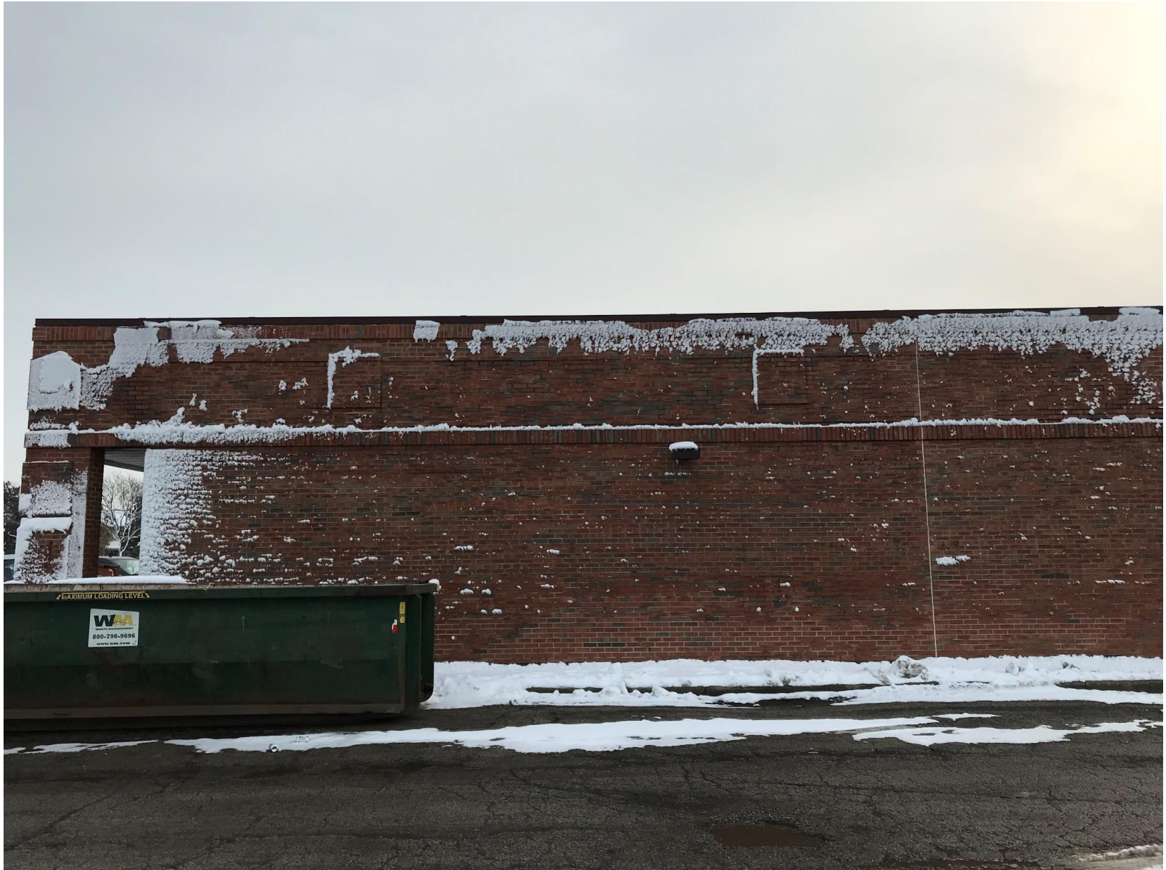
Existing conditions of subject unit (looking south)
