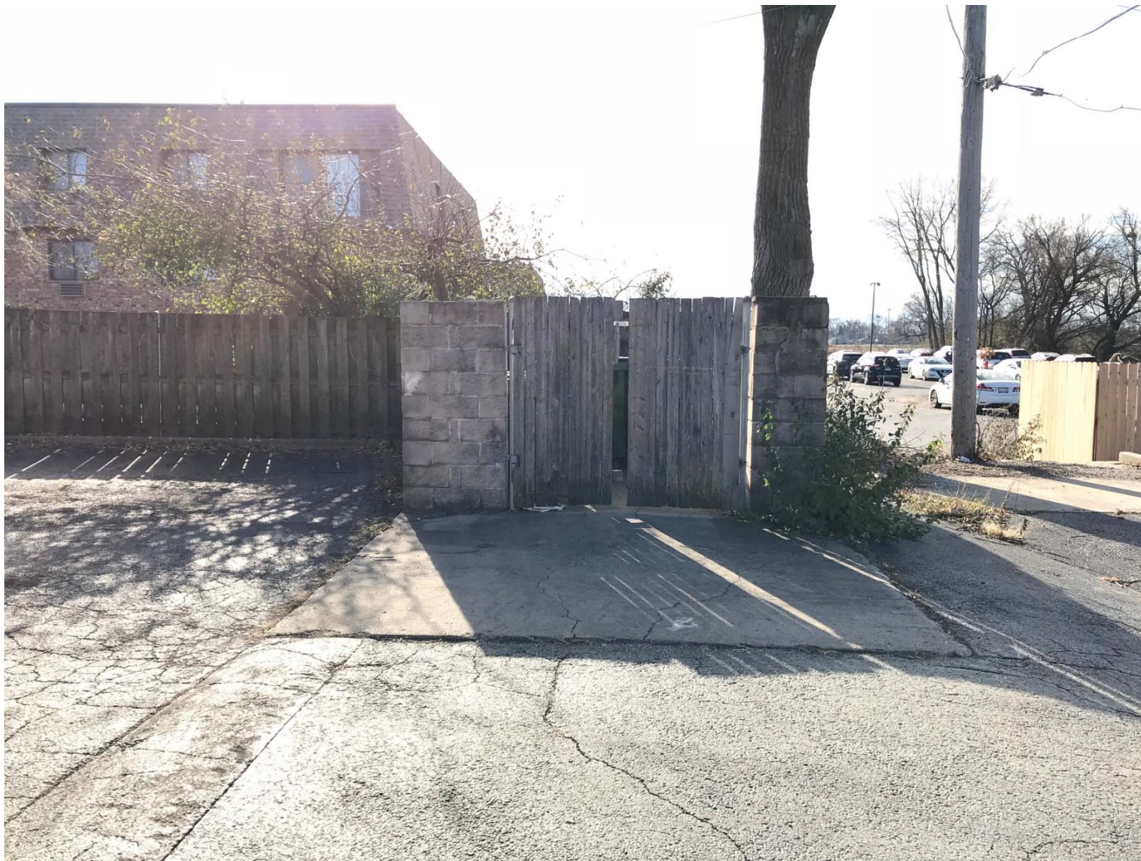
Existing conditions of trash enclosure (looking south)
