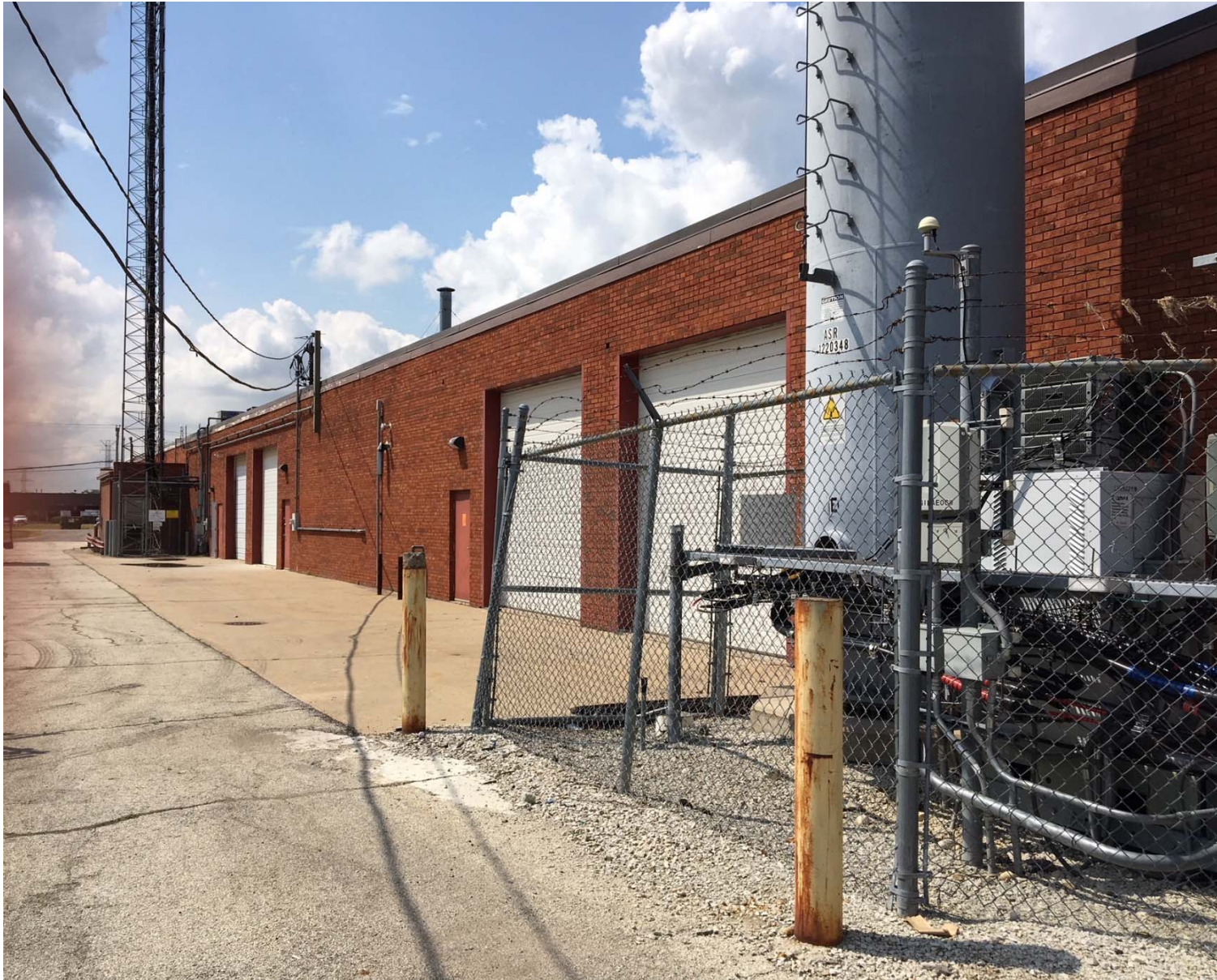
Existing conditions of east side of subject unit (looking southwest)
