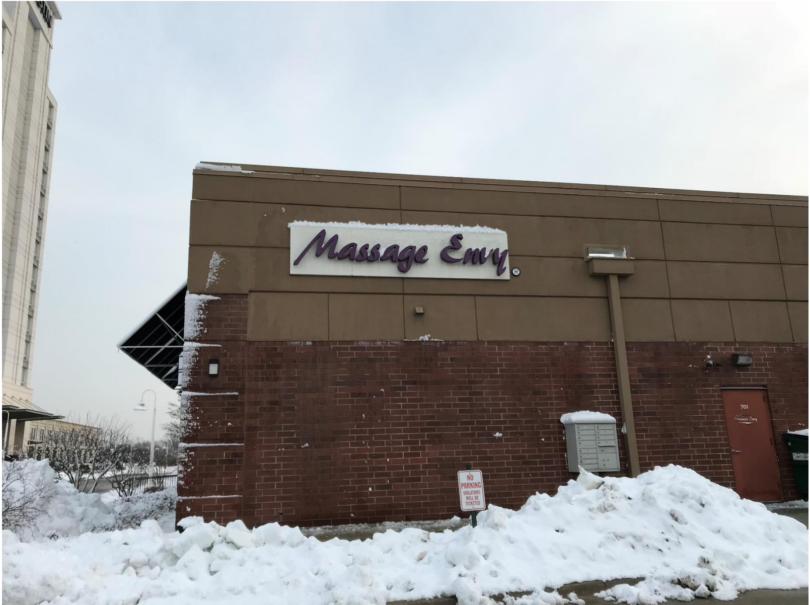
Existing conditions of subject unit (looking south)
