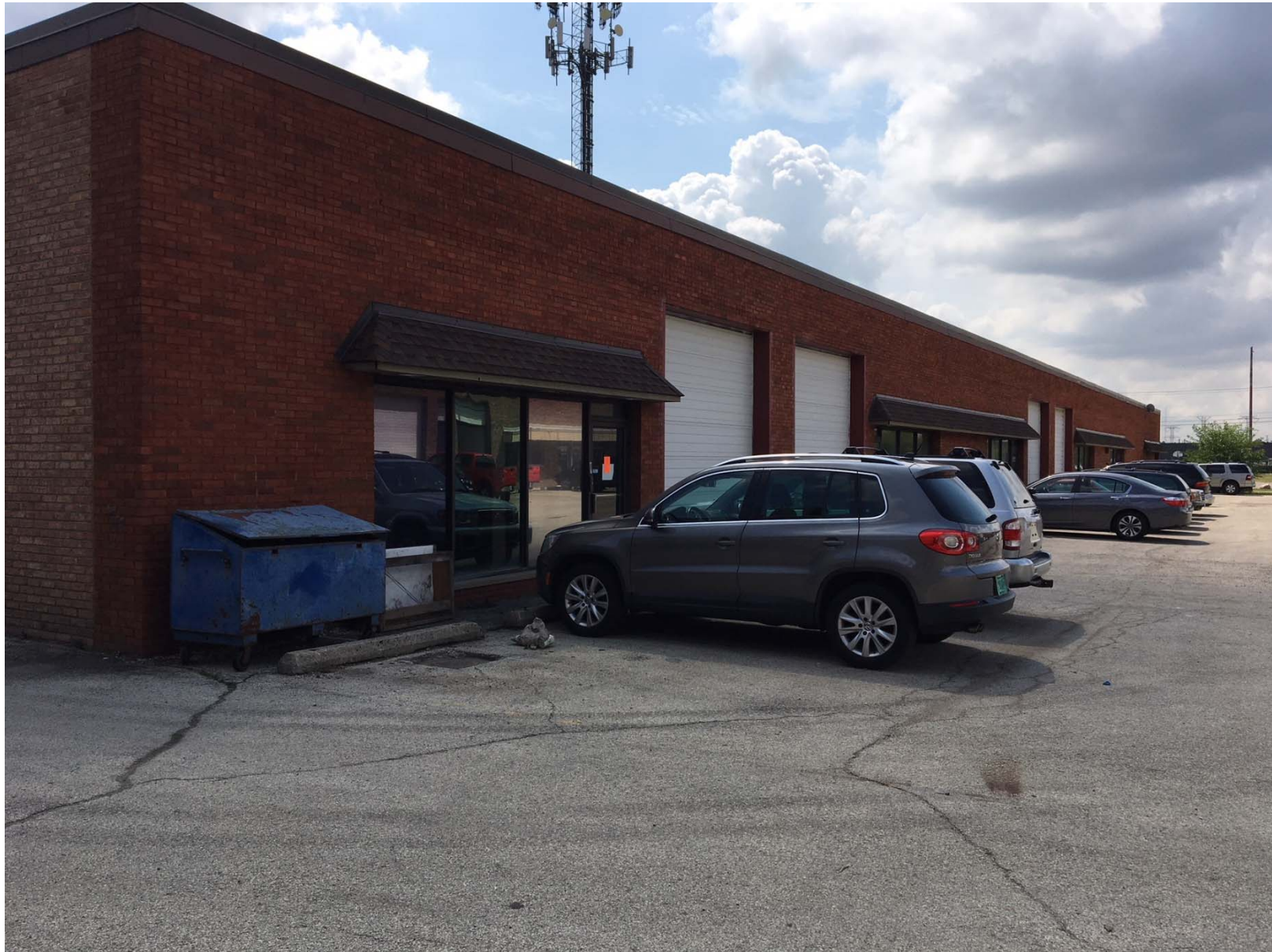
Existing conditions of west side of subject unit (looking southeast)
