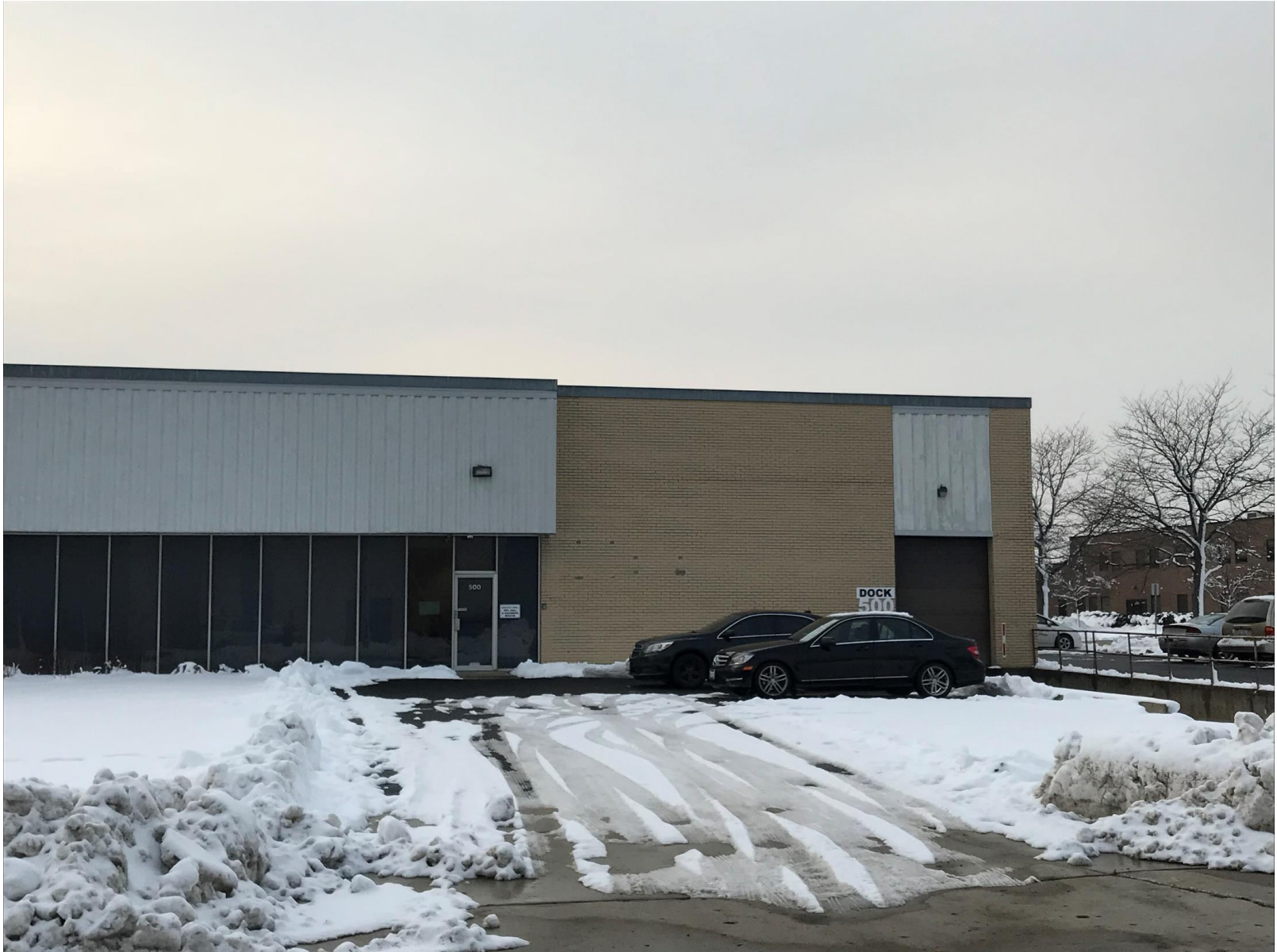
Existing conditions of subject unit (looking west)
