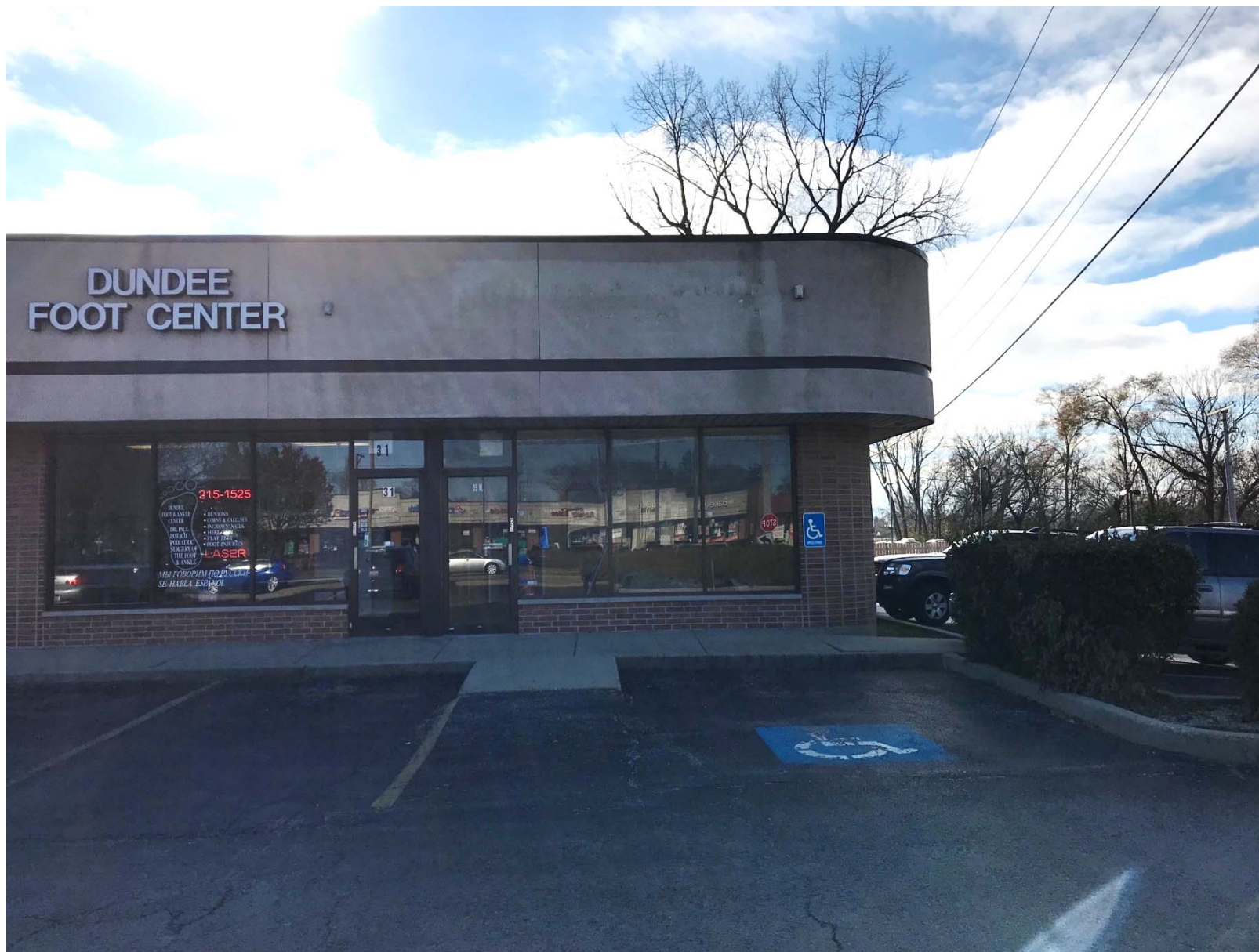
Existing conditions of subject unit (looking south)
