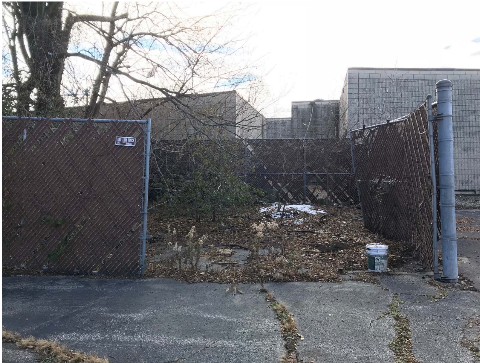
Existing conditions of trash enclosure – looking south
