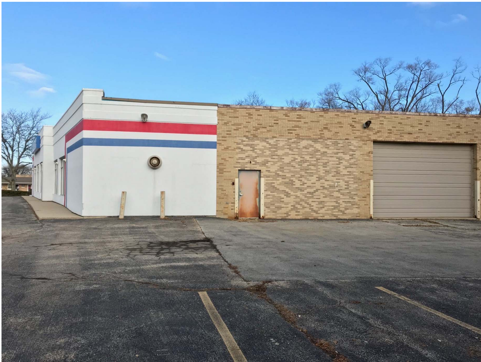
Existing conditions of subject property – north elevation
