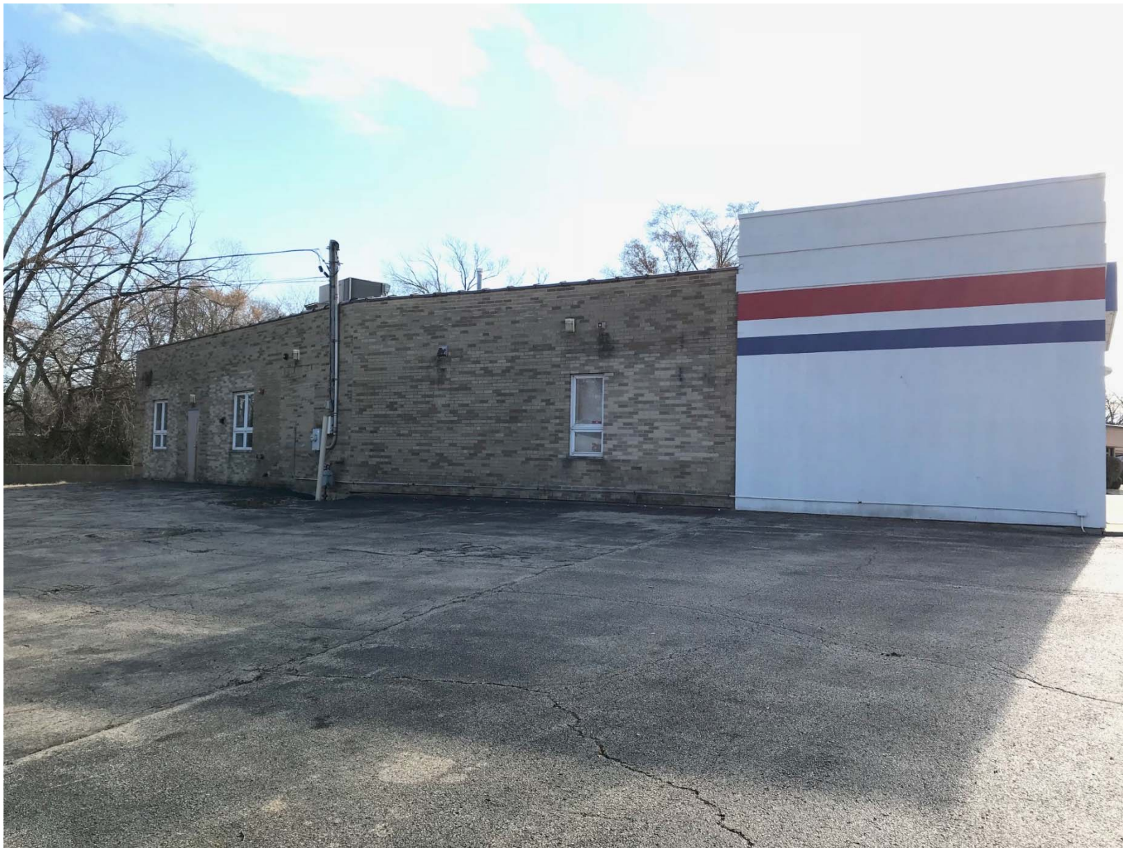
Existing conditions of subject property – north elevation
