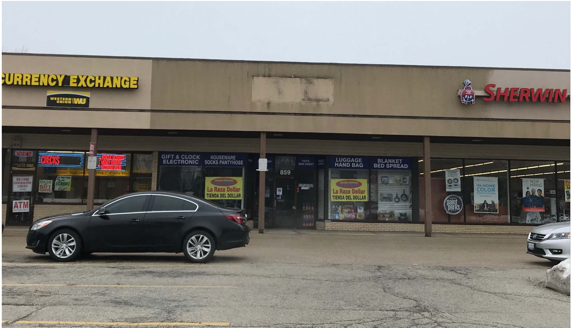
Existing conditions of storefront – looking south
