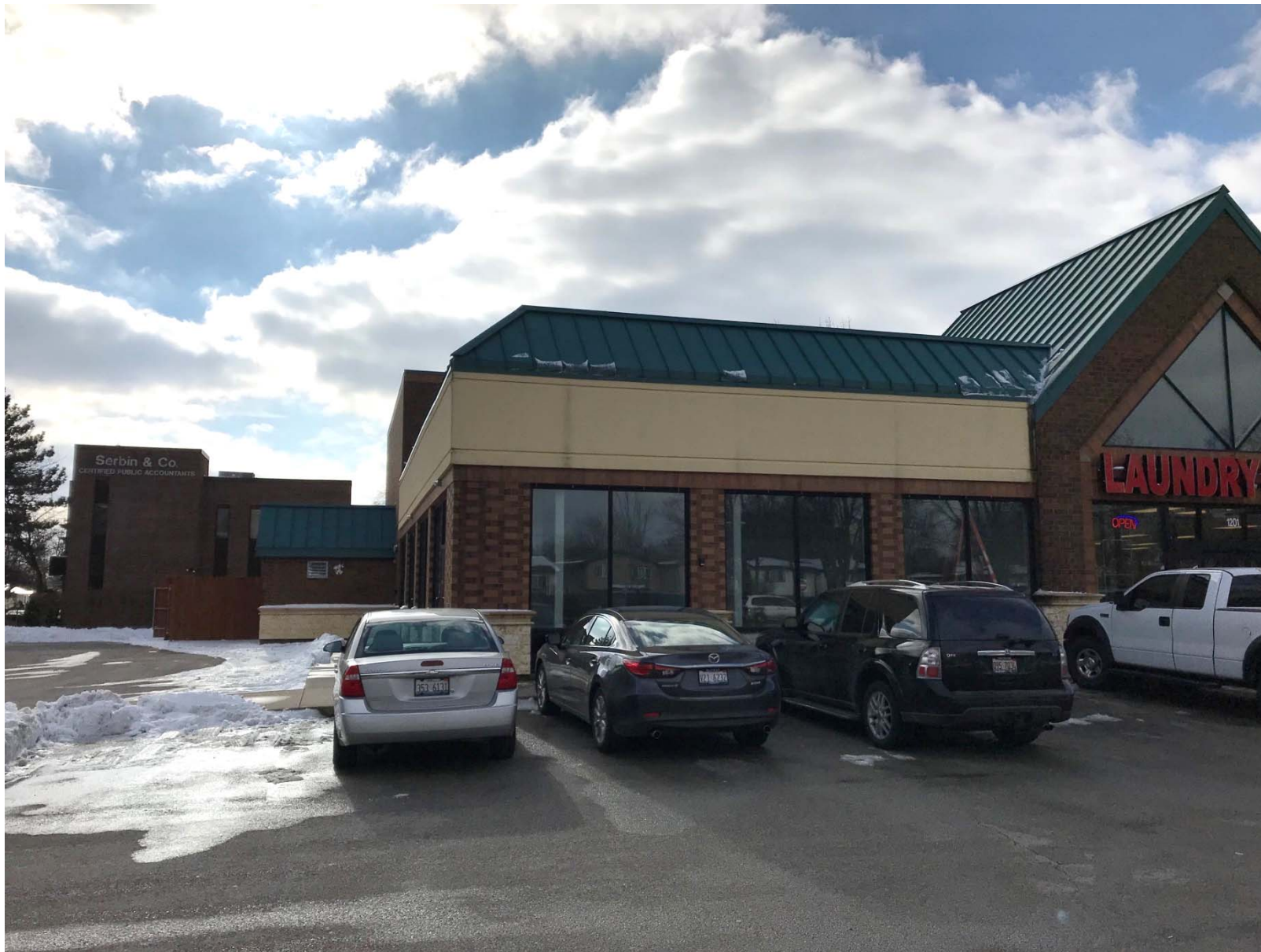
Existing conditions of storefront – looking south
