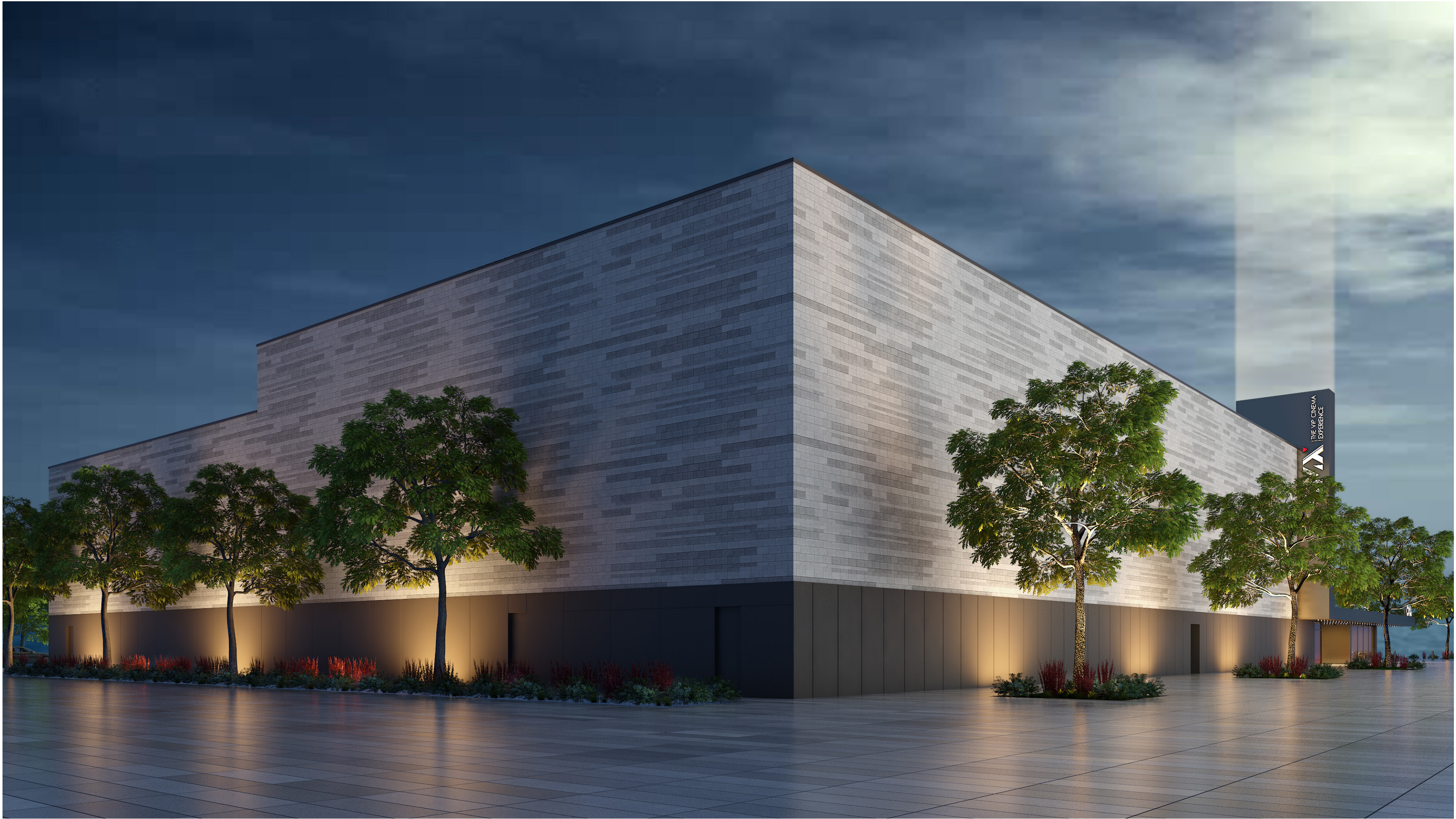
South East Corner View from Apartment Building
