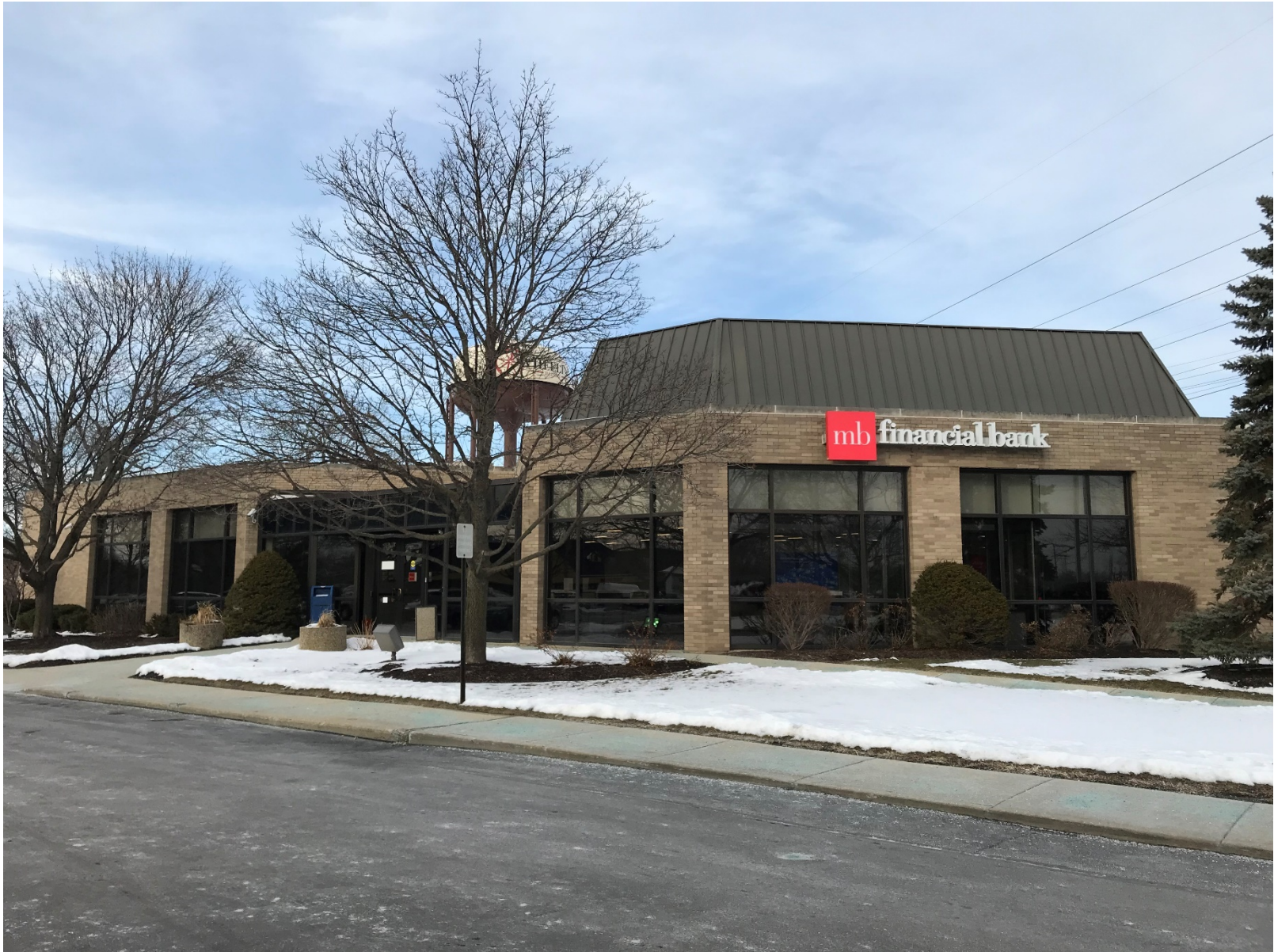
Existing conditions of subject property (looking northeast)
