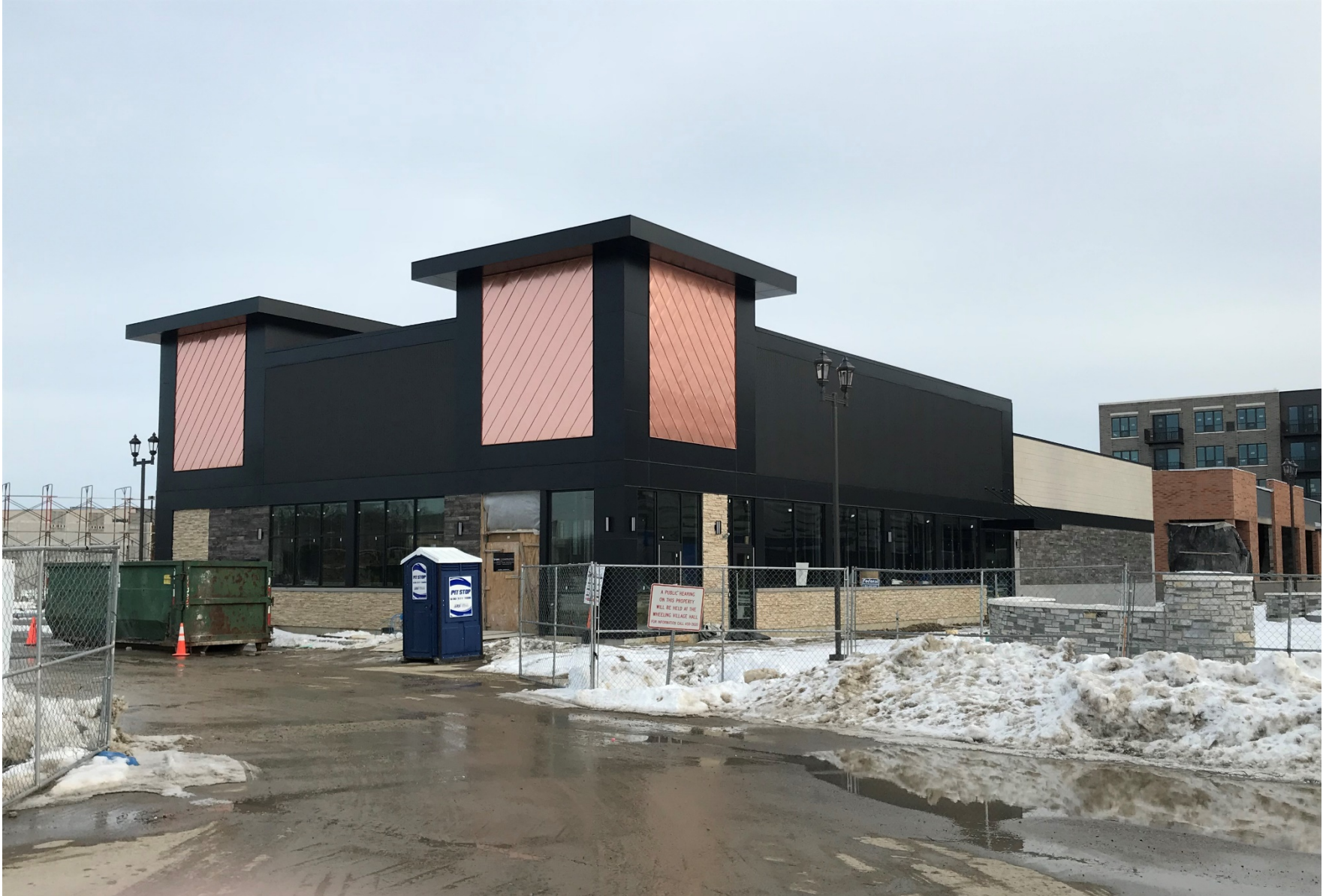
Existing conditions of subject building (looking south)
