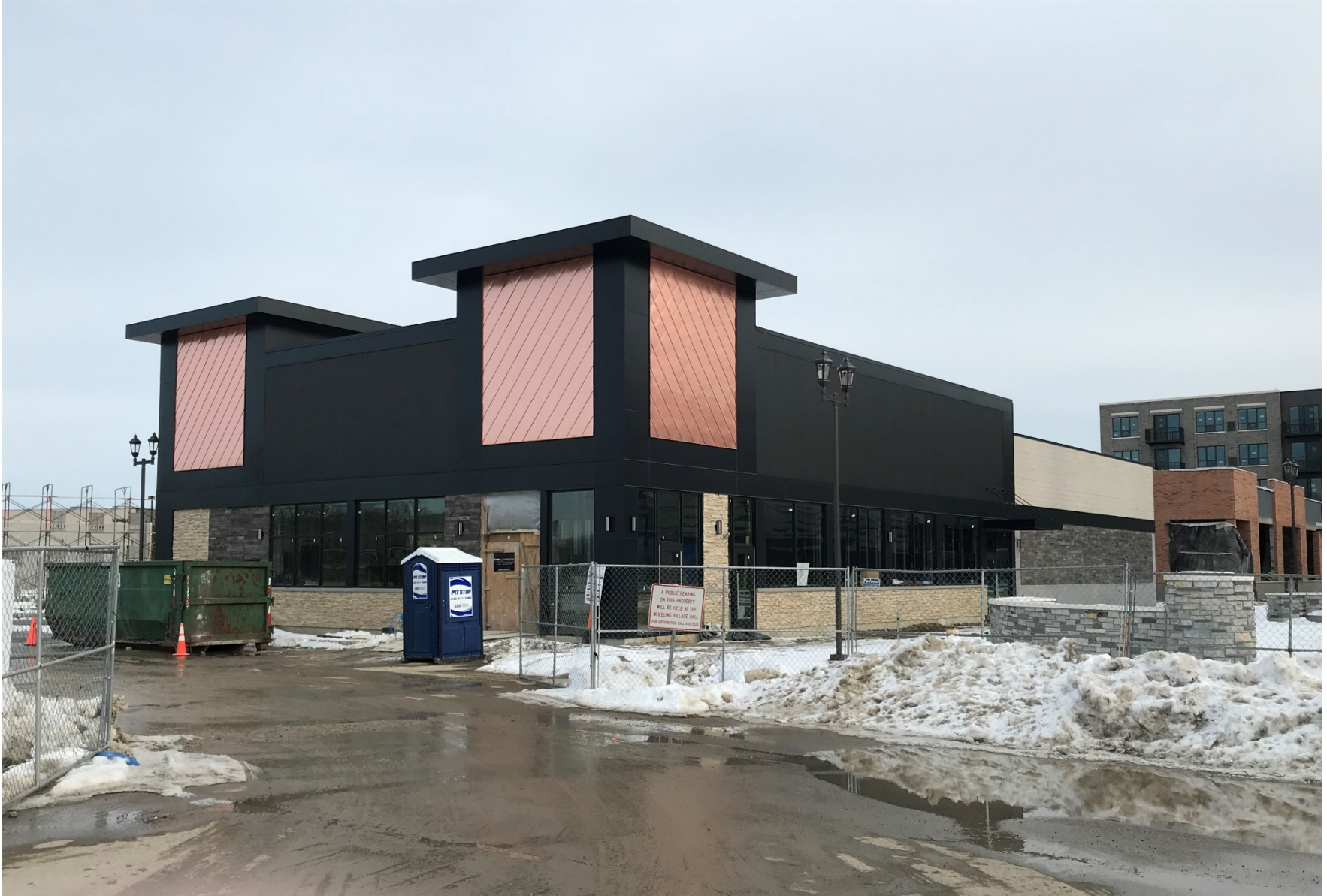
Existing conditions of subject building (looking south)
