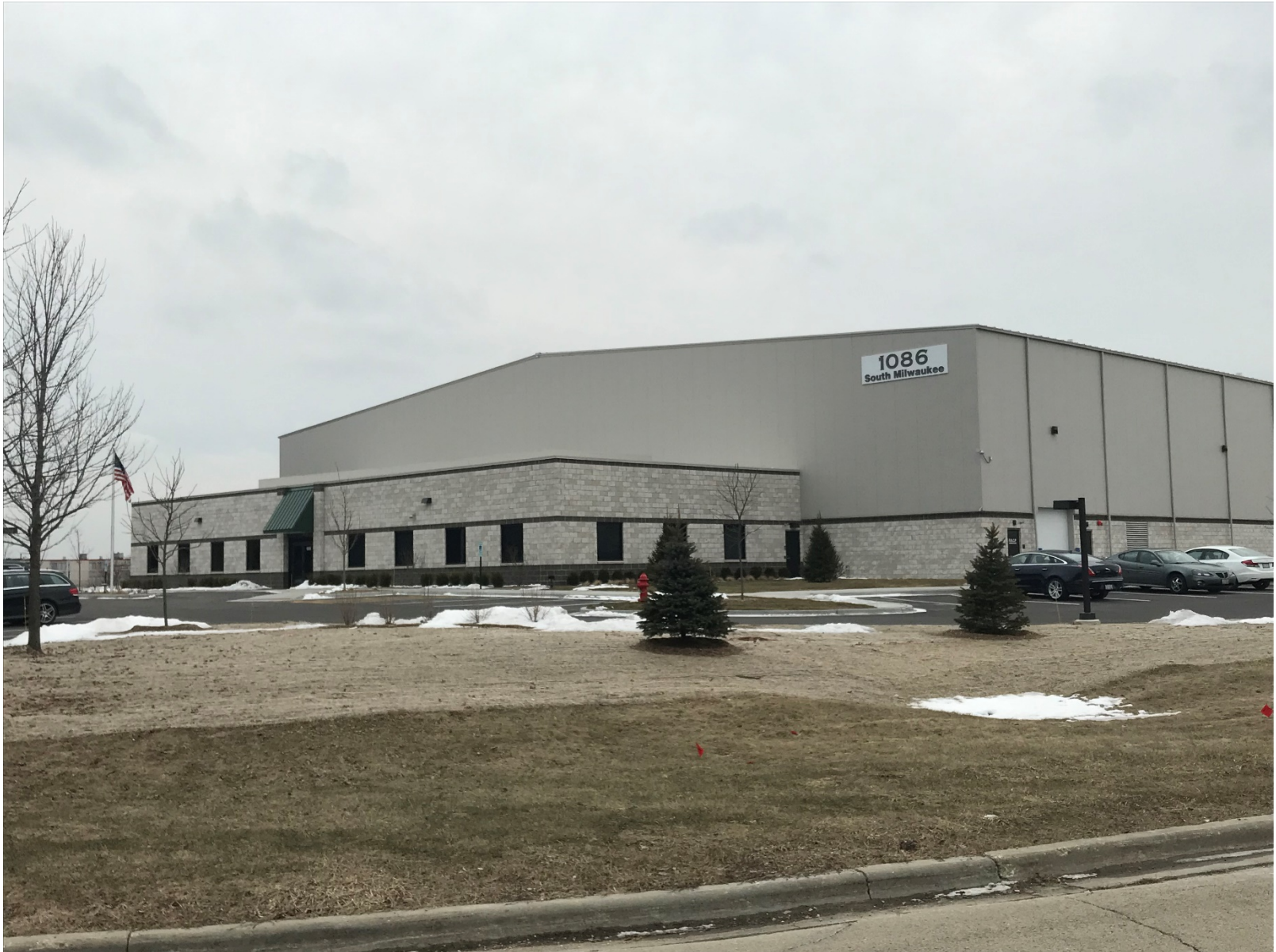
Existing conditions of subject unit (looking west)
