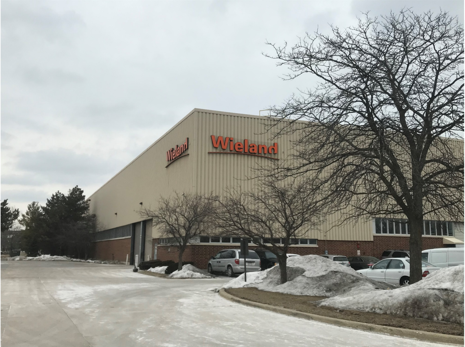
Existing Wall Signs (looking northeast)
