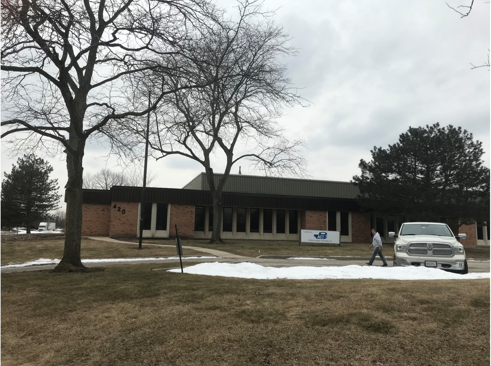
Existing conditions (looking west)
