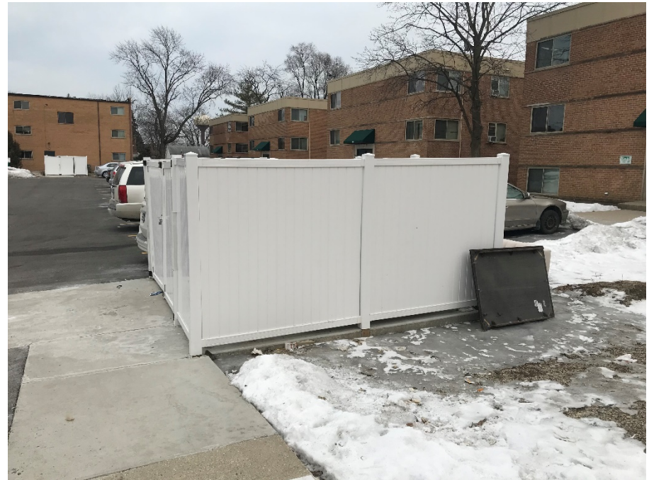
White Vinyl Enclosure (looking east)
