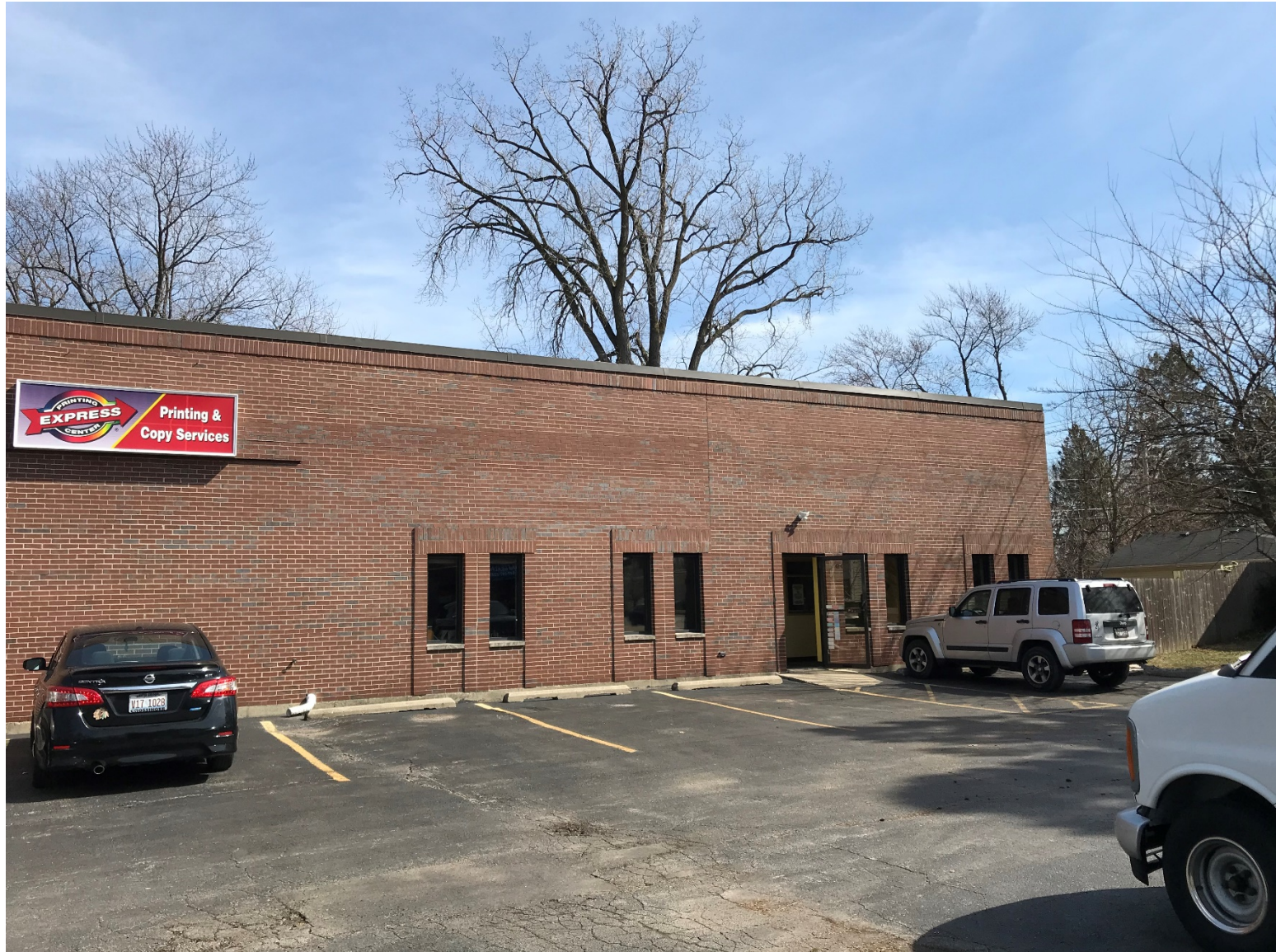
Existing conditions of site (looking east)
