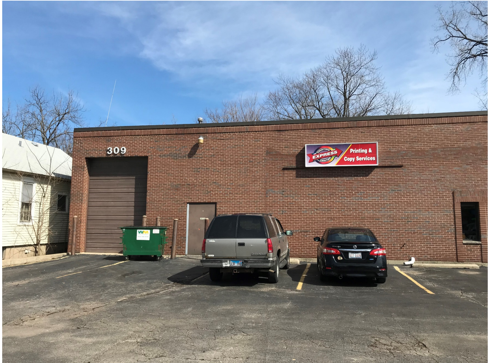
Existing conditions of site (looking east)
