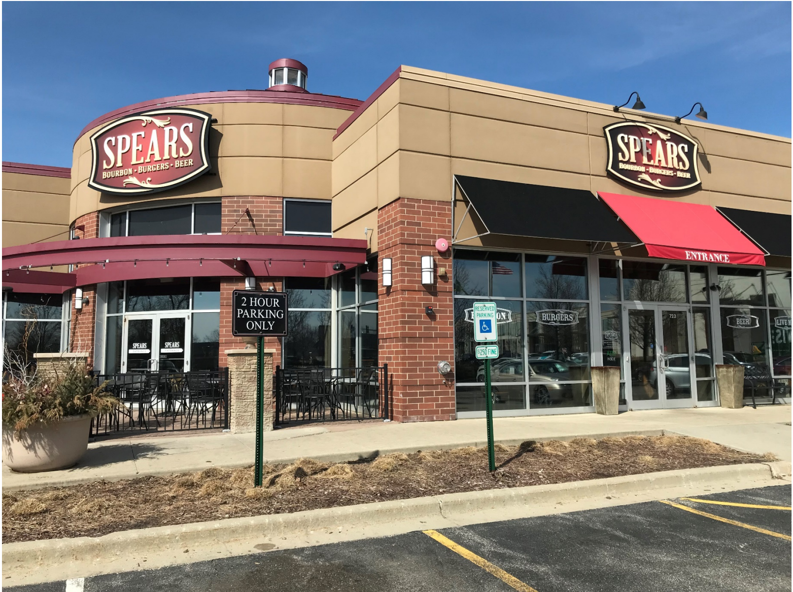
Existing conditions of subject unit (looking north)
