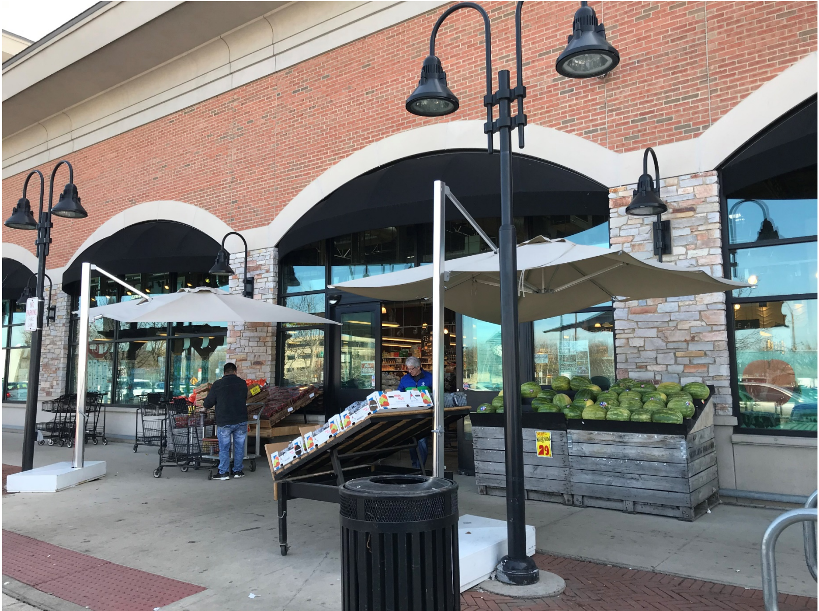
Existing conditions of front entry (looking south)
