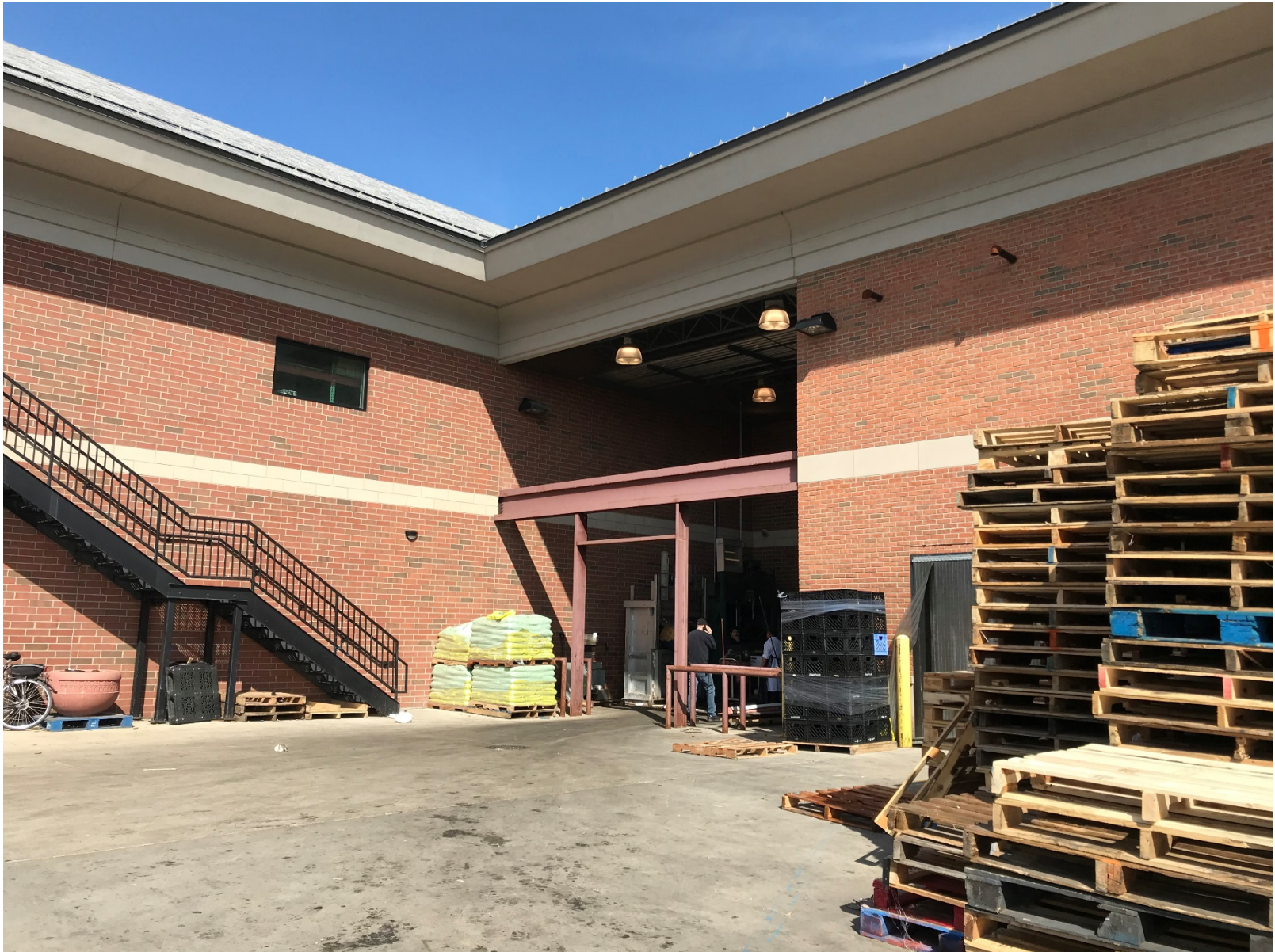
Existing conditions of rear loading area (looking northeast)
