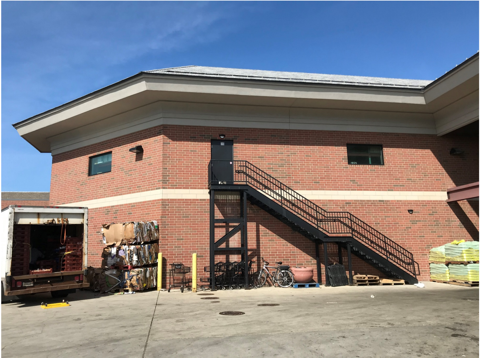
Existing conditions of rear loading area (looking north)
