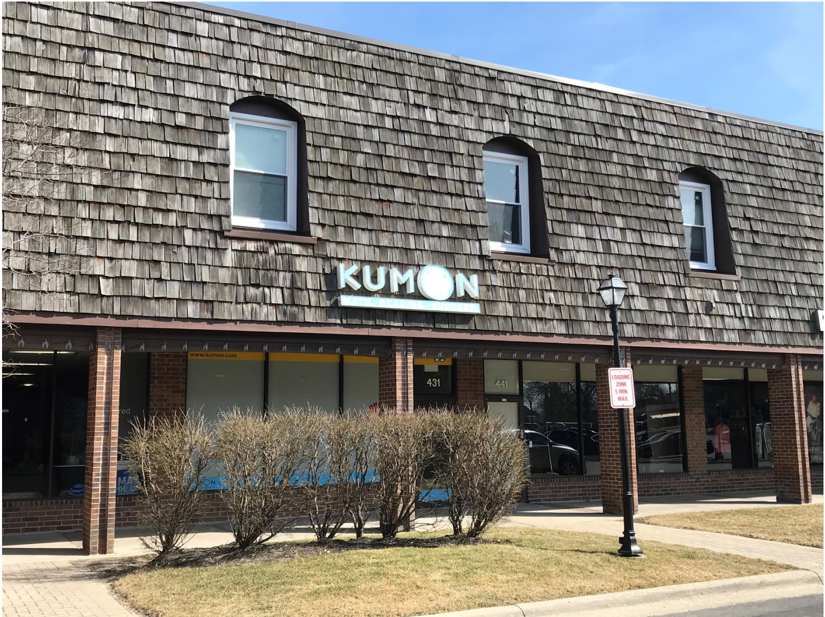
Existing conditions of subject unit (looking east)
