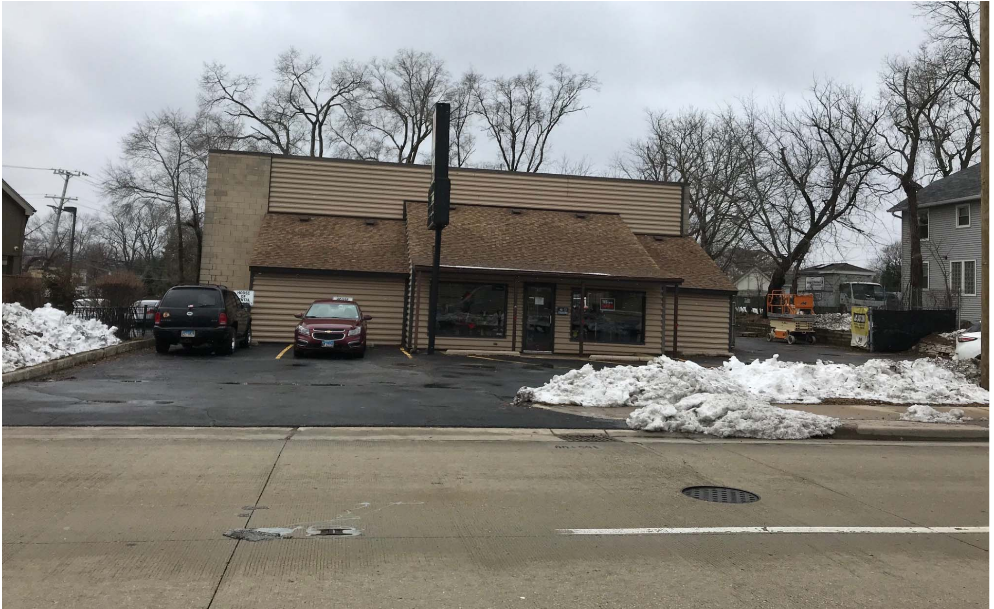
Existing conditions of subject property – east elevation
