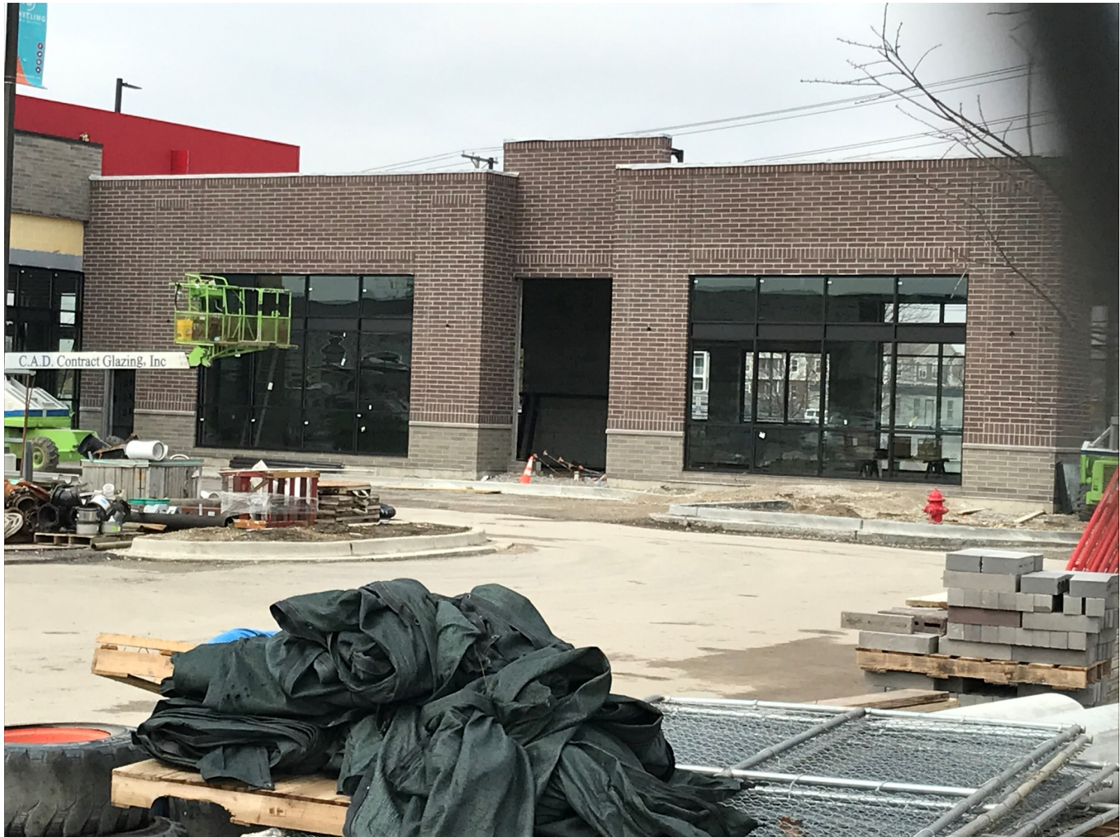
Existing conditions of subject building (looking north)
