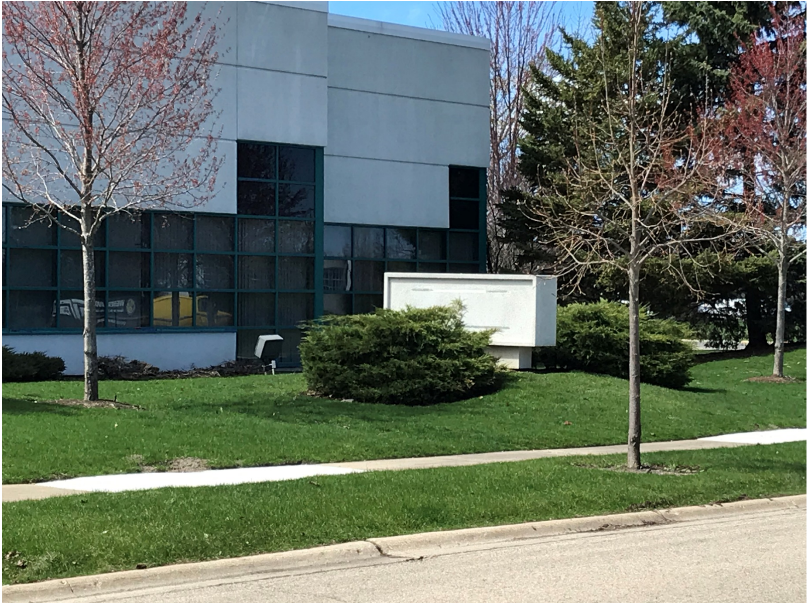
Existing conditions (looking north)
