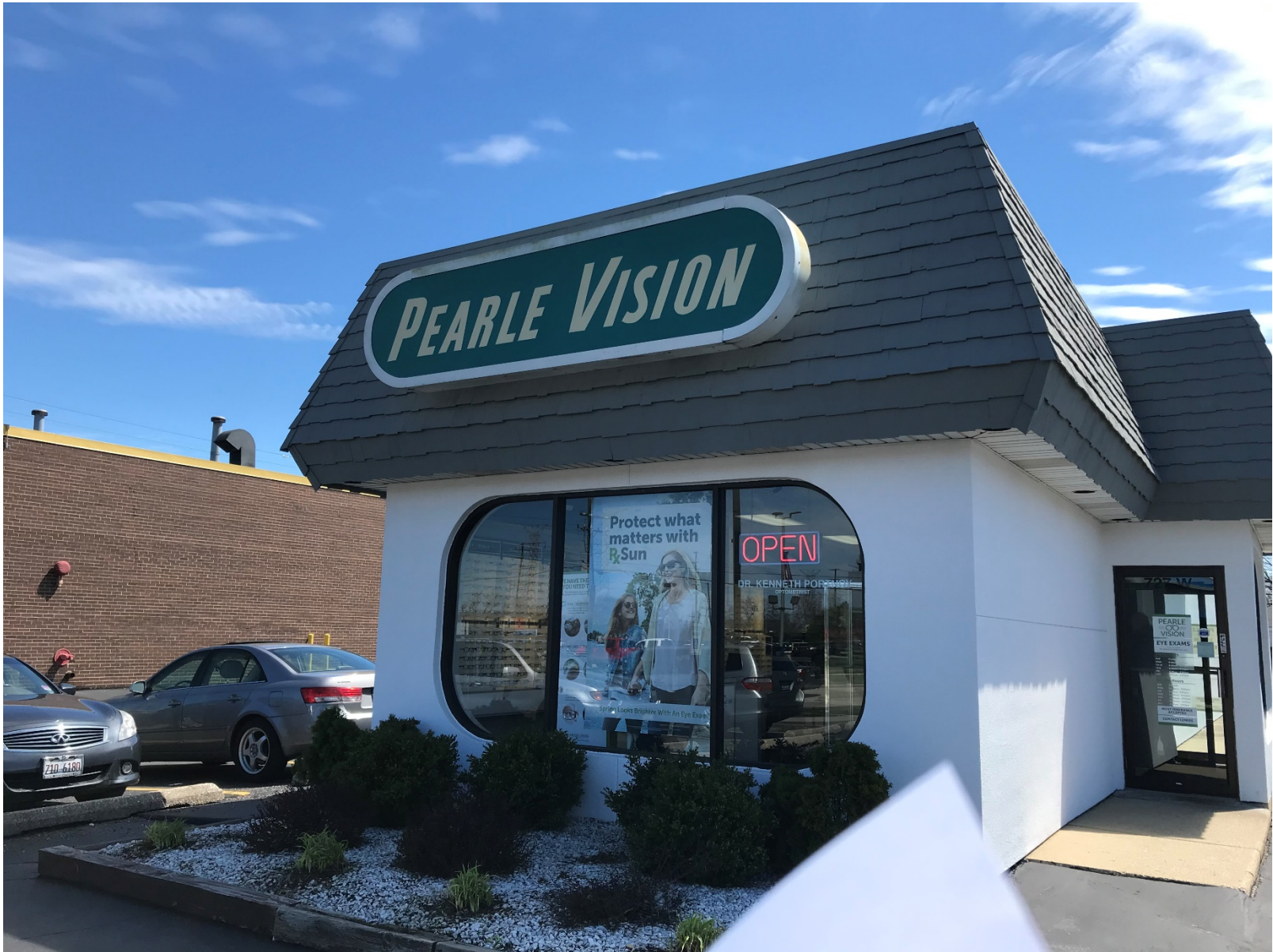
Existing conditions of wall sign (looking south)
