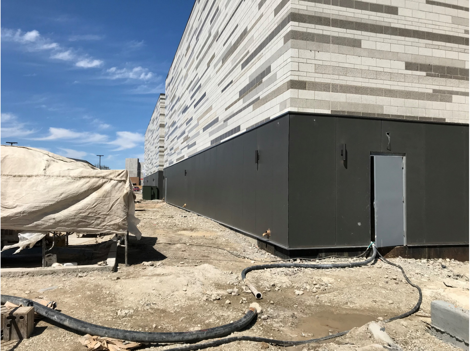
Existing conditions of site – Rear of CMX Building (looking north)
