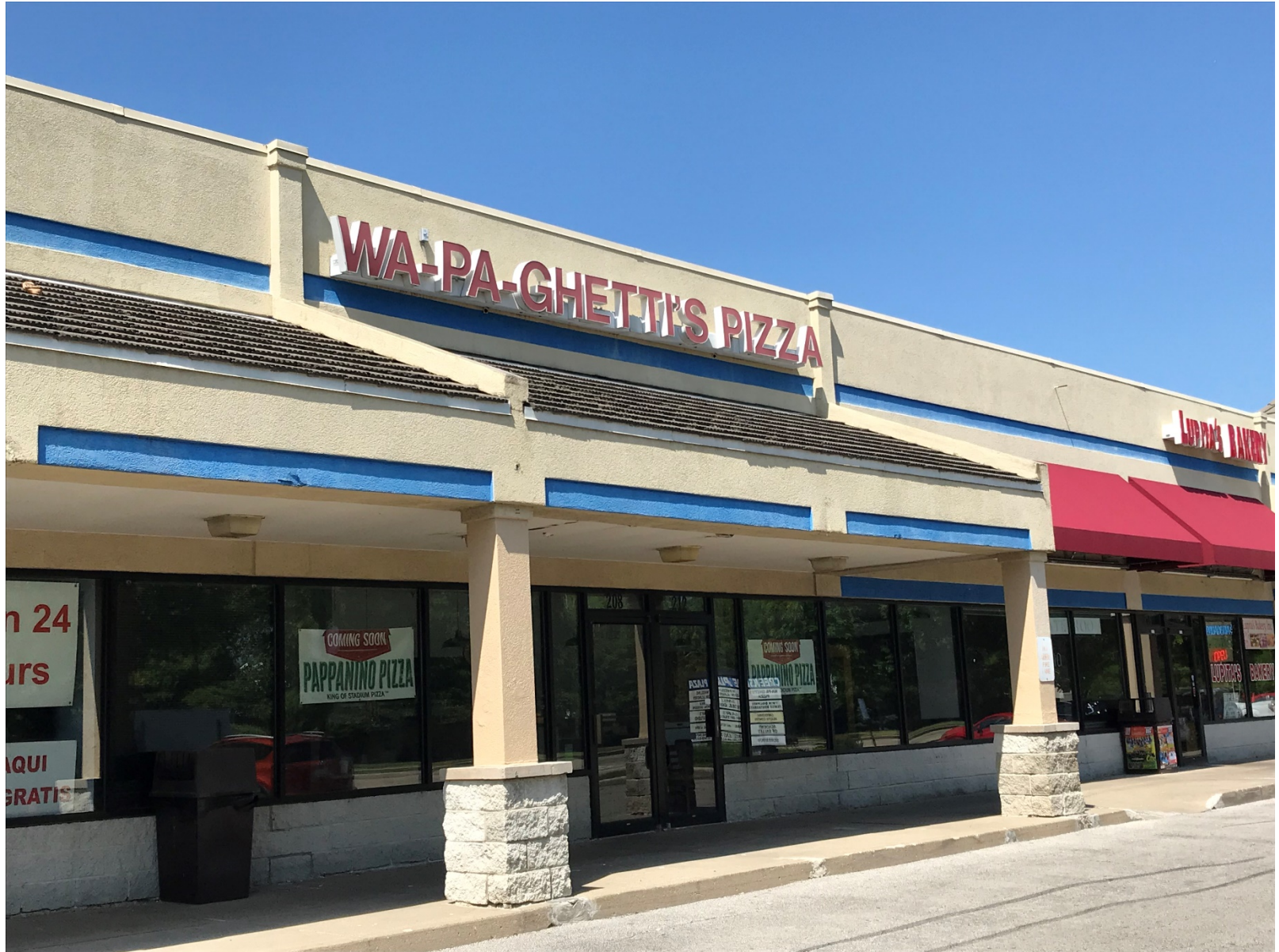
Existing conditions of subject unit (looking northwest)
