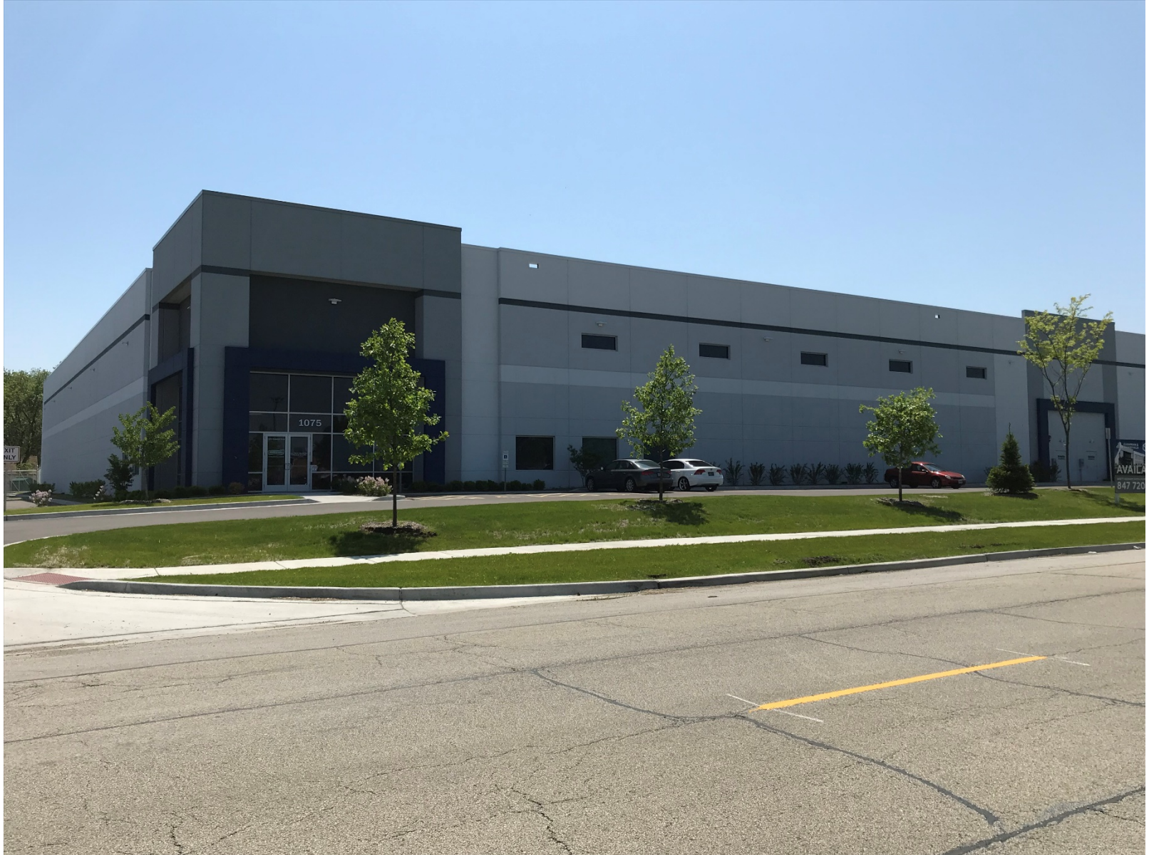
Existing conditions of subject unit (looking east)
