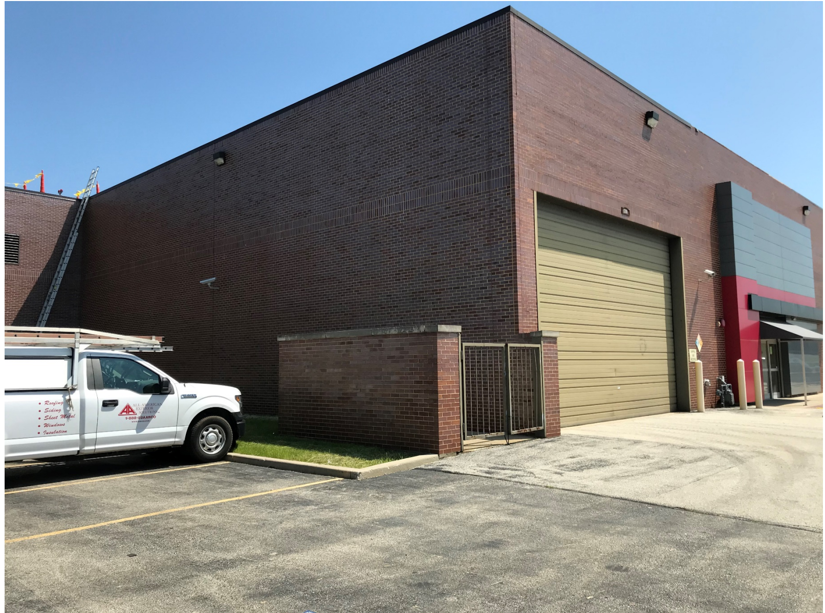
Existing conditions of subject property (looking northeast)
