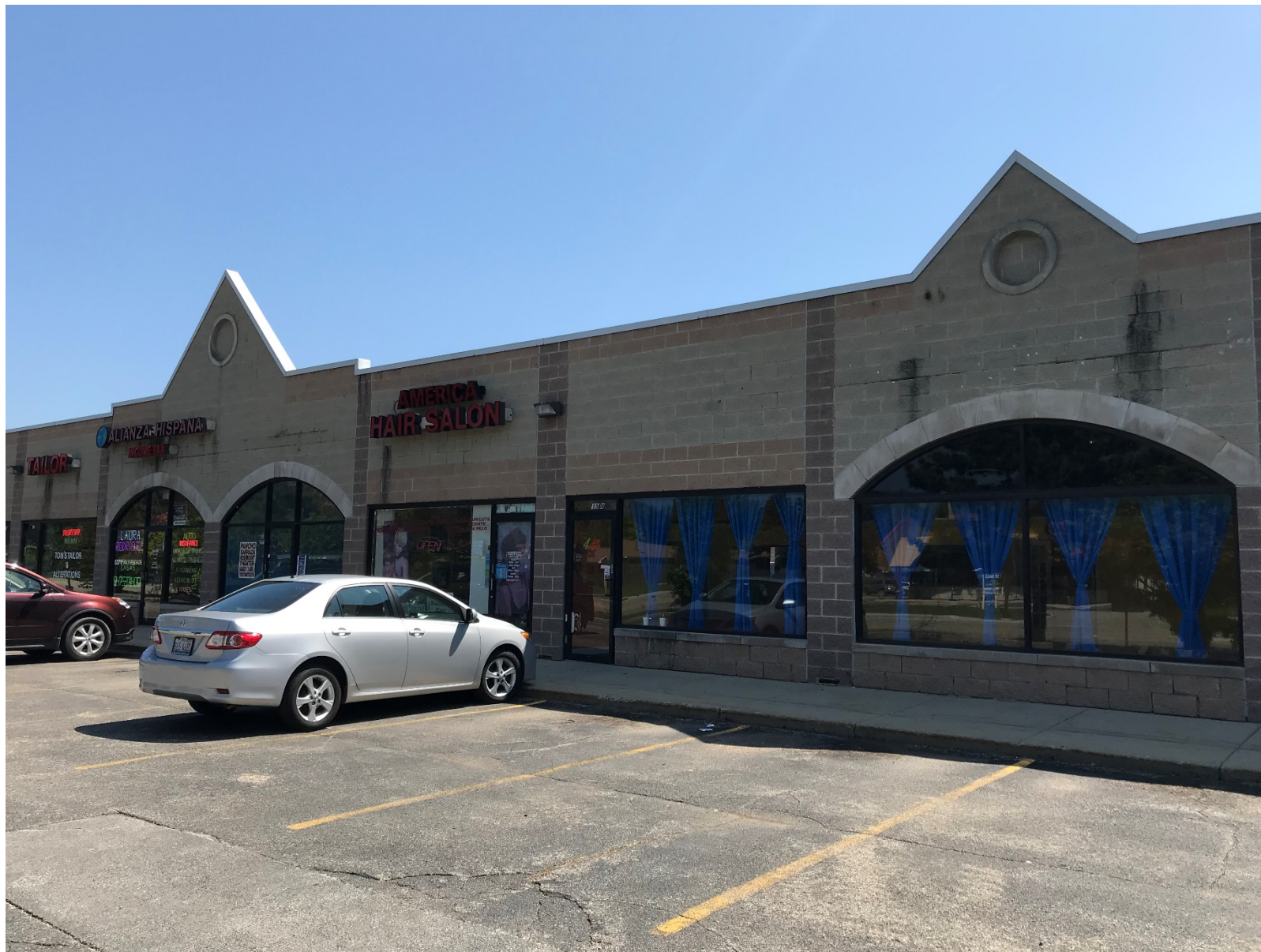
Existing conditions of subject unit (looking east)
