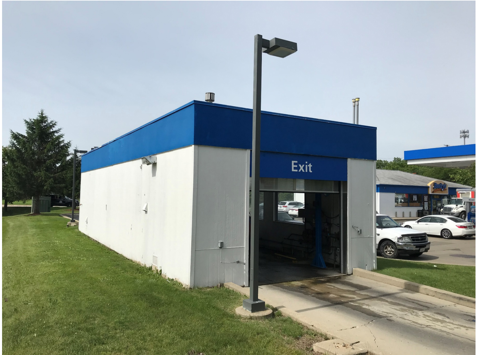
Existing conditions of car wash (looking southwest)
