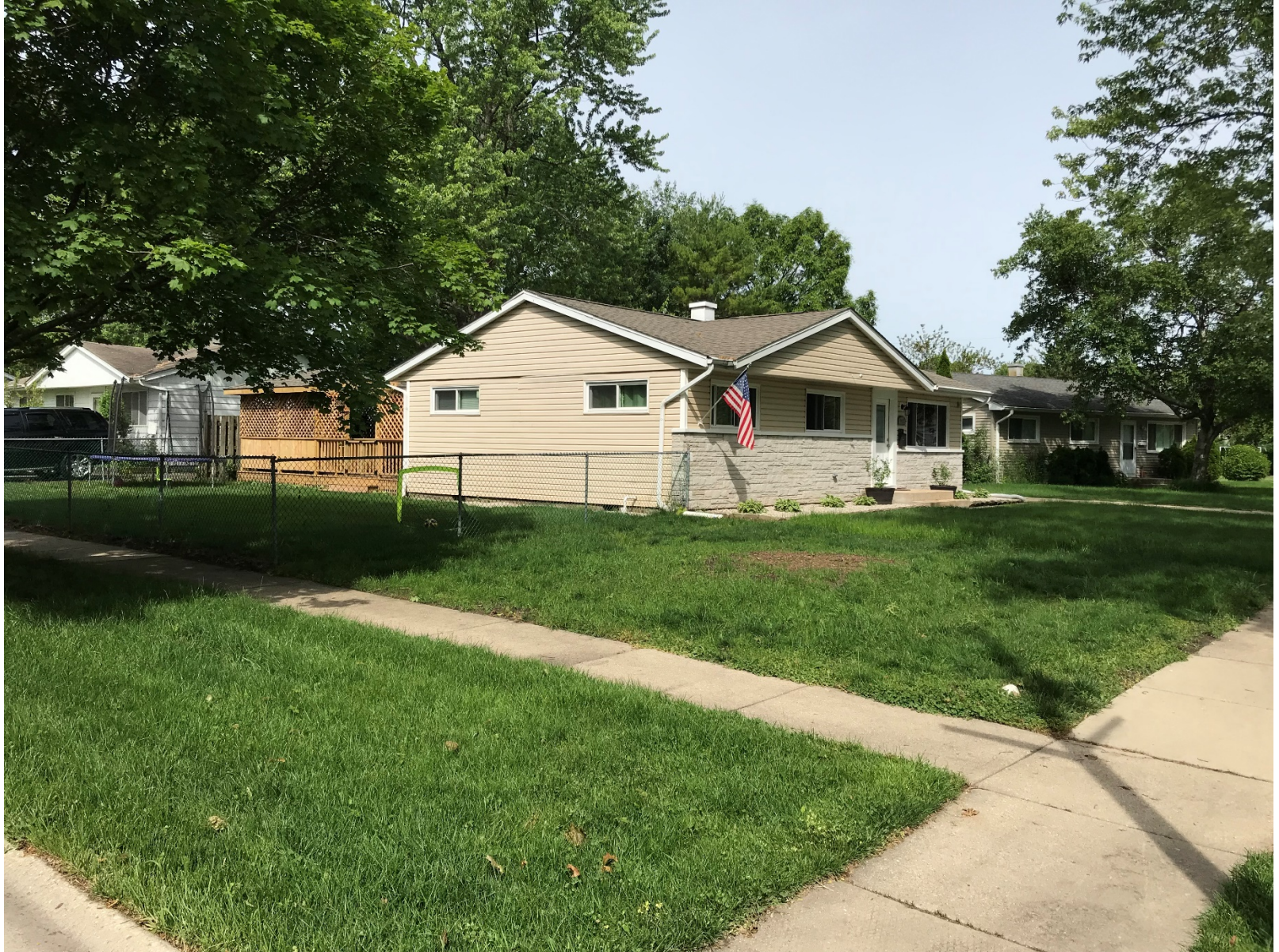
Existing conditions of subject property (looking southwest)
