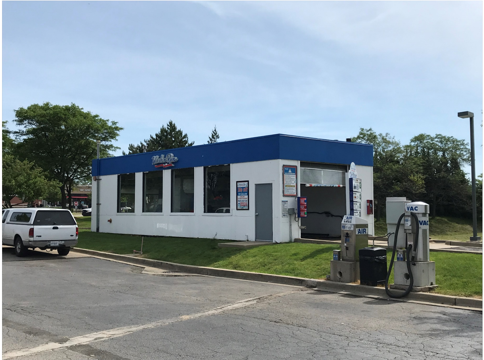
Existing conditions of car wash (looking east)
