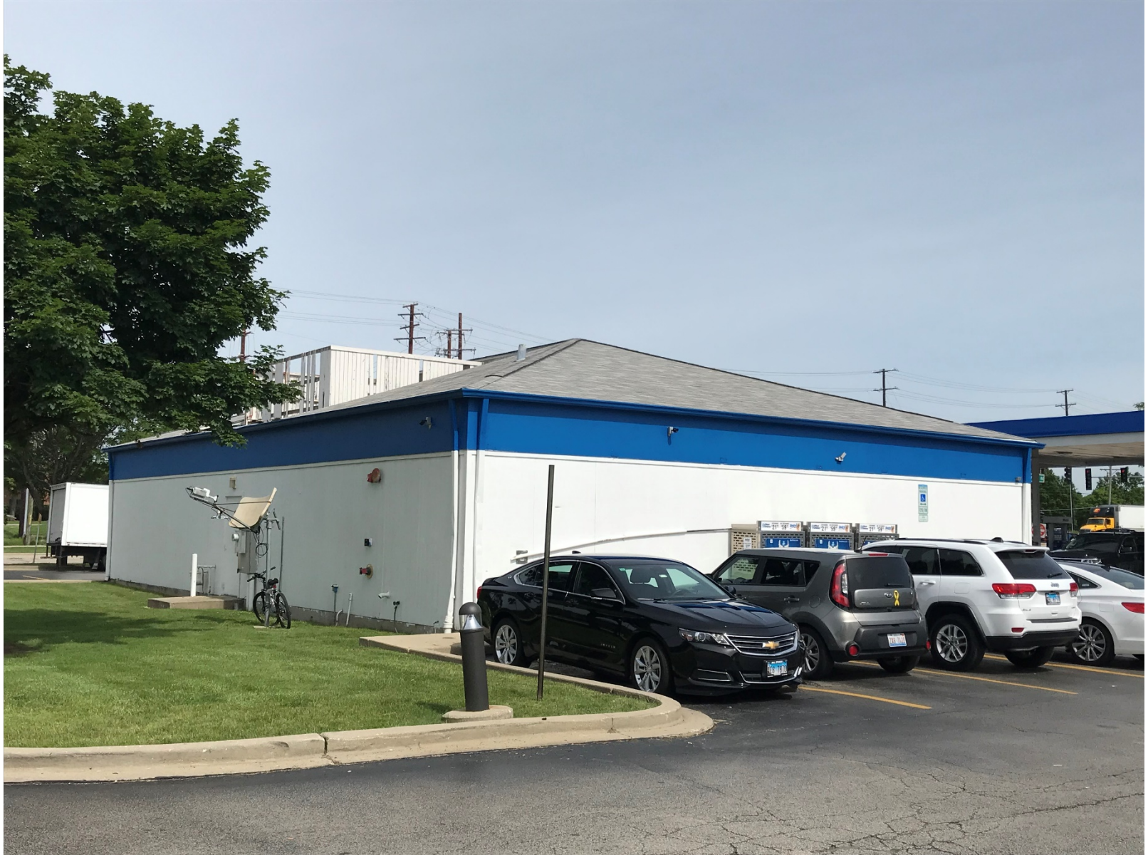
Existing conditions of mini mart (looking west)
