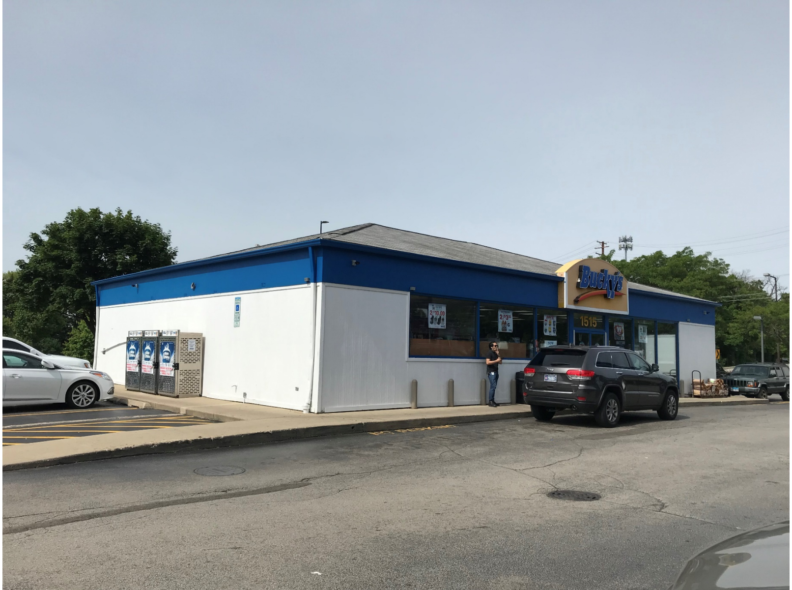
Existing conditions of mini mart (looking southwest)
