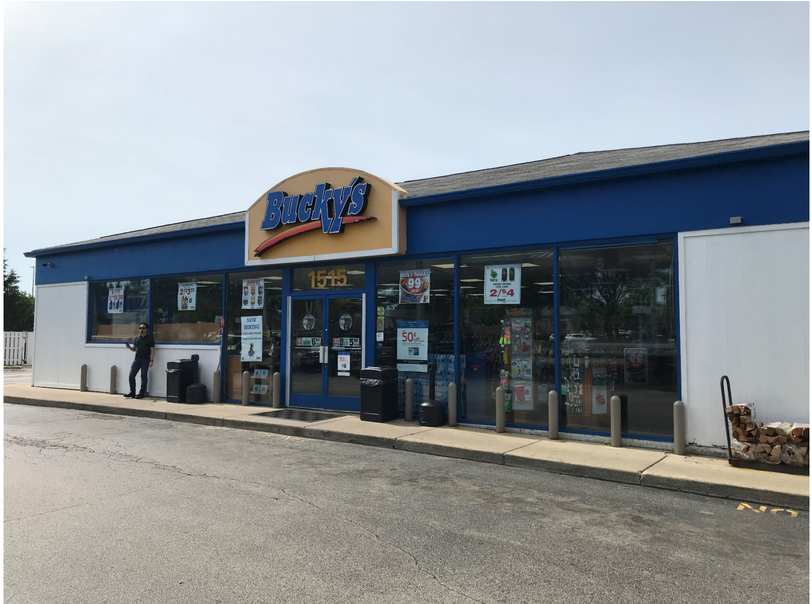
Existing conditions of mini mart (looking south)
