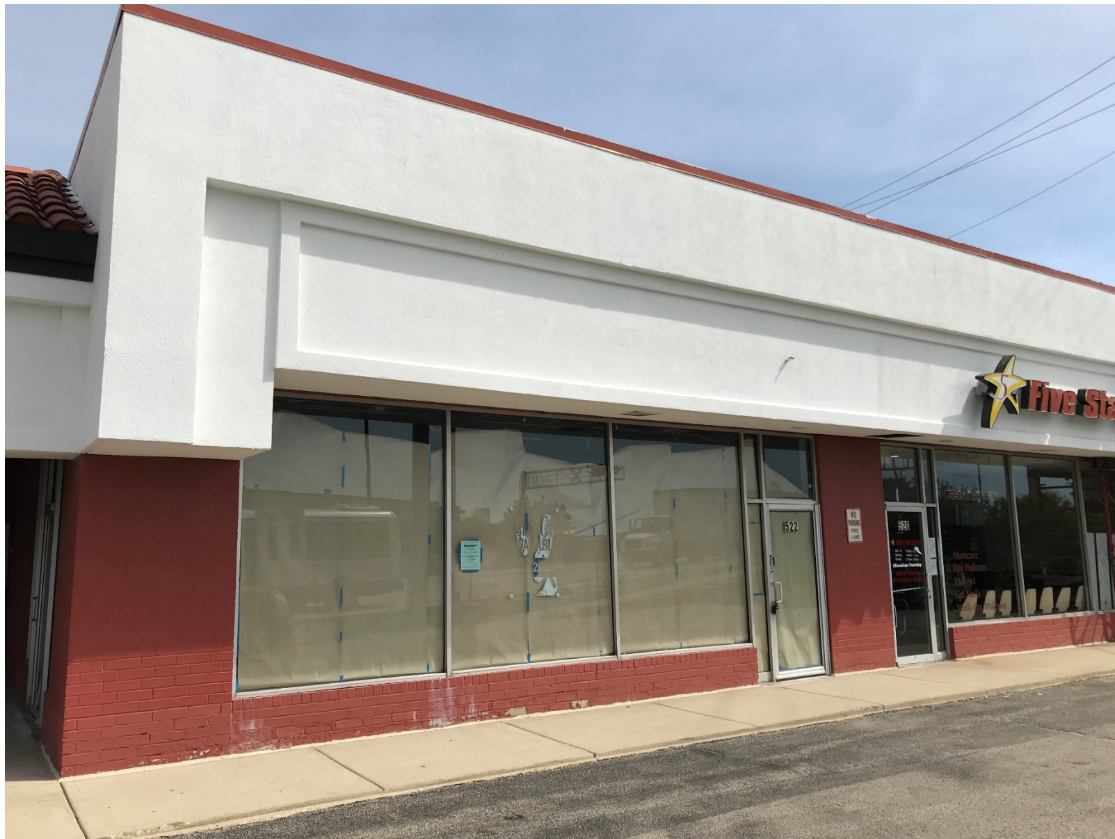
Existing conditions of subject unit (looking north)
