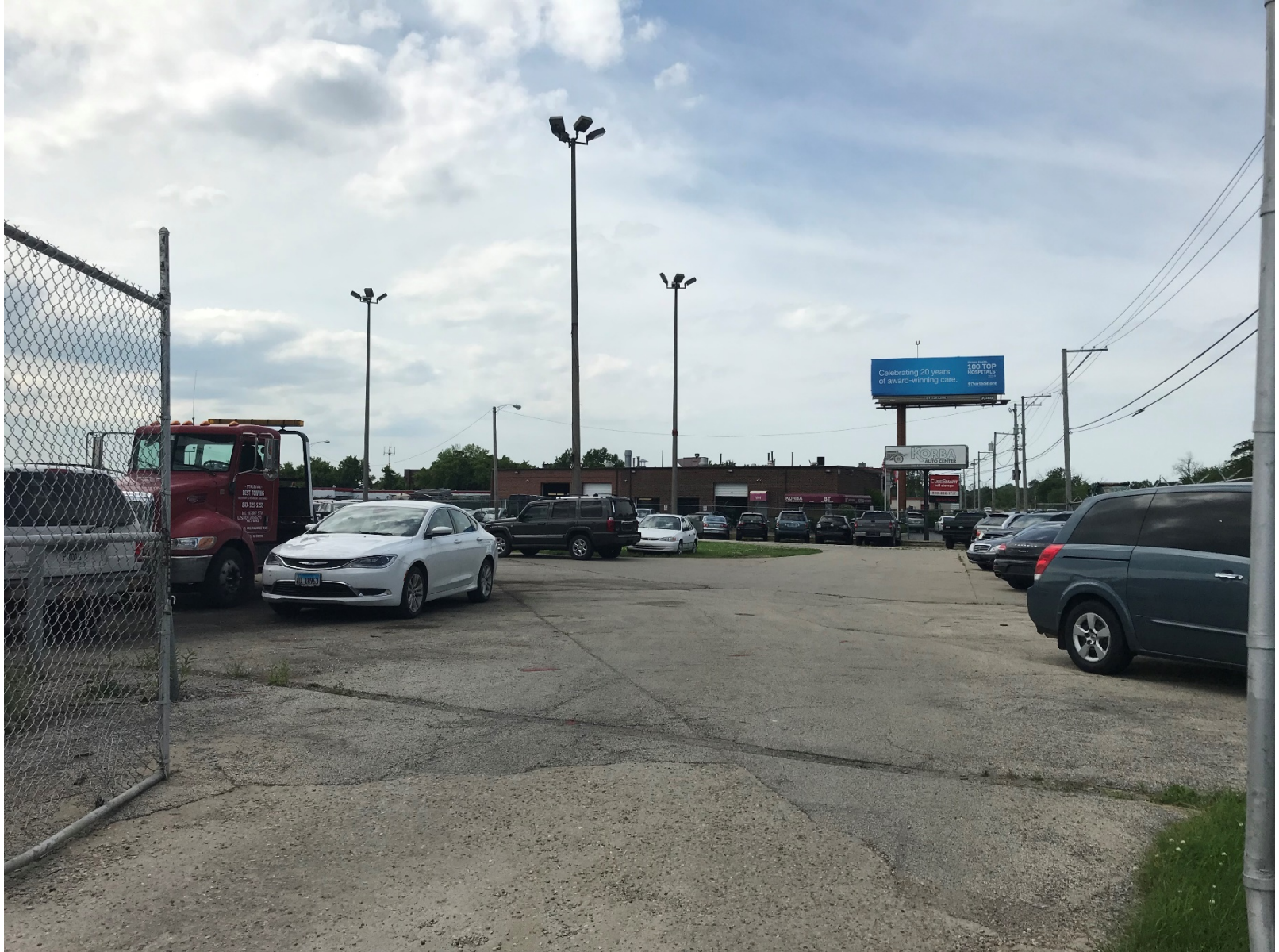
Existing conditions of subject property (looking north)
