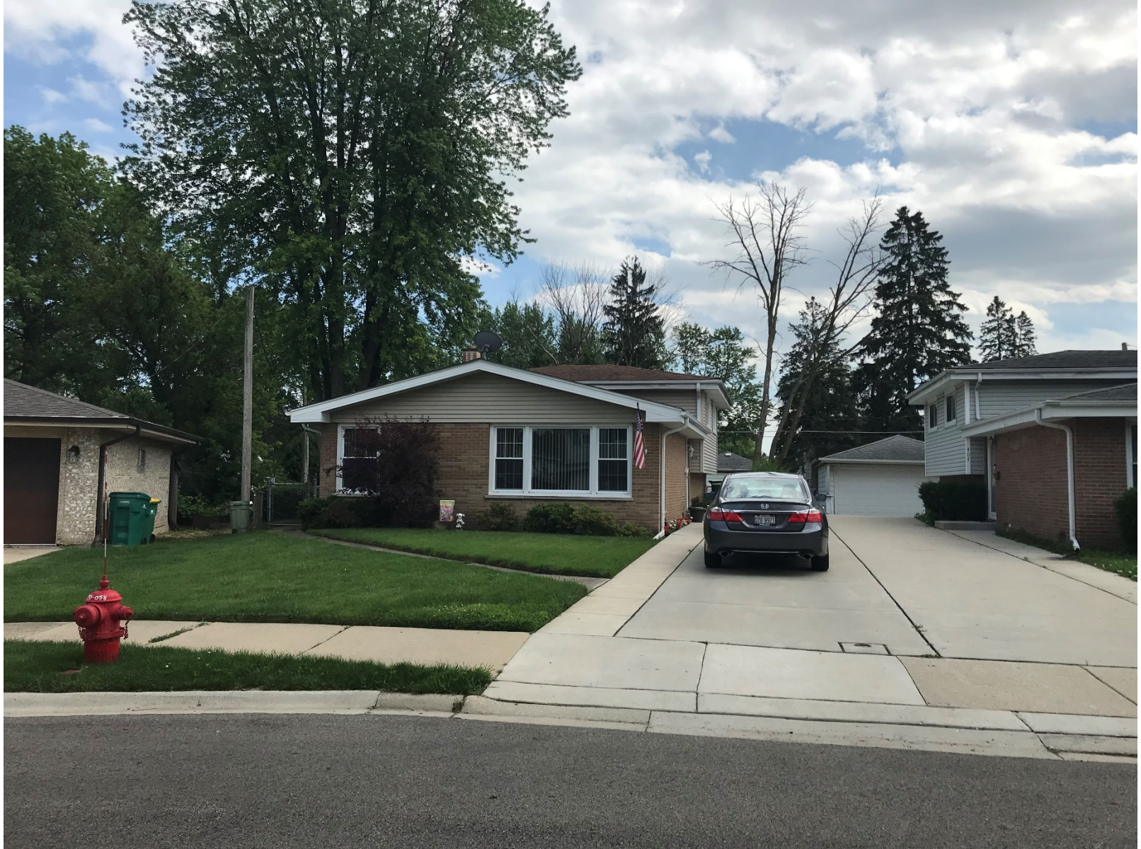
Existing conditions of subject property (looking south)
