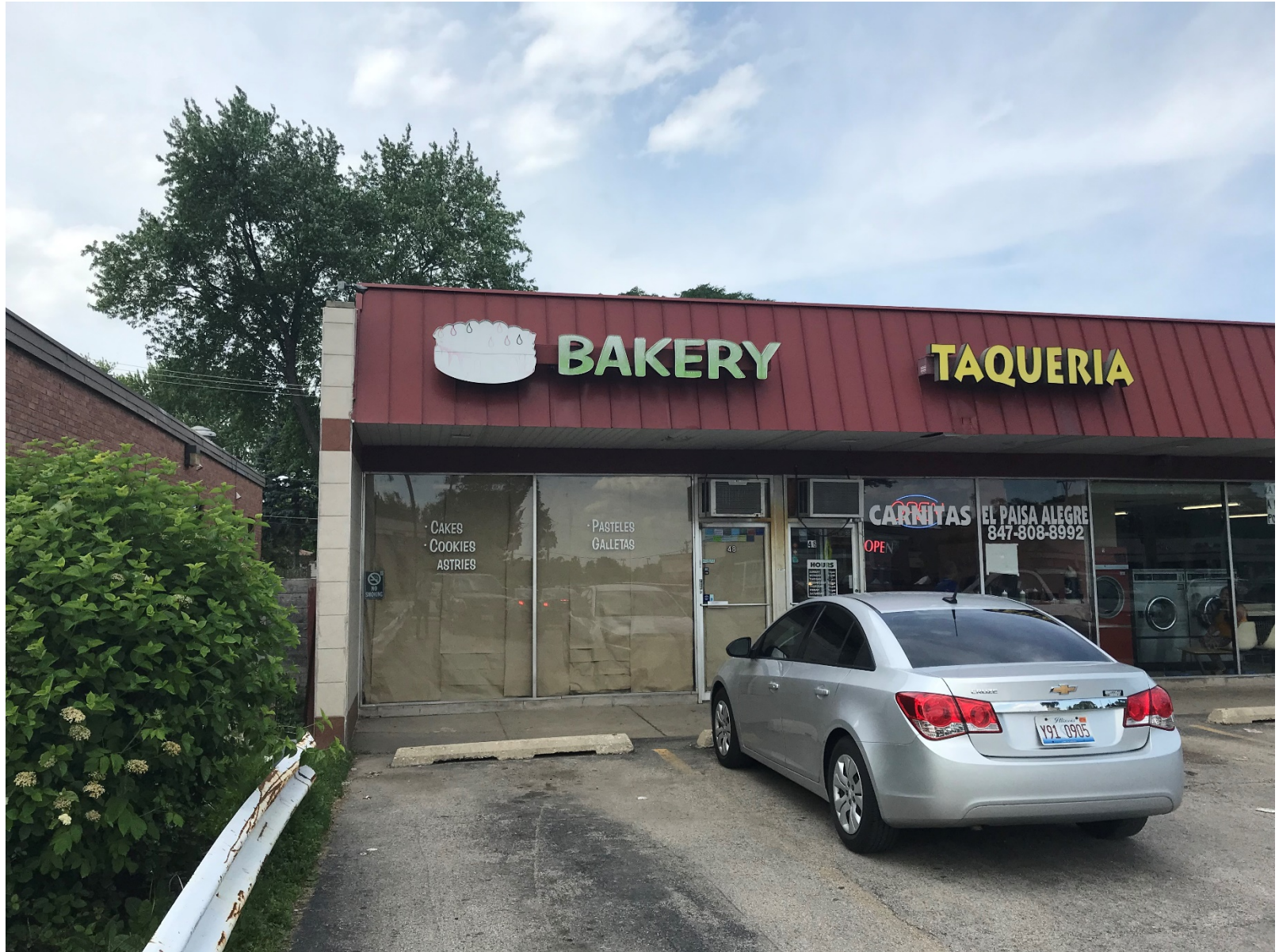
Existing conditions of subject unit (looking south)
