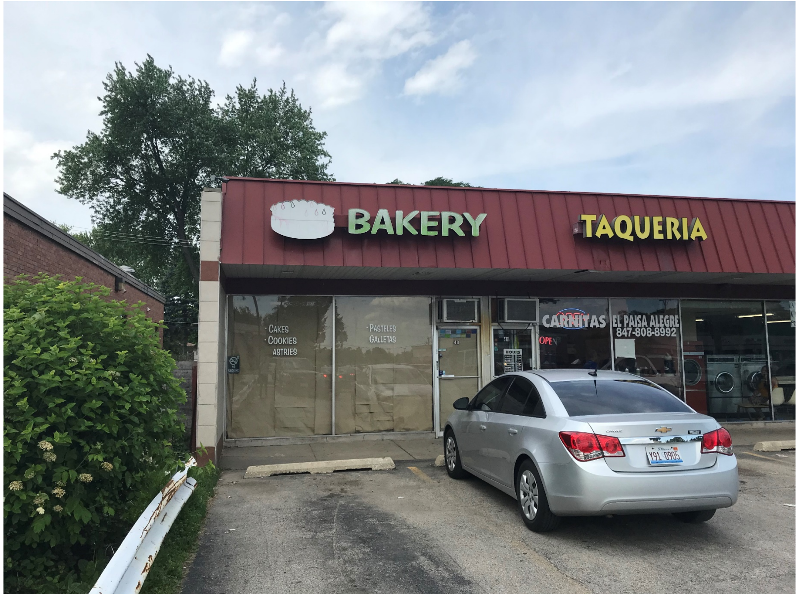
Existing conditions of subject unit (looking south)
