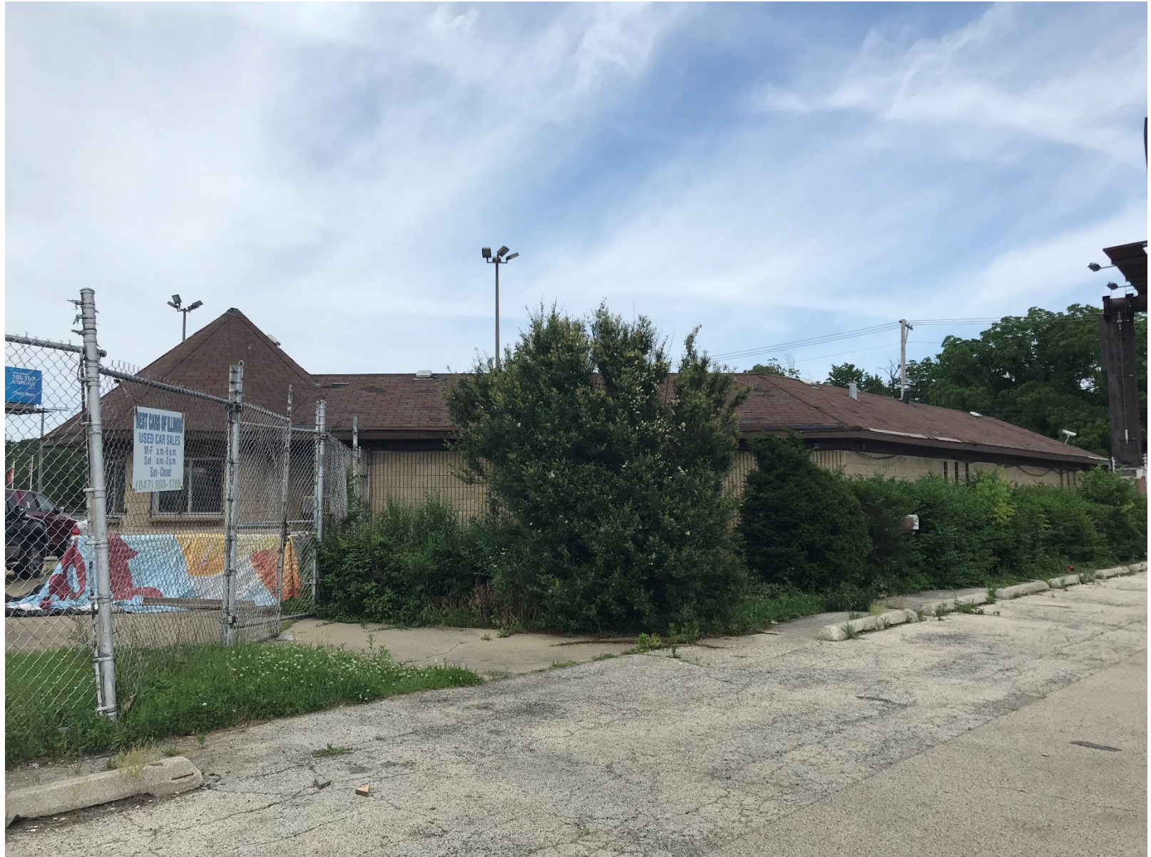
Existing conditions of subject property (looking northeast)
