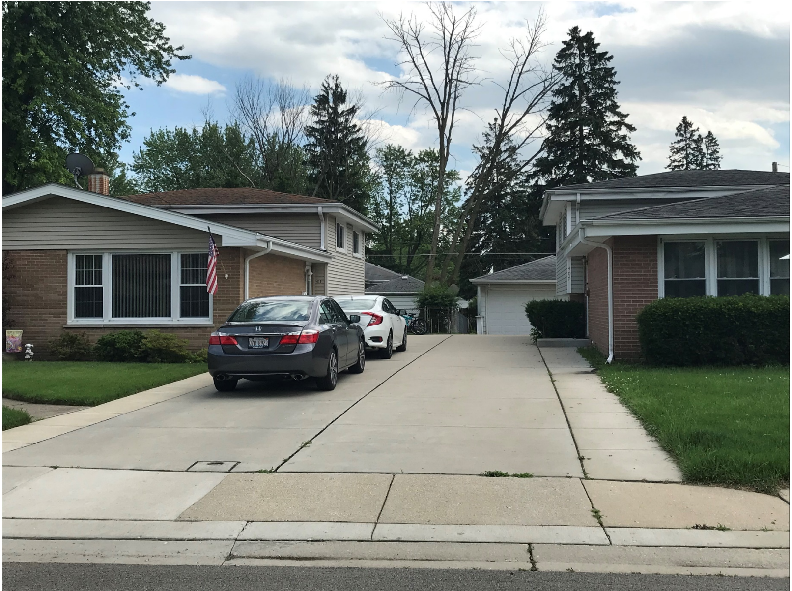
Existing conditions of subject property (looking south)
