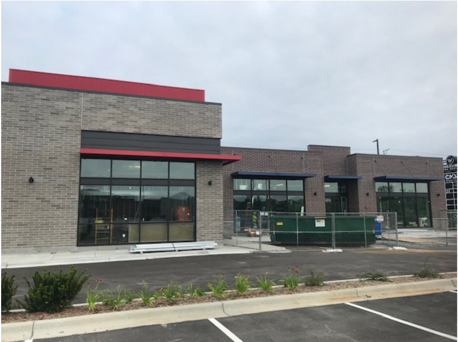
Existing conditions of subject unit (looking northeast at south elevation)
