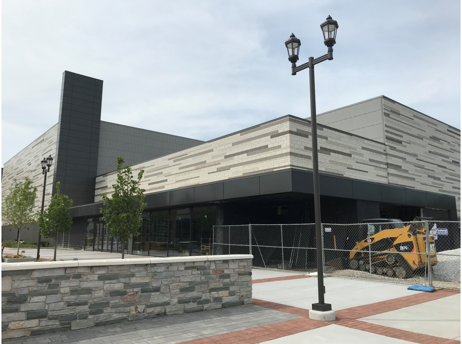
Existing conditions of subject building (looking southwest)
