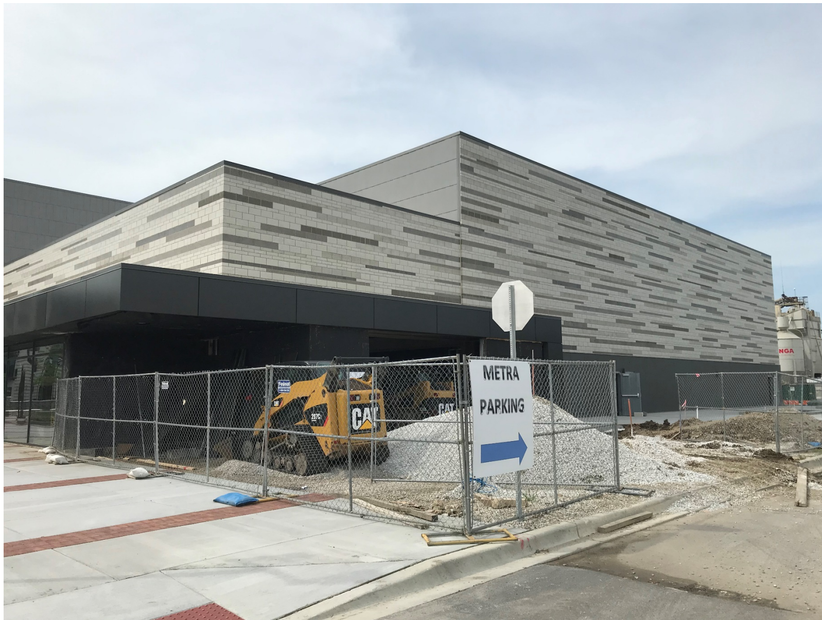
Existing conditions of subject building (looking southwest)
