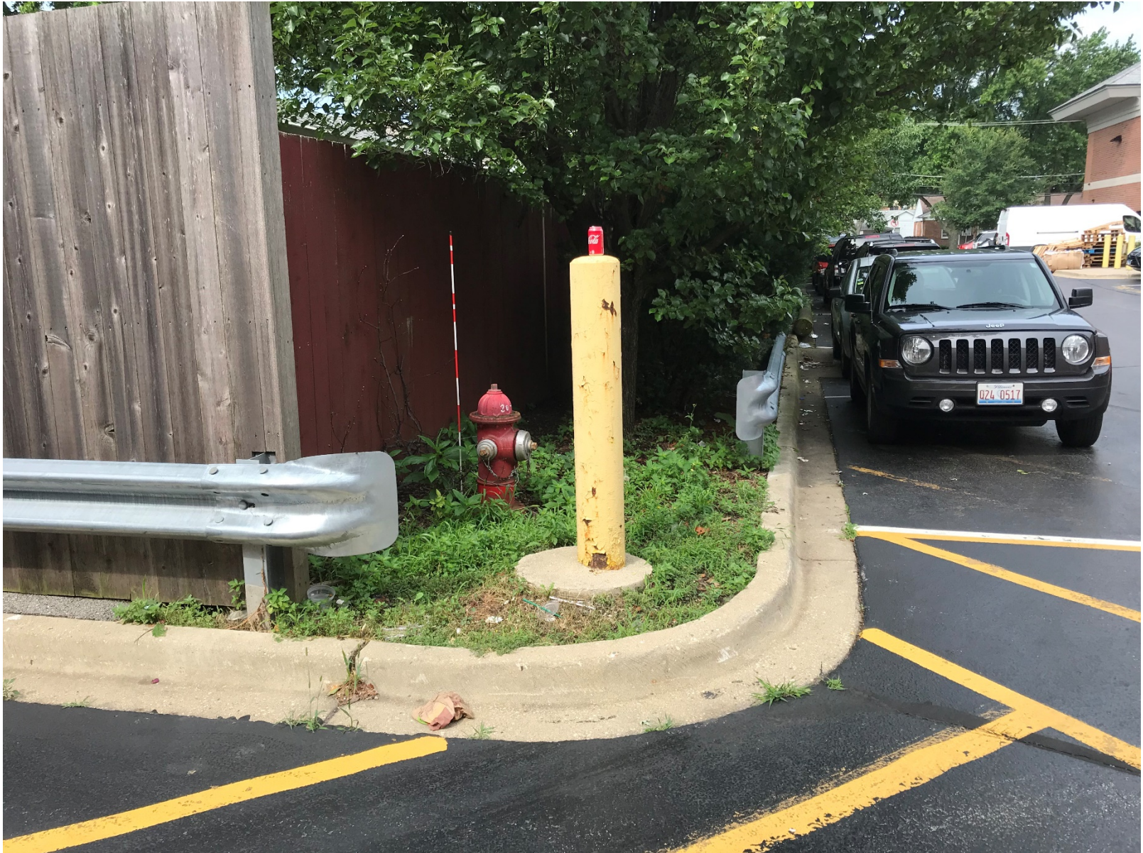
Existing conditions of rear area – fire hydrant and curbing (looking west)
