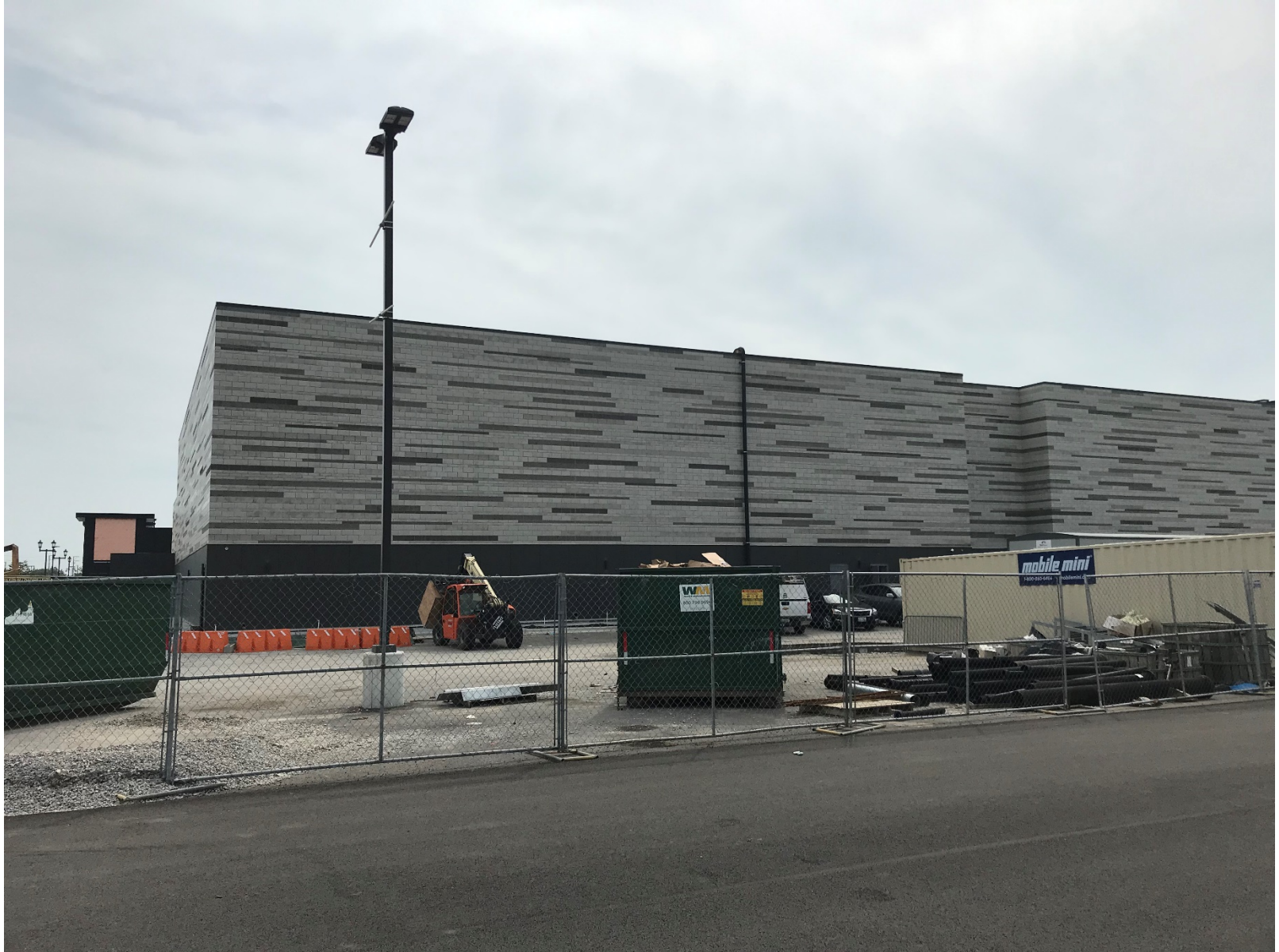
Existing conditions of subject building (looking east)
