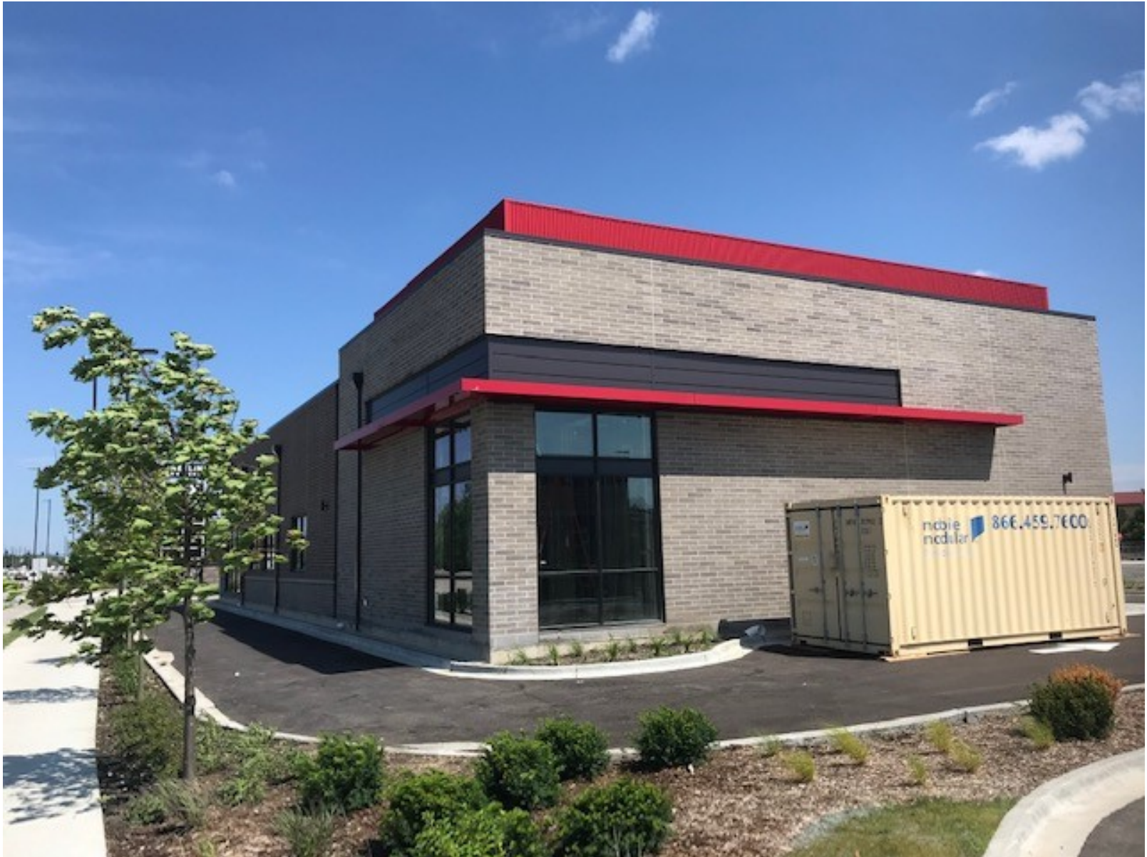
Existing conditions of subject unit (looking southeast at north and west elevations)
