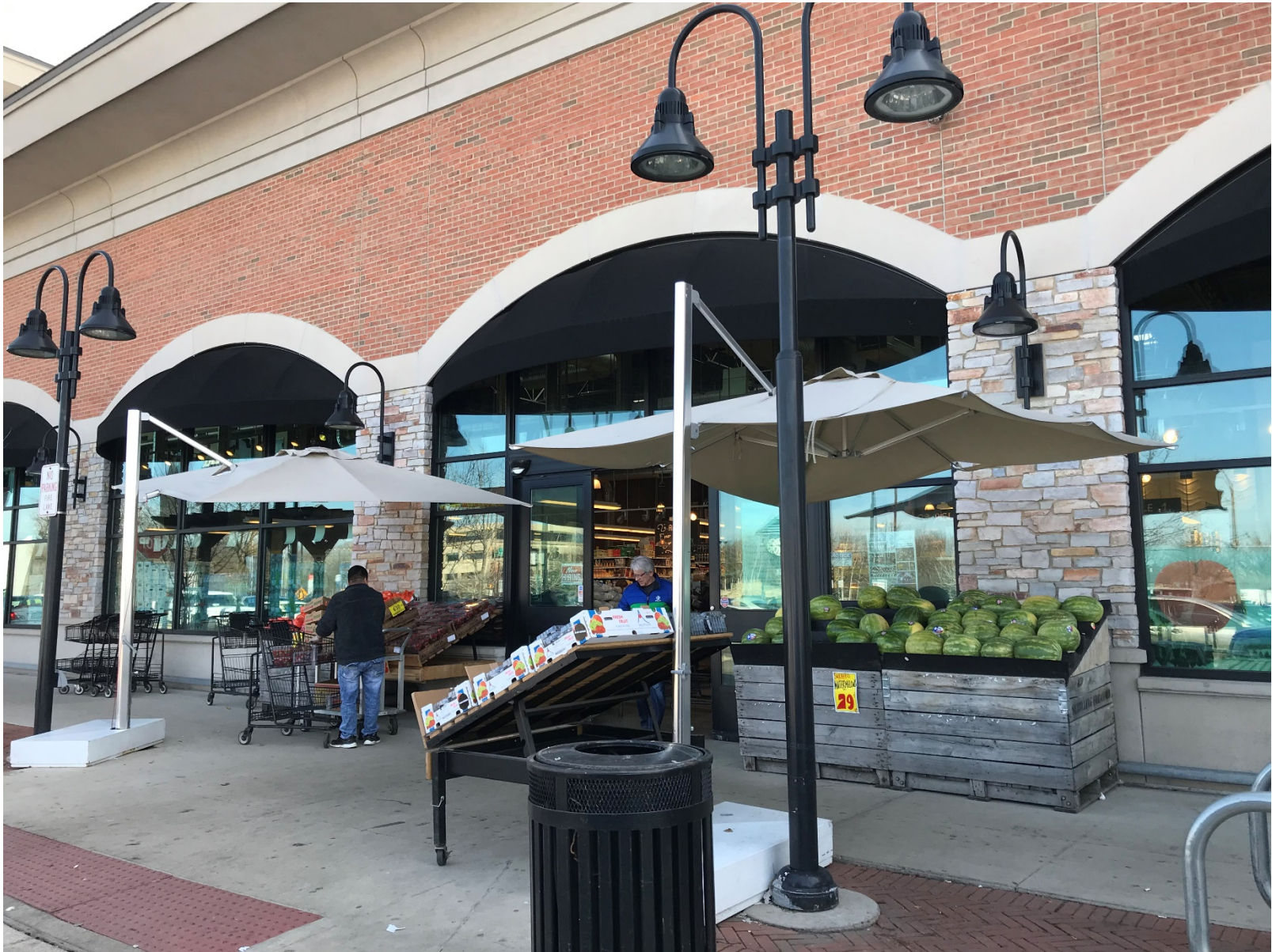
Existing conditions of front entry (looking south)
